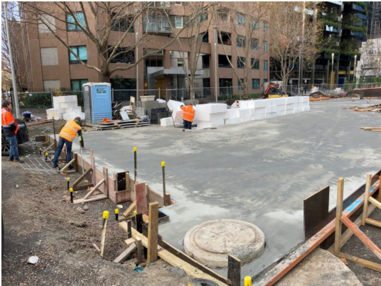
Southbank Boulevard play space concrete slab
