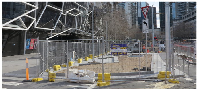
Progress on Stage 2 of Southbank Boulevard.
