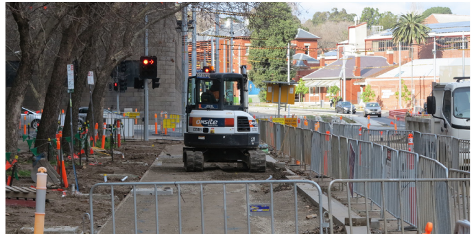
Cycle lane construction underway between Sturt Street and Moore Street.
