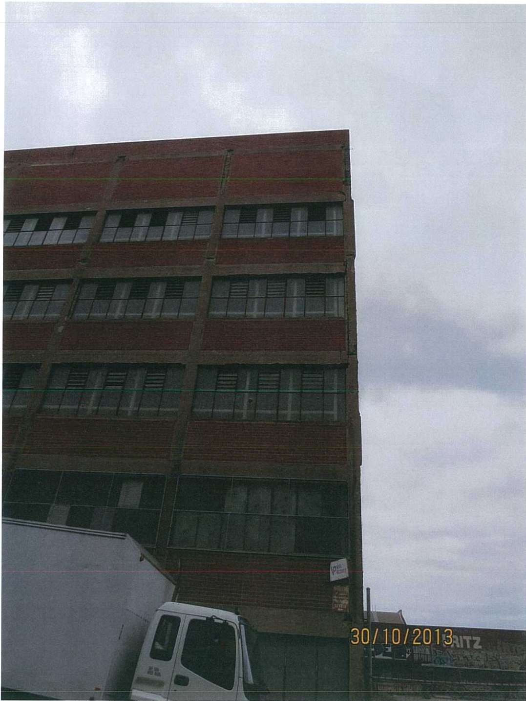
Catch fan required over adjacent building to collect spalls.
