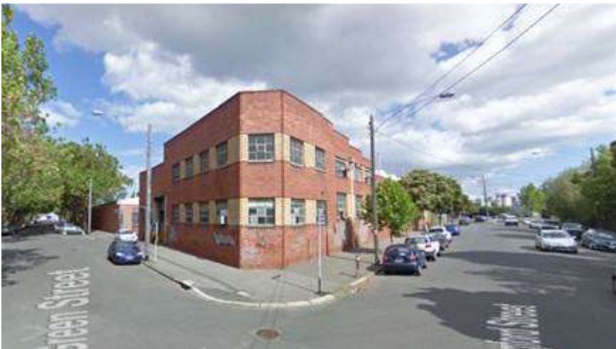
Figure 3: MCC Depot office (Google street view)
