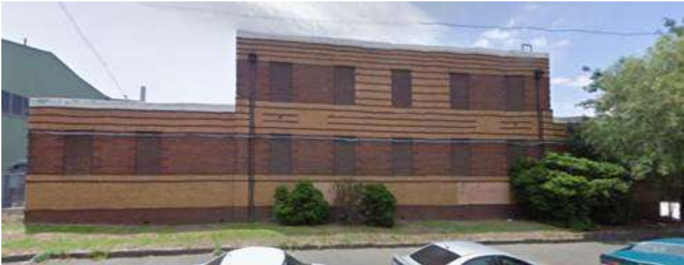
Figure 7: MCC substation (Google street view)
