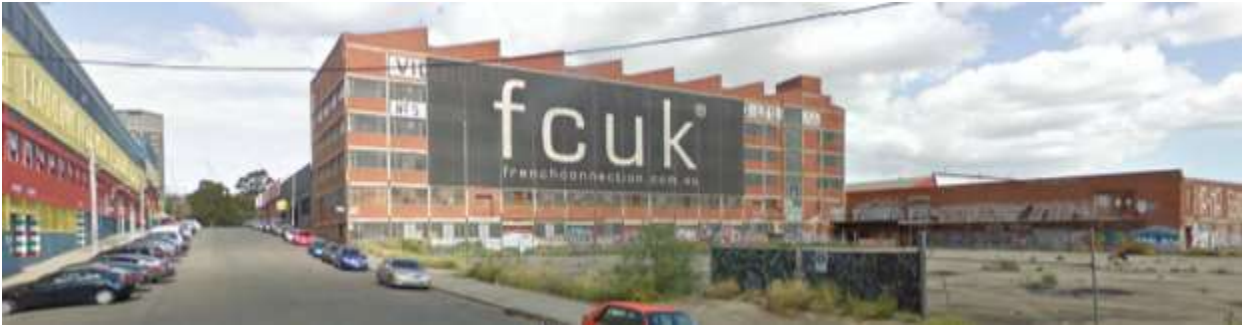
Figure 8: VPC No 5 Wool Store, and adjacent buildings
