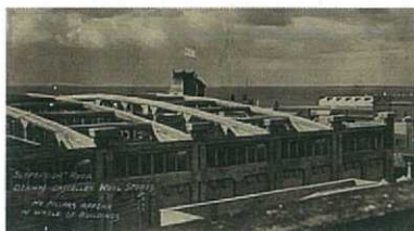
Bow String Truss Building
