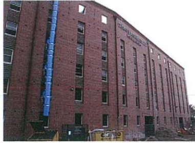
1934 wool store (prior to alterations)
