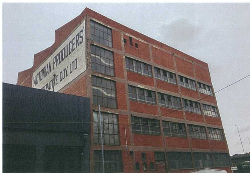
Figure 6 The north (Sutton Street) elevation of the building.
