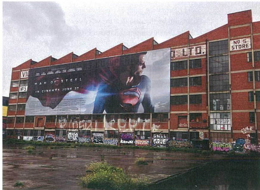
Figure 5 The west elevation of the subject building.
