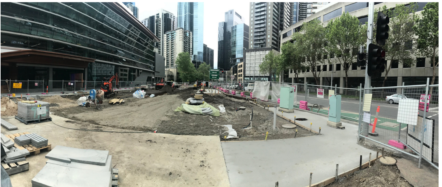
Civic Space works continue
