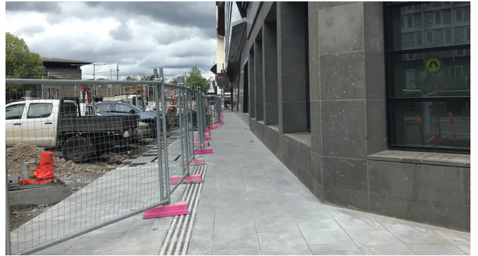
Footpath works in front of the ABC Centre
