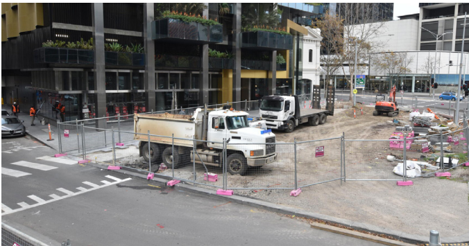
Neighbourhood park, Fawkner Street to City Road
