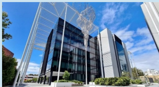
The Workzone East building at 1 Nash Street, Perth Source: Knight Frank
