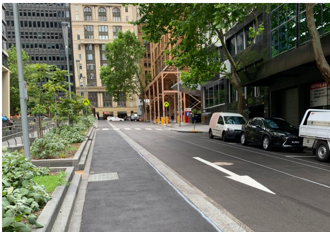
Completed roadway works and bike lane along Market Street
