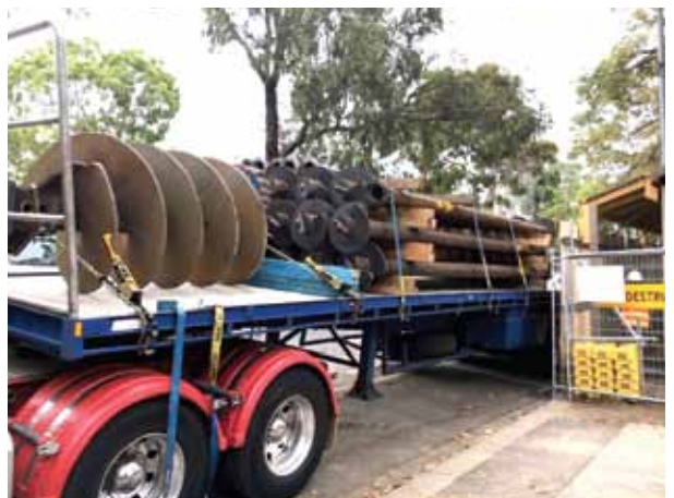
ABOVE: Delivering of the screw piles to site - March 2019
