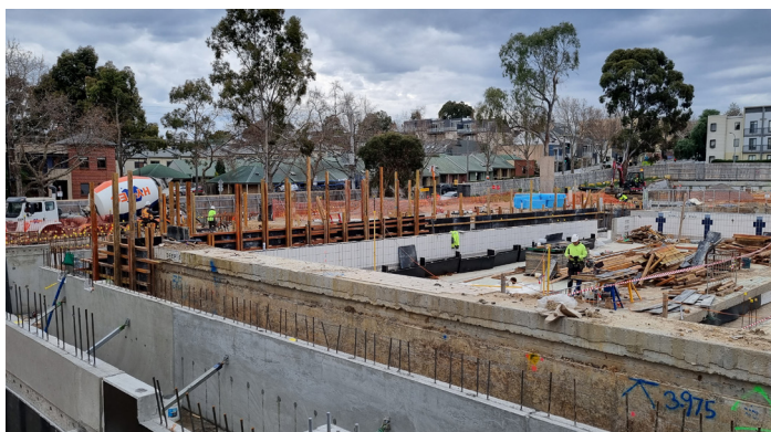
Works on the pool structure have started
