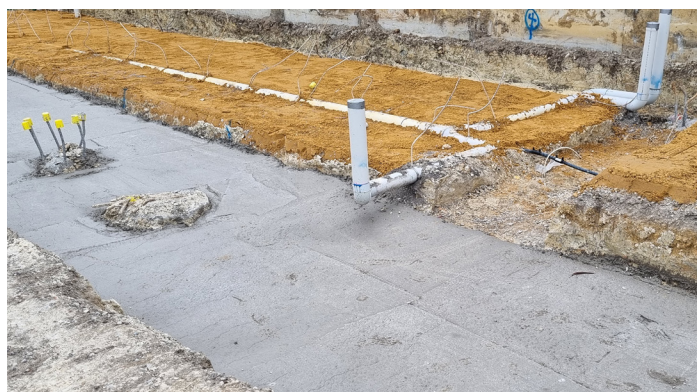
Concrete slabs are being poured
