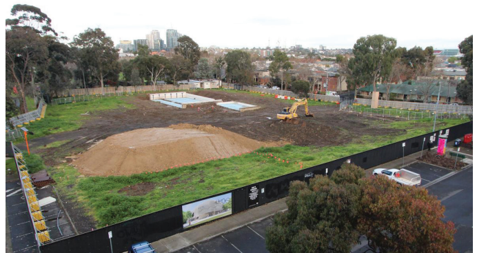
An aerial view of the construction site
