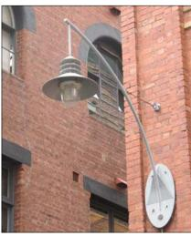
The wall-mounted light is to be used in small streets and laneways within the Central City and Docklands. The light is available in two sizes to accommodate the lights overhang requirements.
