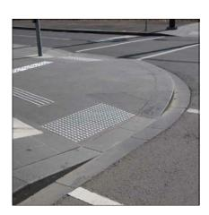
This access ramp detail is for bluestone footpaths at typical street corners within the Central City and Docklands. This detail requires wide footpaths and / or low kerbs in order to maintain preferred slopes and clearances.
