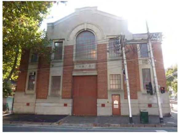
MMTB Substation, 214 Queensberry Street
