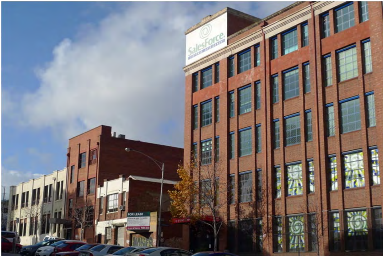
From right to left: 23-31, 19, 15-17, 11-13 Lincoln Square South and 631-645 Swanston St
