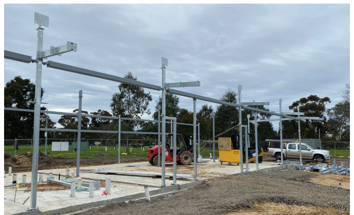
Structural steel framing in the eastern section of the pavilion
