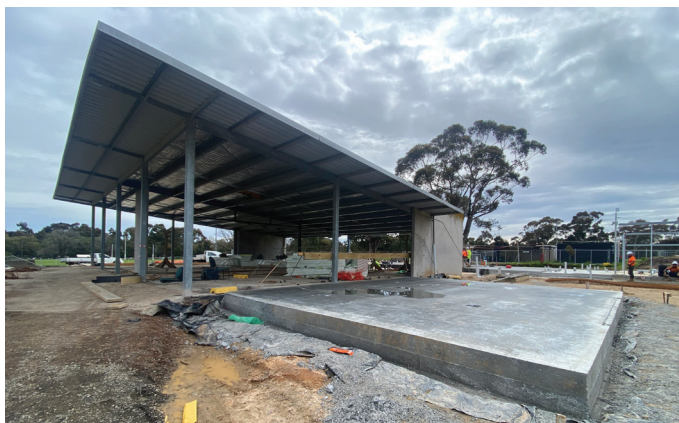
Concrete slab for the eastern section of the social room
