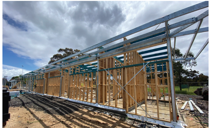
Structural steel and timber framing
