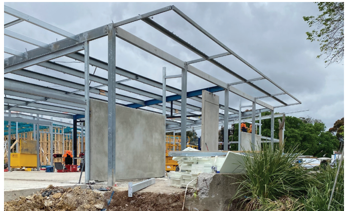
Vertical concrete panel
