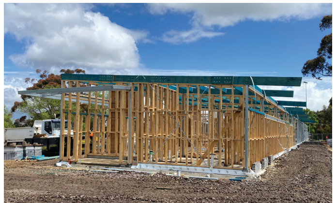
Structural steel and timber framing
