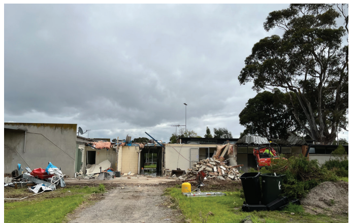
Demolition works have started
