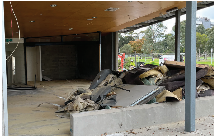
Clearing out the interior of the old pavilion
