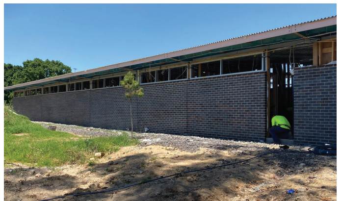
All brick work is now complete
