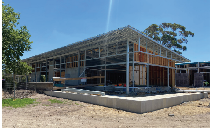
The roof and solar panels have been installed
