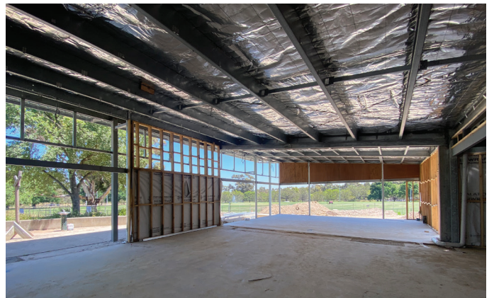
Windows will be installed in the coming weeks
