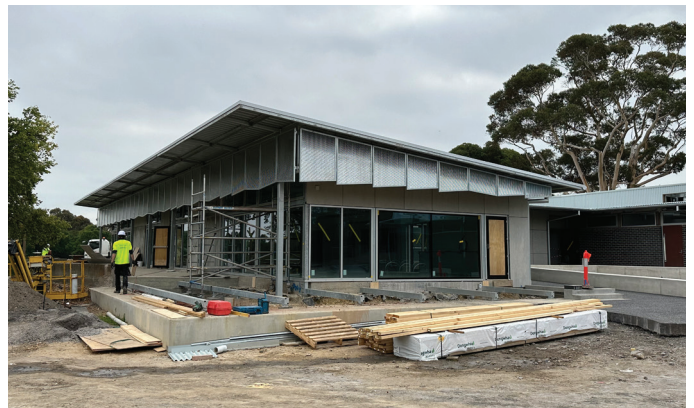
Exterior of the building
