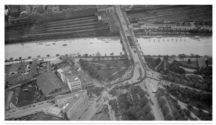
Figure 2.4: The intersection of City Road and St Kilda Road connecting at grade prior to the lowering of City Road circa 1945 Source: State Library of Victoria
