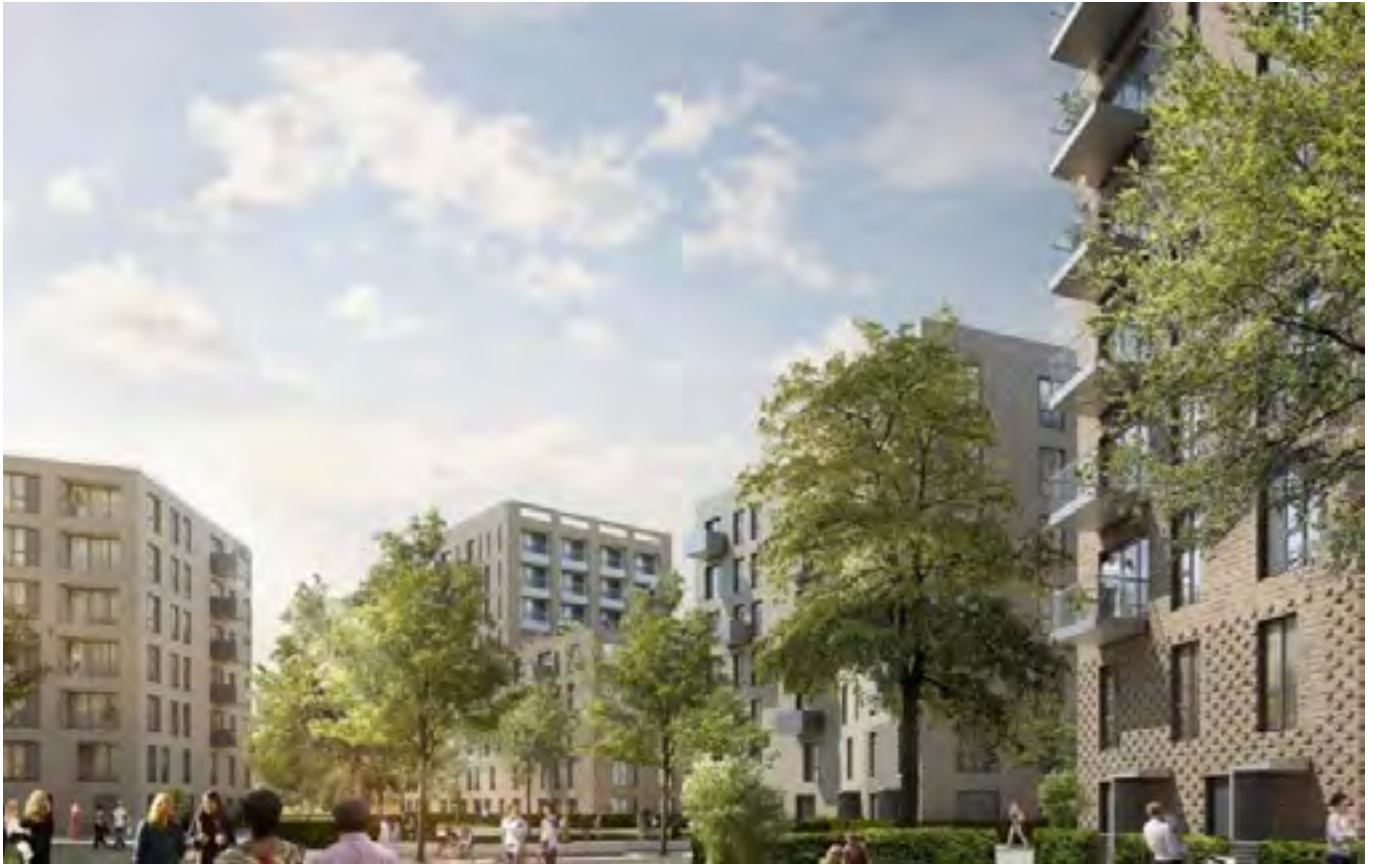
Figure 56 Lampton Road is a new neighbourhood in London that will create over 900 new homes with 50 per cent being affordable housing. Source: Notting Hill Genesis.
