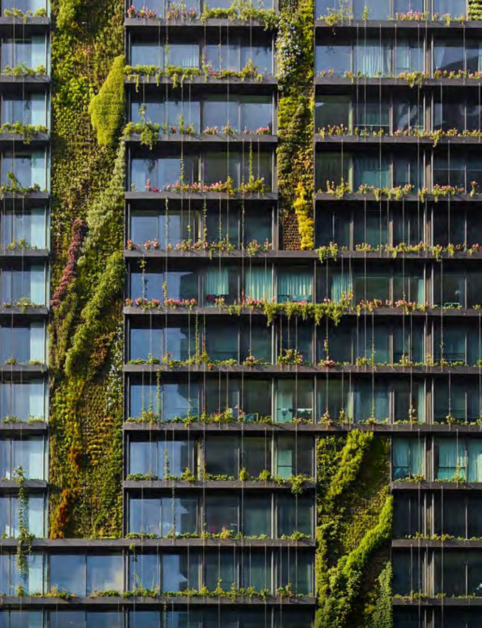
Figure 38 Example of green infrastructure incorporated into the design of One Central Park, Sydney.
