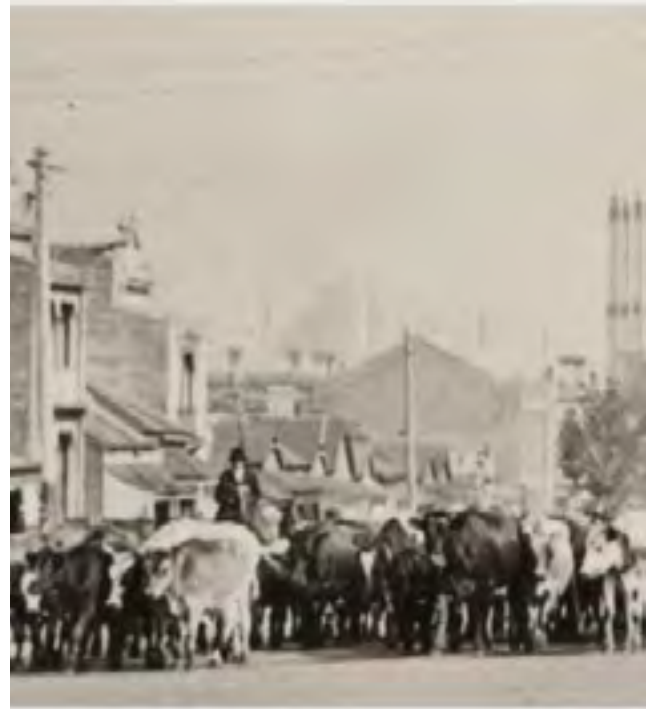
Figure 4 Droving cattle through Arden, view looking west from Haines Street, 1935.
