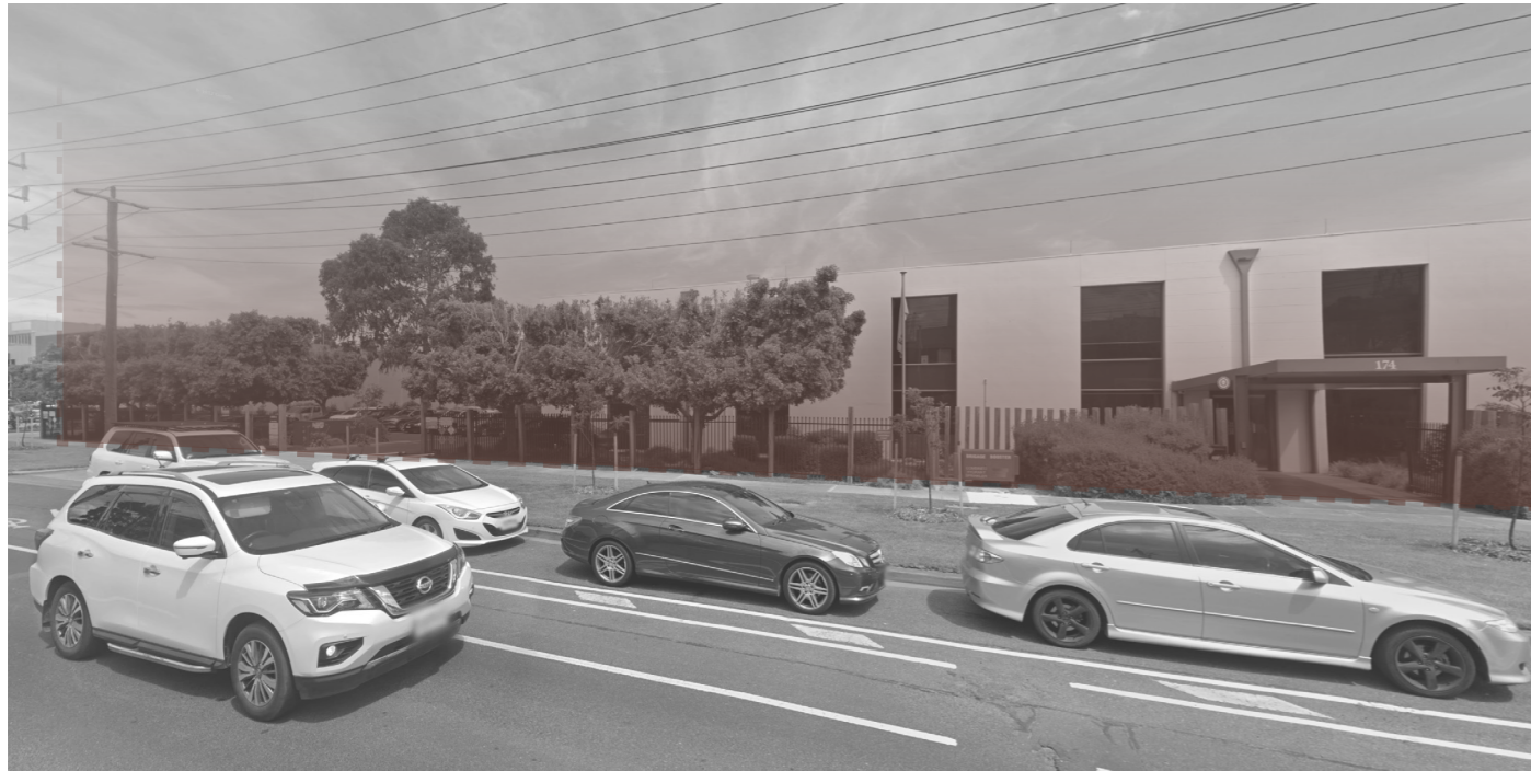
View 1 From Turner Street looking South East
