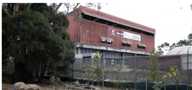
Image 36. Dynon Resource Recovery Centre
