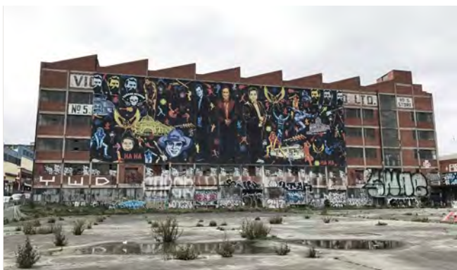
Image 15. Former Factory, Macaulay
