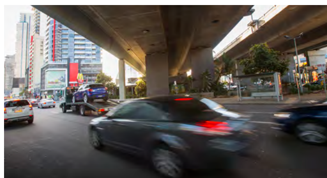
Image 25. City Road underpass
