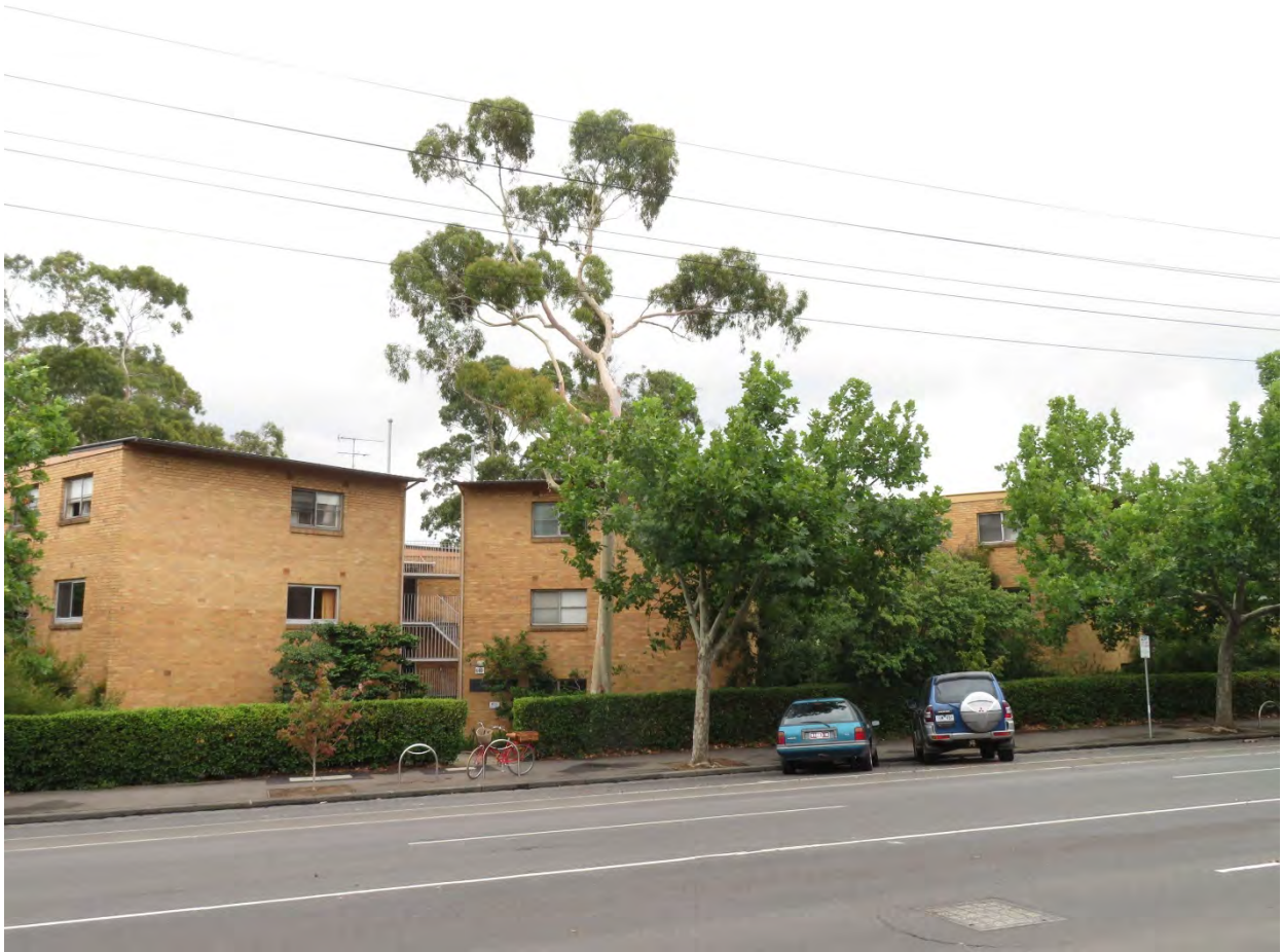
Figure 10 View of Hotham Gardens – Stage 1 from Arden Street, with angled blocks and central stairwell visible
