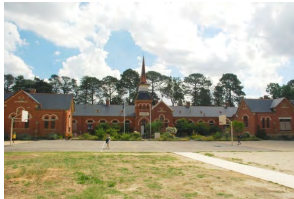
Figure 20 Beechworth Primary School No. 1560 (VHR H1718)
