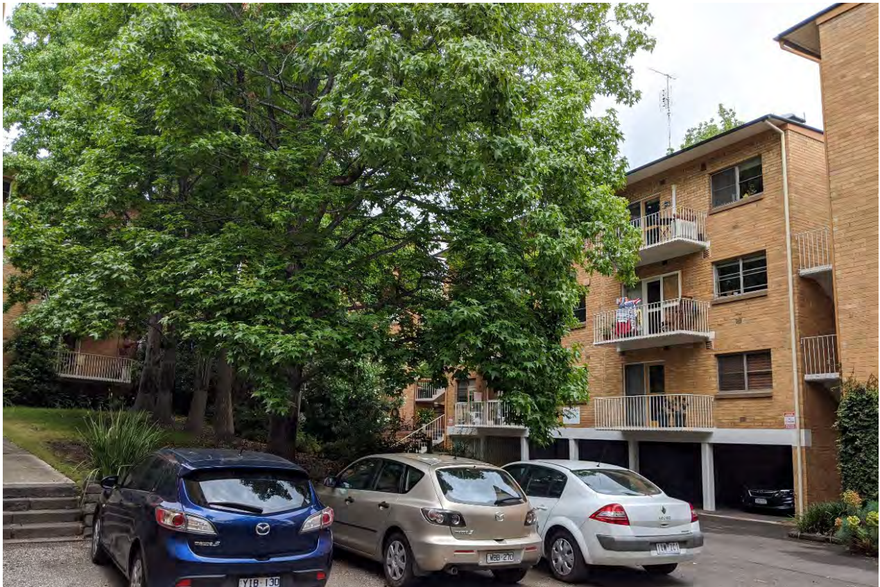
Figure 12 View of motor court and elevated garden area (Blocks B/C courtyard)
