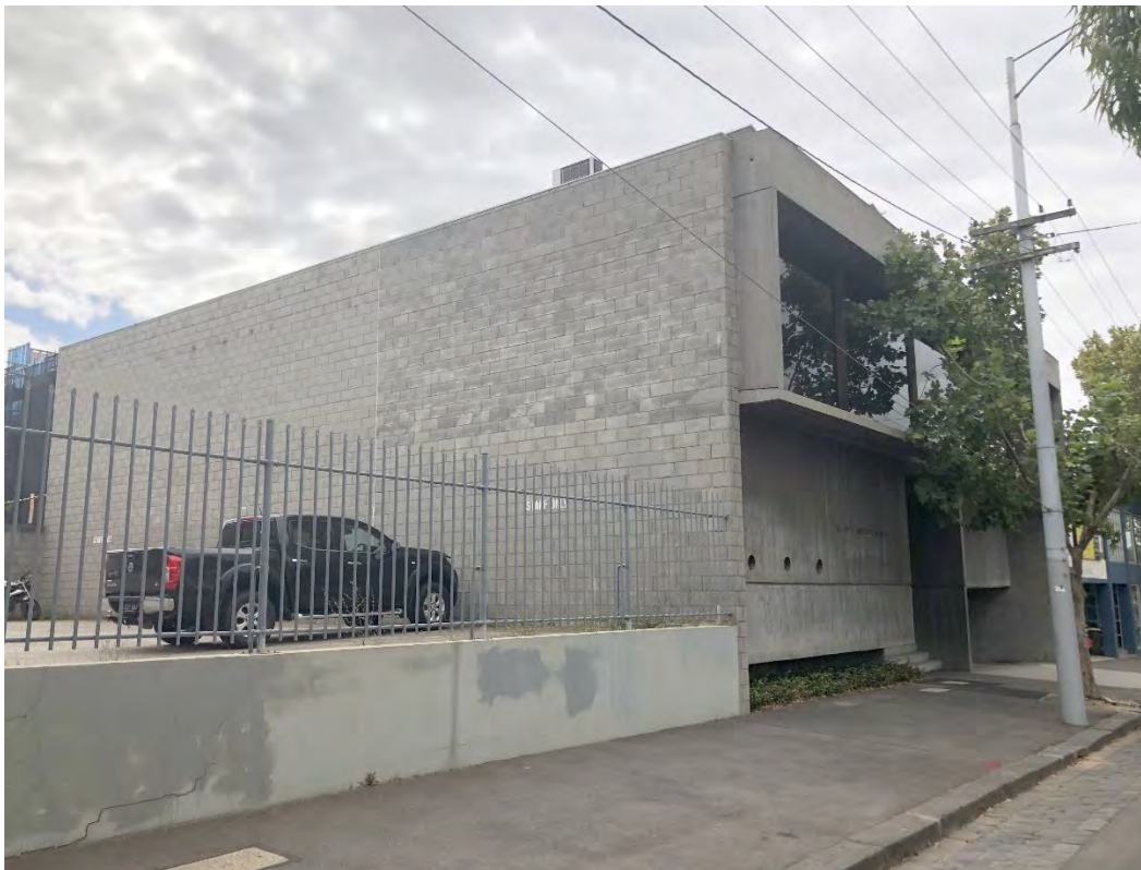
Figure 2 Former Wes Lofts office viewed from the south-east
