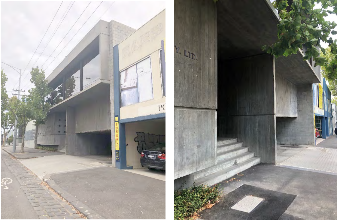
Figure 1 Former Wes Lofts office viewed from the north (left), original concrete detailing at the entry (right)
