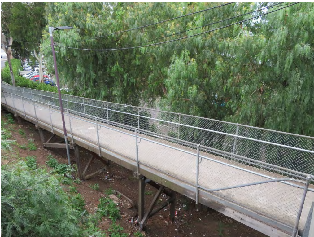
Figure 9 The ramp to the southern platform building retains original substructure
