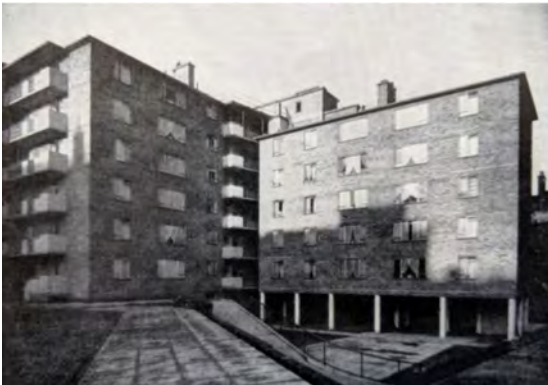
Figure 17 (Rear view) Culver and Brampton Houses , c. 1952
