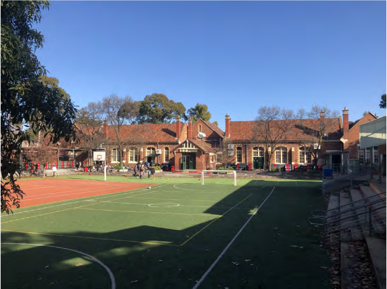
Figure 11 Rear (north) elevation of school
