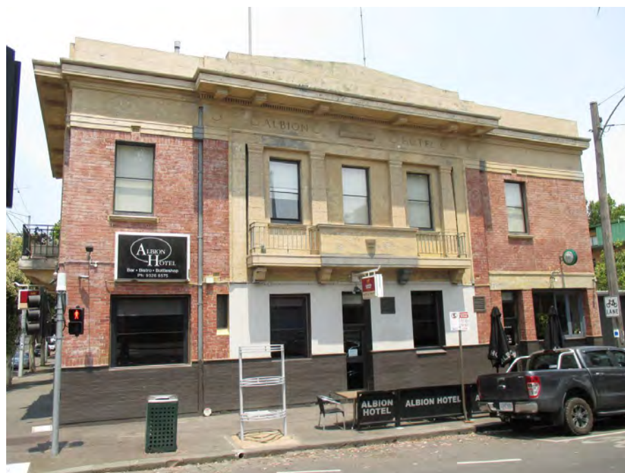
Figure 10 Albion Hotel, Haines Street elevation
