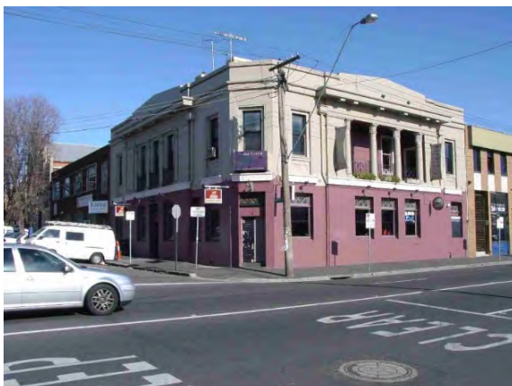
Figure 16 Town Hall Hotel, 170 Johnston Street, Fitzroy (c. 1928)
