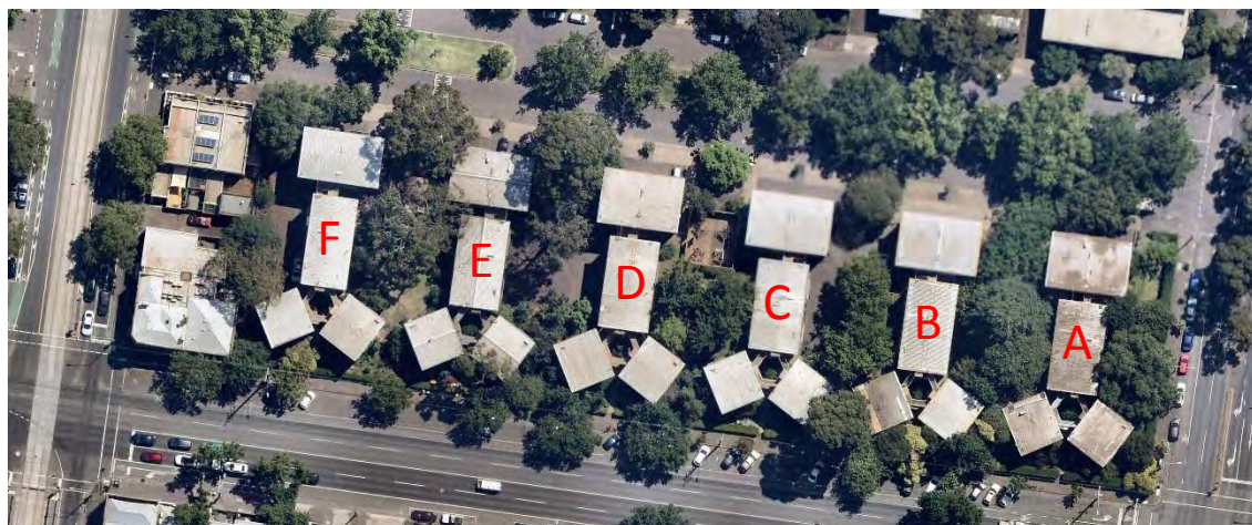
Figure 9 Recent aerial photograph of Hotham Gardens Stage 1, February 2020; blocks labelled A-F for reference
