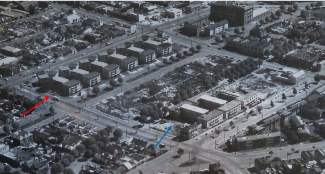
Figure 23 Oblique aerial view of Hotham Gardens development, c. 1962, looking south-west from the corner of Haines and Curzon streets to Arden Street. Stage 1 indicated by red arrow and Stage 2 (under construction) indicated by blue arrow Source: H2012.140/1040, A V Jennings albums, State Library of Victoria
