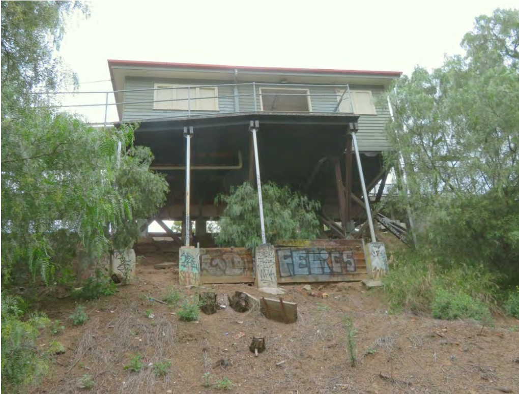
Figure 8 Northern (down side) station building viewed from the banks of the Moonee Ponds Creek
