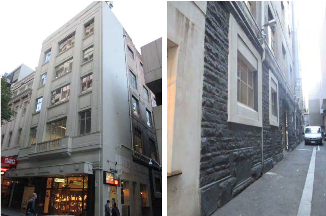
Figure 1 Subject building, south elevation (at left), and east elevation showing earlier bluestone ground floor wall (at right)
