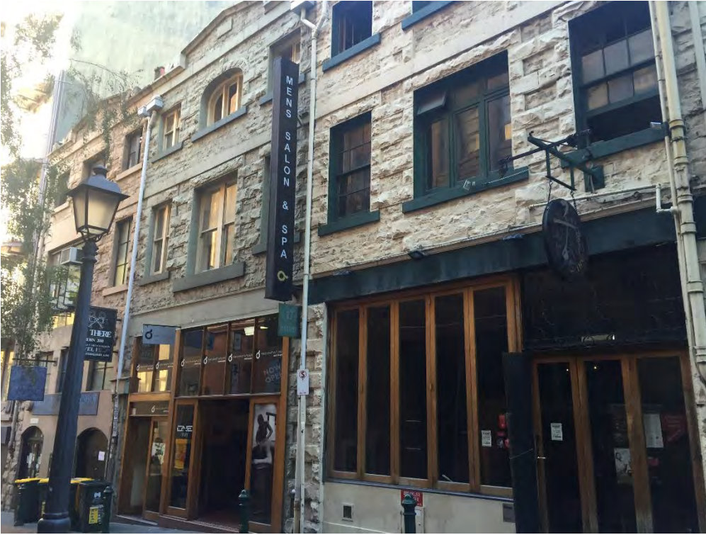
Figure 1 Subject warehouses, with 19 McKillop Street at right
