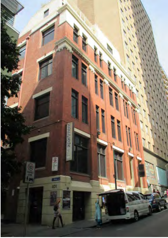
Figure 53 Subject building, looking west
