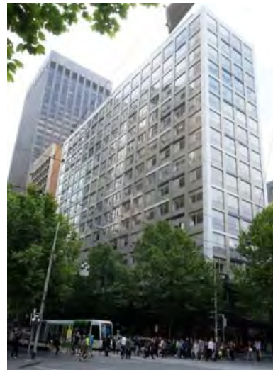
MLA Building, 308-336 Collins Street (Stephenson & Turner, 1963)
