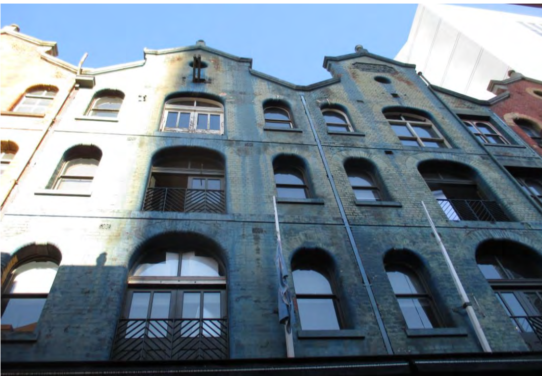
Figure 2 View of upper level facades
