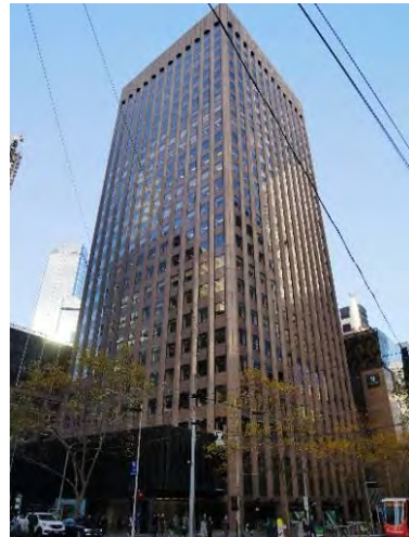
AMP Tower and St James Building Complex, 527-555 Bourke Street (Skidmore Owings & Merrill in association with Bates Smart & McCutcheon, 1965-69)
