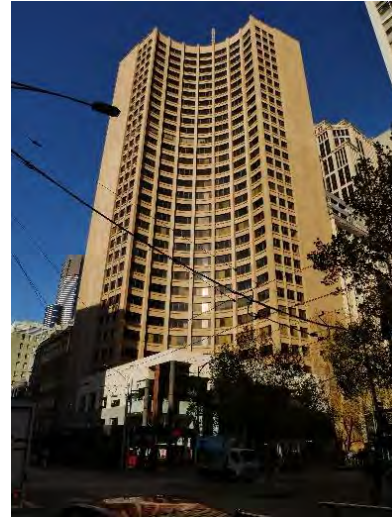
Former MLC Building, 303-317 Collins Street (Demaine, Russell, Trundle, Armstrong & Orton, c1970-1973)
