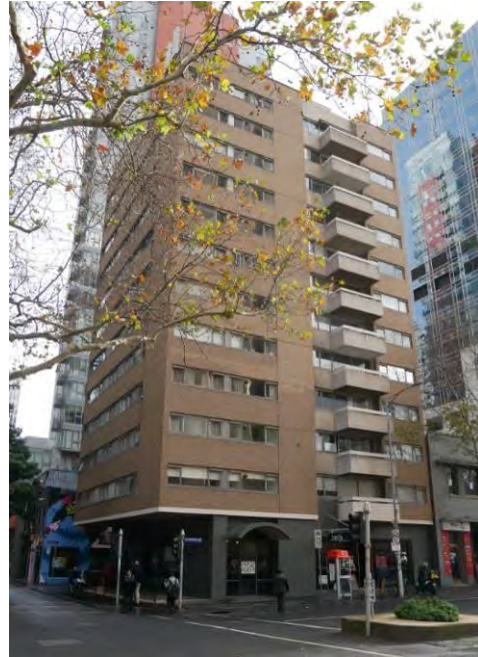
Exhibition Towers, 287-293 Exhibition Street (Kenneth McDonald & Associates, 1969-71)
