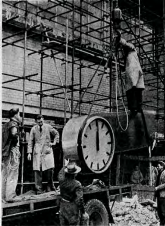
Figure 4. Extract from photograph showing the 6cw (approximately 300kg) timepiece being installed at Russell Street Exchange building in 1954. (Source: Age 23 July 1954:8)
