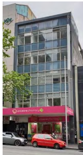
Former Coles and Garrard Building, 376-378 Bourke Street (Meldrum & Noad, 1957).
