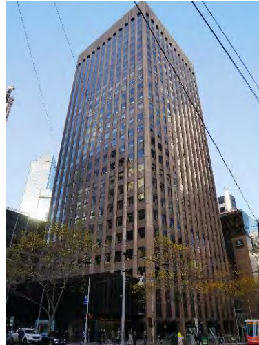
AMP Tower and St James Building Complex, 527-555 Bourke Street (Skidmore Owings & Merrill in association with Bates Smart & McCutcheon, 1965-69)
