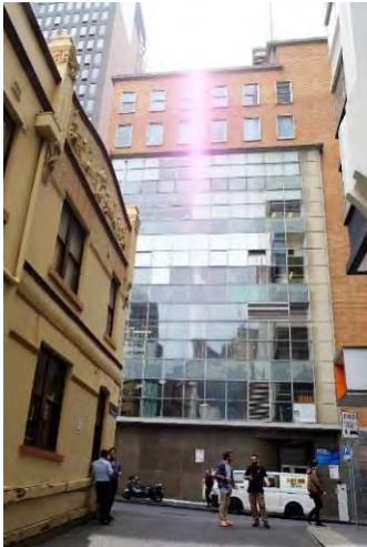
Former Batman Automatic Telephone Exchange, 376 Flinders Lane (Commonwealth Department of Works, 1957).
