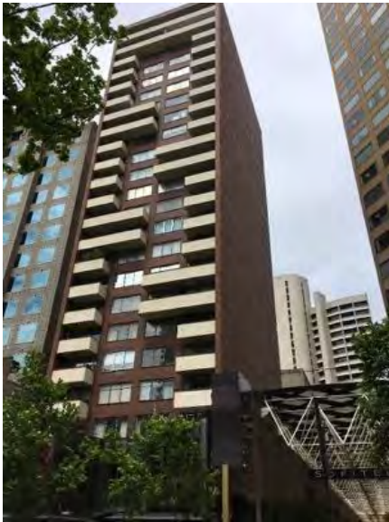
Apartment Building, 13-15 Collins Street (Kurt Popper, 1970) (Interim HO1265, & currently included as a Significant place in Collins East Precinct HO504)
