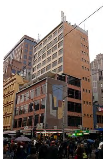
Former Hosie's Hotel, 1-5 Elizabeth Street & 288-290 Flinders Street (Mussen McKay & Potter, 1954-55), included in HO505 Flinders Gate Precinct as a Significant place.
