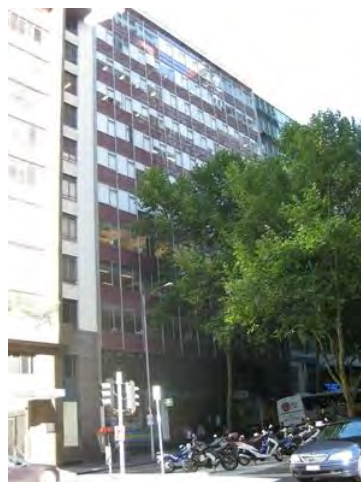
Canton Insurance Building, 43-51 Queen Street (Bates Smart & McCutcheon, 1957).
