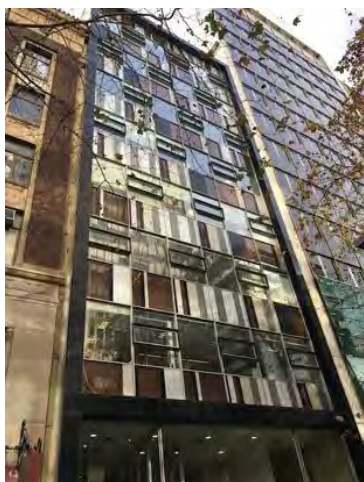
London Assurance House, 468-470 Bourke Street (Bernard Evans, 1960).
