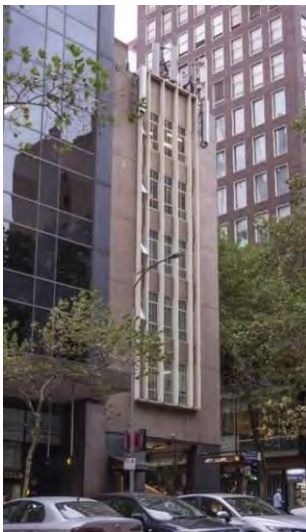
Former Ajax House, 103-105 Queen Street (HD Berry, 1956).
