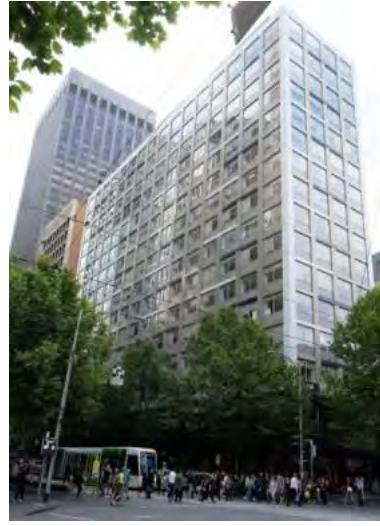
MLA Building, 308-336 Collins Street (Stephenson & Turner, 1963)
