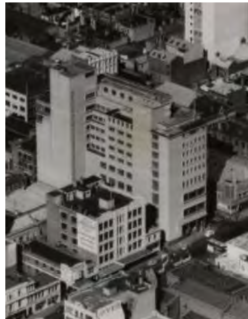
Figure 2. Aerial view of the Telephone Exchange and Postal Building, Russell Street, Melbourne, Victoria 1954-60. (Source: Charles Pratt and Airspy 1954-56, SLV copyright)
