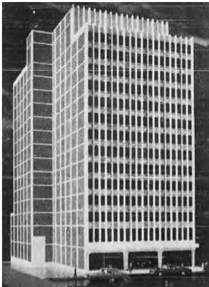
Figure 4. Rendering of 95-99 York Street, Sydney, built in 1970 using same precast concrete moulds. The secondary elevation to 168-172 Clarence Street also features same panels. The lower section of York Street façade has been since altered. (Source: Sydney Morning Herald 21 July 1969:54)
