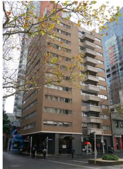
Exhibition Towers, 287-293 Exhibition Street (Kenneth McDonald & Associates, 1969-71)
