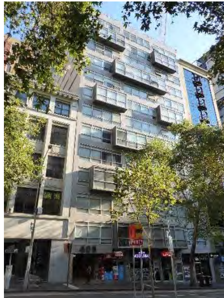
Former AMP Building, 402-408 Lonsdale Street (Bates Smart & McCutcheon, 1956-59).
