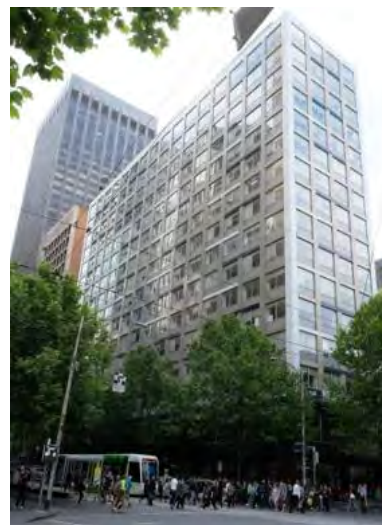
MLA Building, 308-336 Collins Street (Stephenson & Turner, 1963)
