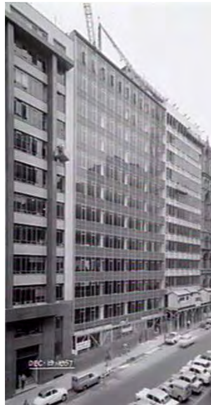
Figure 3. The Union Insurance Society of Canton Ltd building at 43-51 Queen Street (middle), and the Norwich Union Fire Insurance Society at 53-55 Queen Street (RHS), both under construction in December 1957. (Source: Fowler 1957, SLV copyright)
