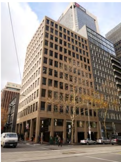
Office Building, 178-188 William Street (McIntyre McIntyre & Partners, 1972-73)
