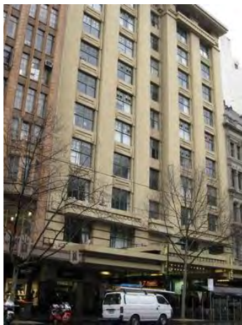
Figure 5. Capitol Arcade, 115 Swanston Street, built in 1924.
