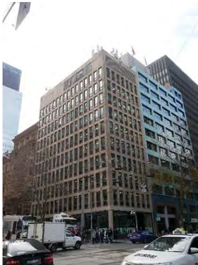
Former Guardian Building, 454-456 Collins Street (Bates Smart & McCutcheon, 1960-61)
