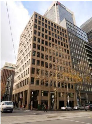
Office Building, 178-188 William Street (McIntyre McIntyre & Partners, 1972-73)
