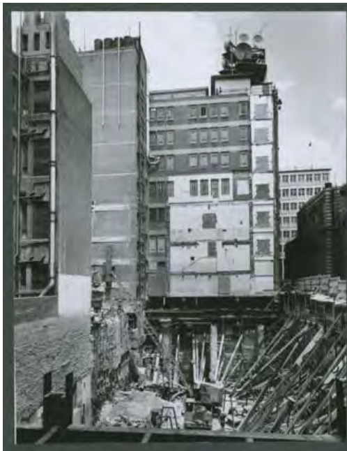
Figure 5. Excavation for the Lonsdale Telephone Exchange showing the back wall of the 1937 City West Telephone Exchange building. (Source: NAA 1966: series B6295, item: 1609B )
