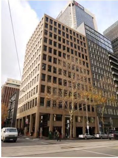
Office Building, 178-188 William Street (McIntyre McIntyre & Partners, 1972-73)
