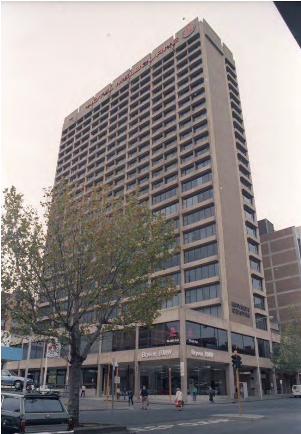
Figure 10. The subject site in 1984 (City of Melbourne Libraries online Heritage Collection, reference no. Butler 13733).
