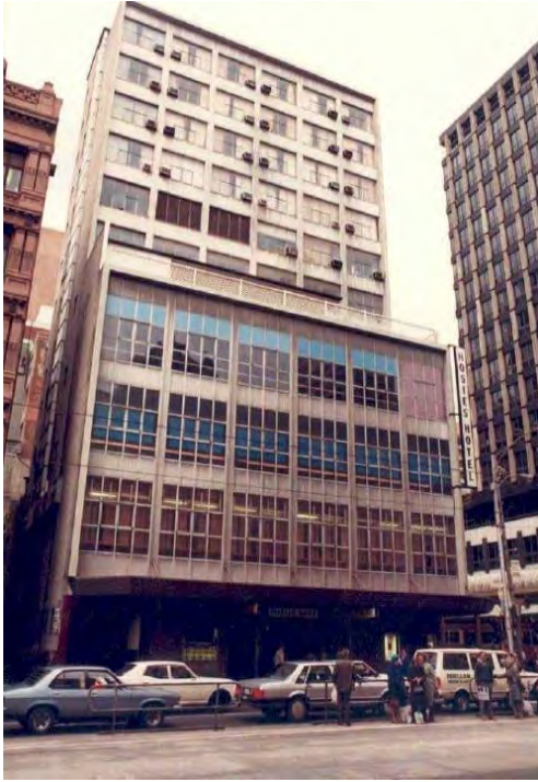
Figure 12. The hotel in 1985 (Butler 1985: Building ID Form).
