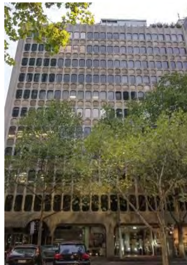
Former Law Department Building, 221-231 Queen Street (Fischer Group, 1972)
