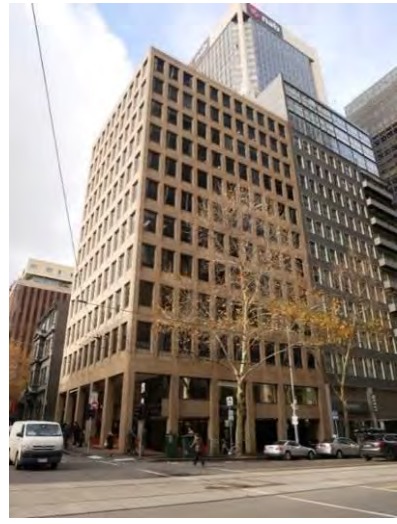
Office Building, 178-188 William Street (McIntyre McIntyre & Partners, 1972-73)
