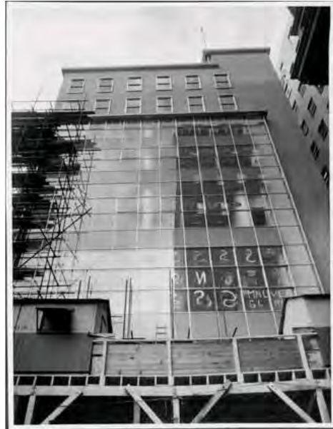
Figure 2. The subject building at completion c1957. (Source: NAA 1957-1984, Series: B6295, Item no: 9723653)
