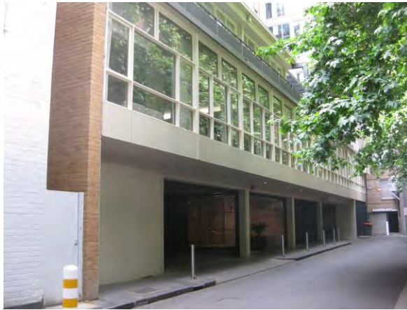
Figure 2. Lyceum Club, 2-18 Ridgway Place constructed 1959.
