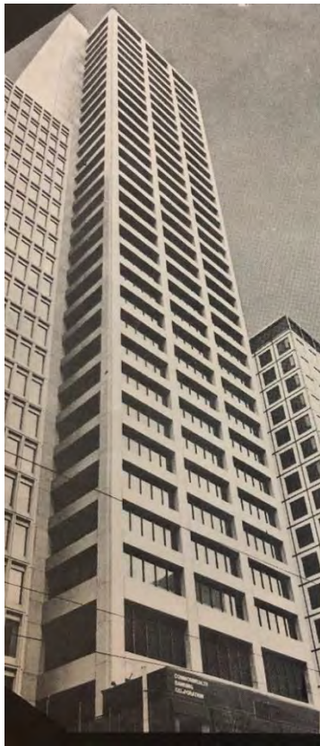
Figure 5. Illustration of the building published in the Nov/Dec 1974 issue of Architect , advertising reconstructed granite cladding by Melocco.
