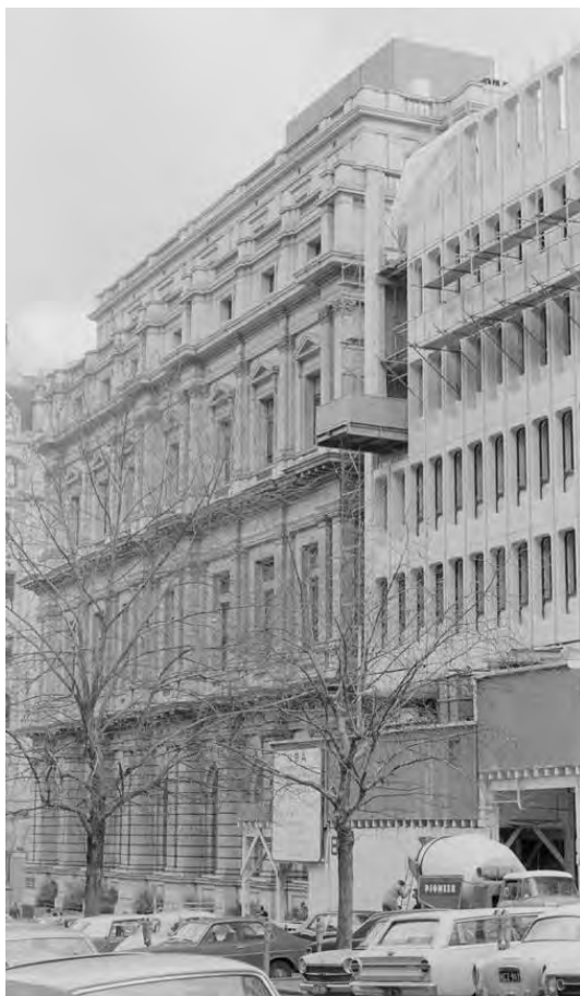
Figure 2. A c1972 photograph showing 85-91 Queen Street (right) under construction. (Source: Halla c1972, SLV copyright)
