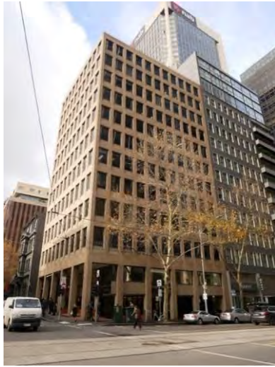
Office Building, 178-188 William Street (McIntyre McIntyre & Partners, 1972-73)
