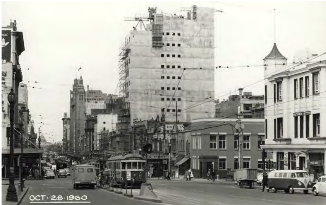
Figure 1. State Bank building, corner Little Bourke and Swanston streets under construction, 28 October 1960. (Source: Commercial Photographic Co 1960, SLV)
