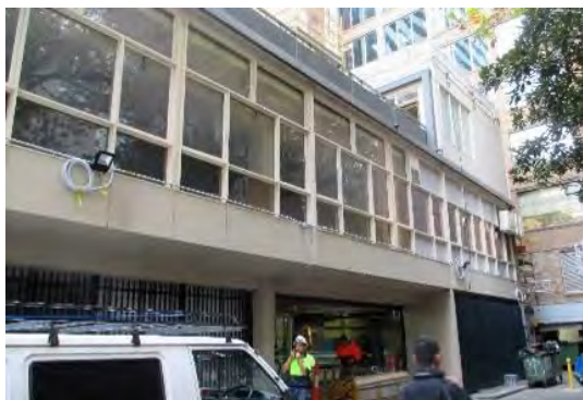
Figure 5. 2-18 Ridgeway Place, built in 1959. (Source: Context 2017)
