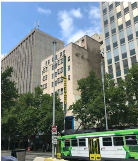
Figure 15. The Graham Hotel (GJM Heritage, February 2020)
