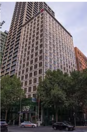
Former Legal & General House, 375-383 Collins Street (B Evans, Murphy, Berg & Hocking, 1967)
