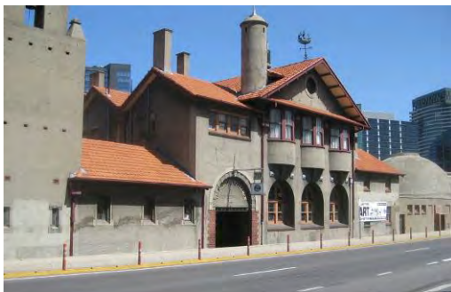
Figure 3. 717 Flinders Street, built in 1937.
