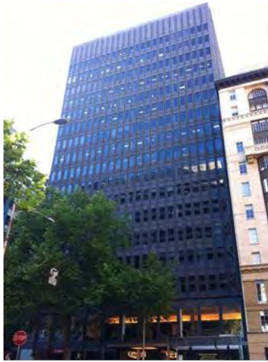
Royal Insurance Group Building, 430-442 Collins Street (Yuncken Freeman, 196)
