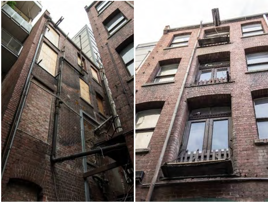
Figure 21. On the left is the rear (northern) elevation of 418-420 Bourke Street, and on the right is the front (eastern) elevation of 3 Kirks Lane. (Source: Context, January 2019)
