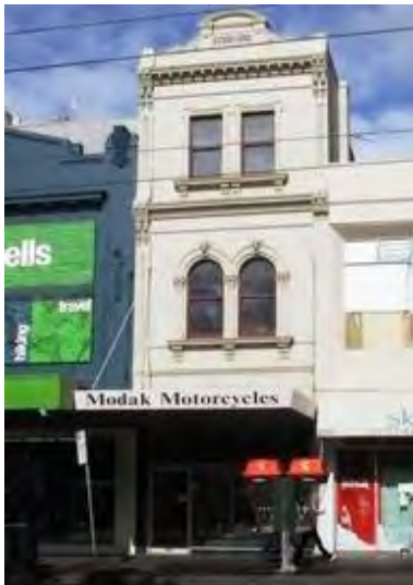
Figure 22. 299 Elizabeth Street, constructed 1885. (Source: CoMMaps)
