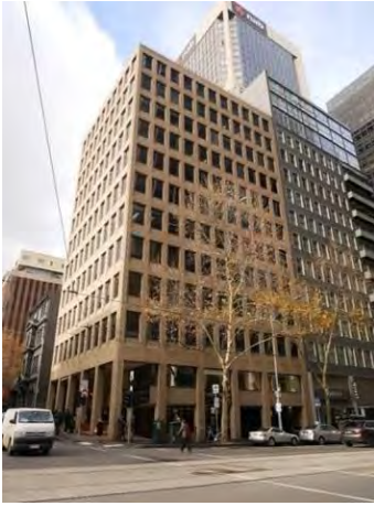
Office Building, 178-188 William Street (McIntyre McIntyre & Partners, 1972-73)
