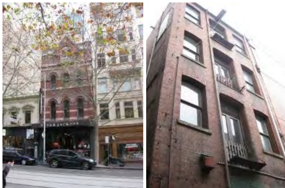
Figure 16. 418-420 Bourke Street (left) and 3 Kirks Lane, both built in 1890.
