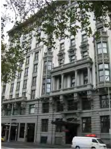
Figure 7. 318-324 Flinders Street, built in 1913.
