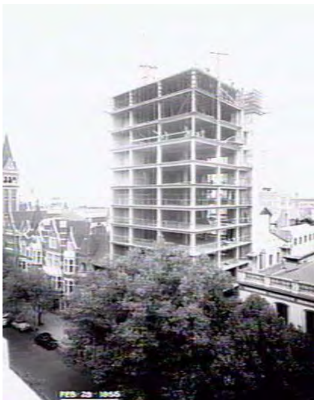
Figure 2. Construction of Gilbert Court, photo dated 28 February 1955 (SLV, Lyle Fowler, photographer, Image H92.20/5270).
