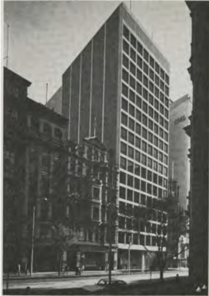
Figure 6. Photo of the Collins Street façade, published in 1970 ( Cross-Section , No. 209, Apr 1970:3).
