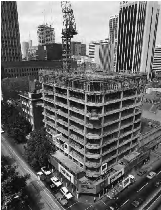
Figure 4. The corner building under construction in 1974 (SLV, Wolfgang Sievers, photographer, Image H99.50/383).
