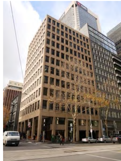
Office Building, 178-188 William Street (McIntyre McIntyre & Partners, 1972-73)
