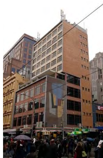
Former Hosie's Hotel, 1-5 Elizabeth Street & 288-290 Flinders Street (Mussen McKay & Potter, 1954-55), included in HO505 Flinders Gate Precinct as a Significant place.
