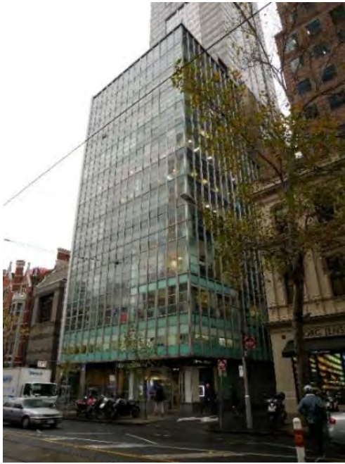
Former Gilbert Court, 100-104 Collins Street (John A La Gerche, 1954-55) included in HO504 Collins East Precinct as a Significant place.
