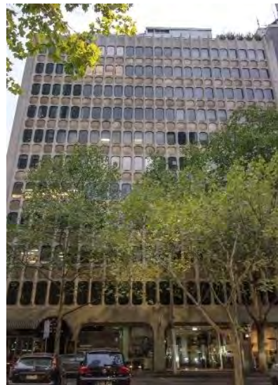
Former Law Department Building, 221-231 Queen Street (Fischer Group, 1972)
