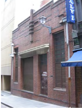
Figure 17. 23-25 George Parade, constructed in 1938. (Source: Context 2017)
