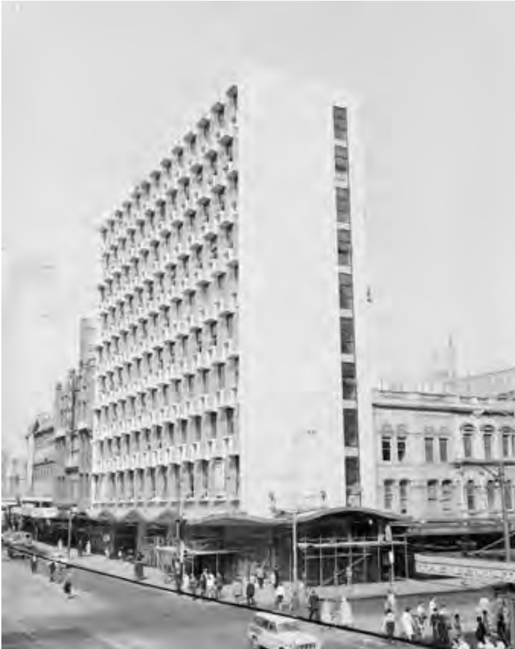
Figure 4. Royal Mail House in the final stages of completion in 1963 (NAA, Wells, photographer, A1200, L45445).
