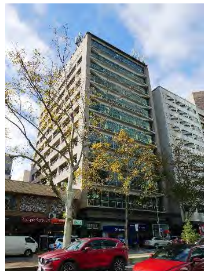
Former Australia Pacific House, 136-144 Exhibition Street (McIntyre McIntyre & Partners, 1975-78)
