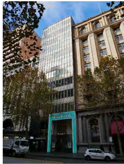
Former Bank of Adelaide Building, 265-269 Collins Street (Godfrey & Spowers, Hughes, Mewton & Lobb, 1959-60) included in HO502 The Block Precinct as a Contributory place.
