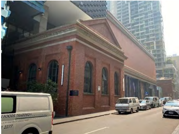
Figure 9. The Economiser Building (earlier known as the Pumping House). (Source: Context, January 2020)
