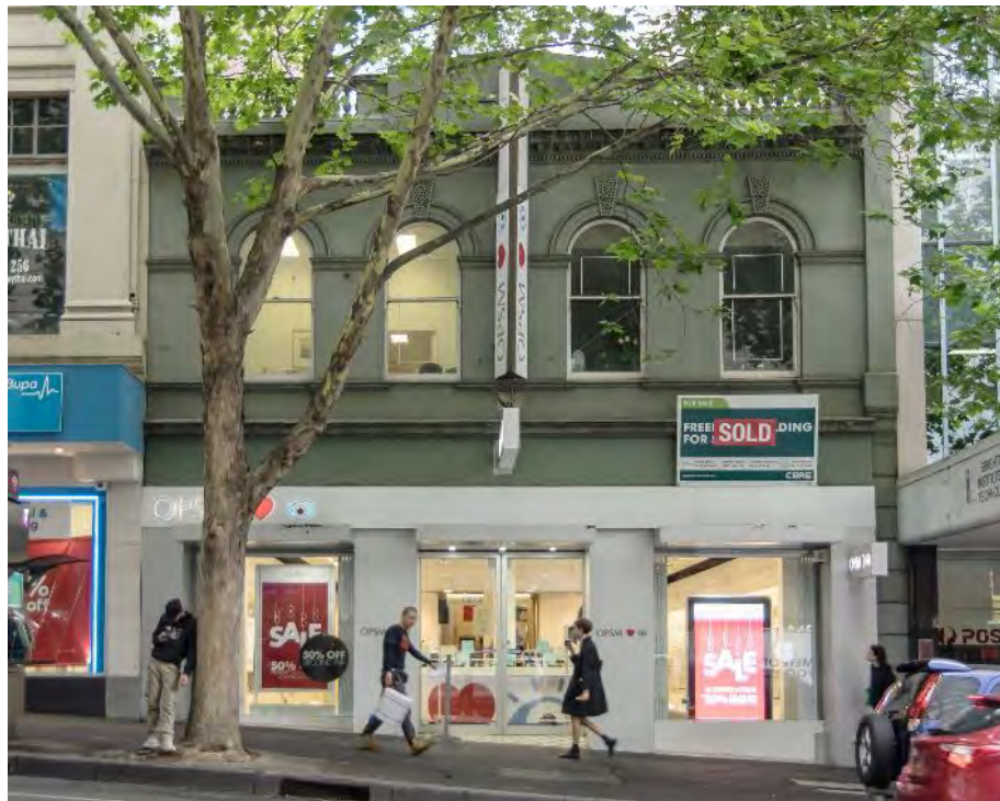
Figure 5. Bourke Street elevation of 384-386 Bourke Street. Note the unusual moulded string course that runs between each pair of upper-level windows at the sill level. (Source: Context, January 2020)
