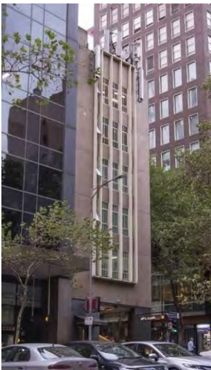
Former Ajax House, 103-105 Queen Street (HD Berry, 1956).
