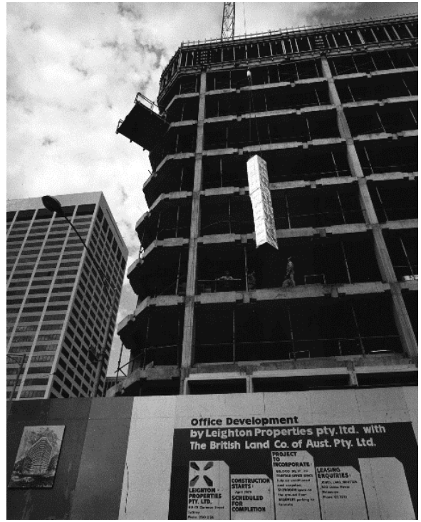
Figure 5. The building under construction in 1974. The site board states that the office development was by Leighton Properties Pty Ltd with The British Land Co. of Aust. Pty Ltd, and that construction started in April 1973 (SLV, Wolfgang Sievers, photographer, Image H99.50/384).
