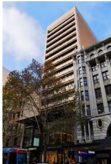
Former Commercial Banking Company of Sydney Building, 251-257 Collins Street, (Bates Smart & McCutcheon, 1974-73) included in HO502 The Block Precinct (fronting Collins Street) & HO506 (fronting Flinders Lane) (Non-contributory).
