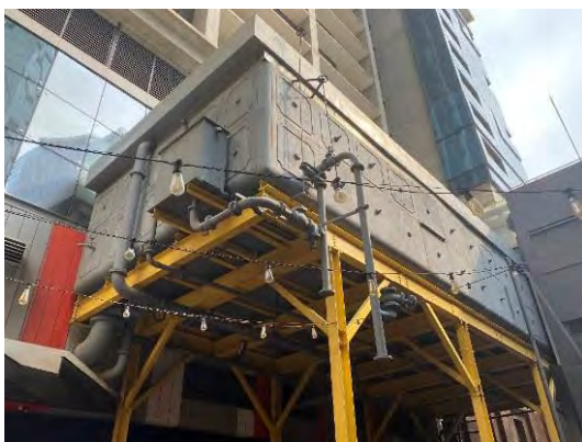
Figure 14. The Overhead Water Tank, built 1888 and relocated to this site in c1927. (Source: Context, February 2020)
