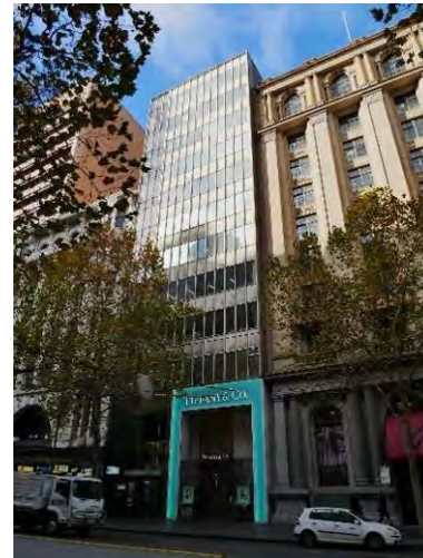
Former Bank of Adelaide Building, 265-269 Collins Street (Godfrey & Spowers, Hughes, Mewton & Lobb, 1959-60) included in HO502 The Block Precinct as a Contributory place.
