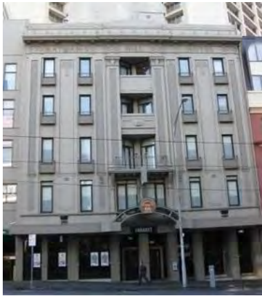
Figure 4. 66-70 Spencer Street, built in 1926-28.
