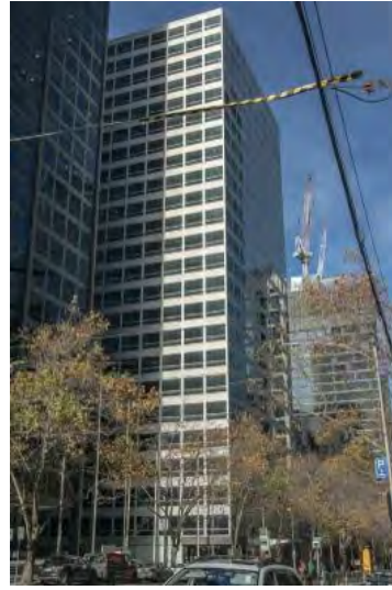
Former Dillingham Estates House, 114-128 William Street (Yuncken Freeman, 1976) (Interim HO1180)
