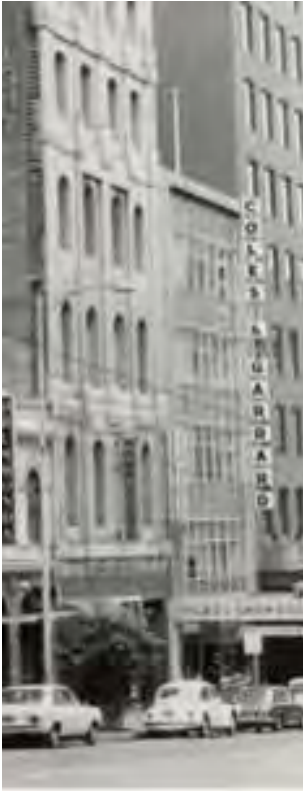
Figure 2. Showing the Coles and Garrard building (second from right-hand side) in the 1960s. (Source: Halla 1960-170, Picture Victoria copyright )
