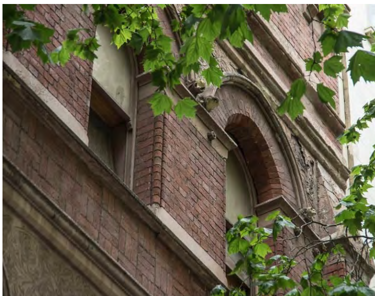
Figure 20. Detailing to the Bourke Street façade, including the rendering over the windows debossed with a leaf motif and a band of brickwork laid in chequerboard pattern between the first and second floors. (Source: Context, January 2020)
