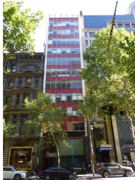
Former Allans Building, 276-278 Collins Street (Godfrey & Spowers, Hughes, Mewton & Lobb, 1956-1957) included in HO502 The Block Precinct as a Significant place.
