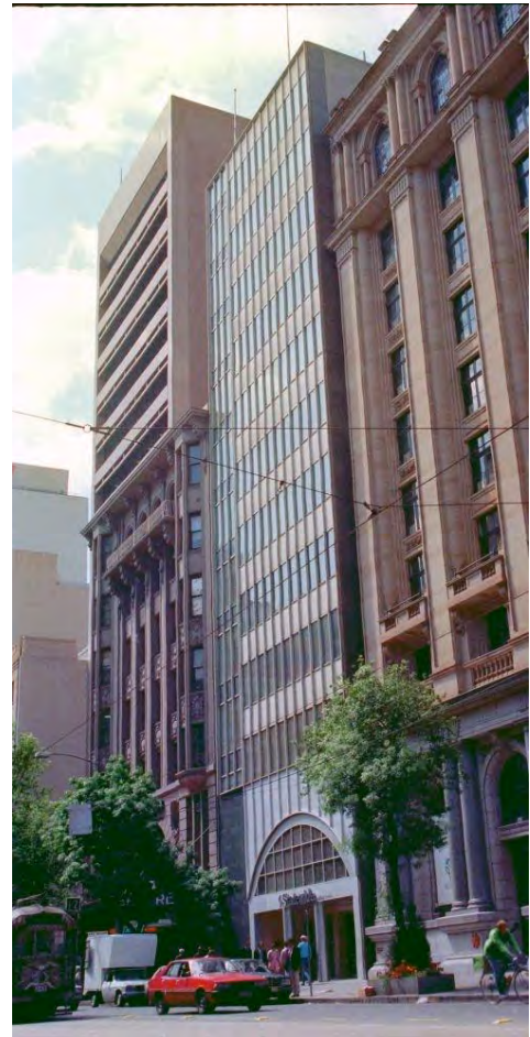
Figure 6. The building in 1984 with an altered ground floor shopfront (City of Melbourne Libraries online Heritage Collection, Reference no. Butler13528).
