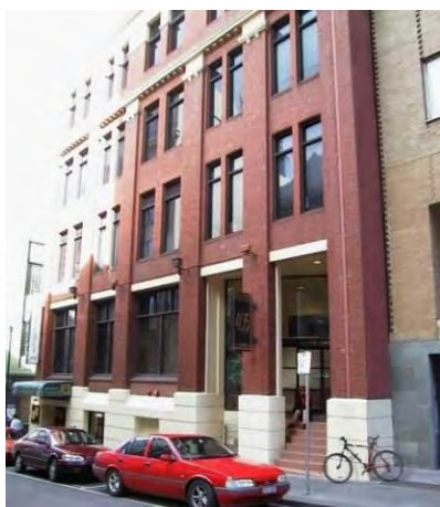
Figure 7. 401-405 Little Bourke Street, built in 1911.
