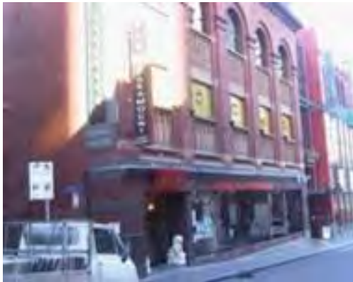
Figure 3. 91 Little Bourke Street constructed 1907. (Source: HERMES 131386)
