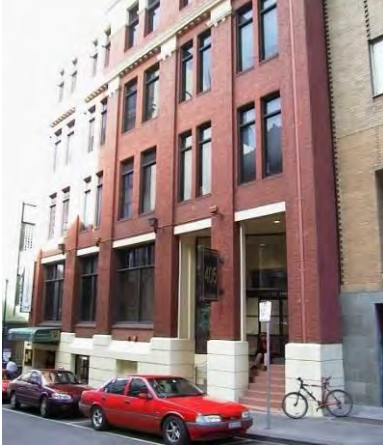
Figure 9. 401-405 Little Bourke Street, built in 1911.
