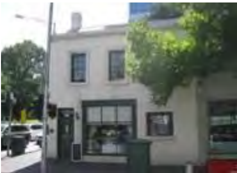
Figure 5. 330 King Street constructed 1850.
