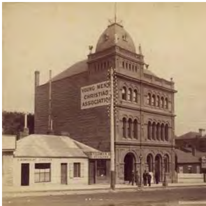
Figure 1. YMCA Building, 168 Russell Street, erected in 1878 and since demolished. (Source: SLV)
