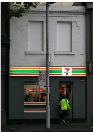
Figure 6. 261 William Street constructed 1856.
