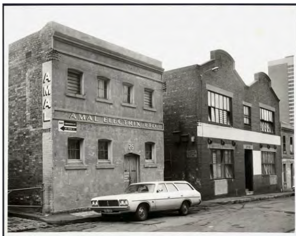
Figure 5. Image showing the subject site on the right-hand side c1980s. (Source: Australian Department of Works c1980s, SLV copyright)
