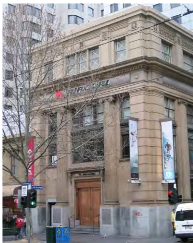
Figure 11. 219-225 Swanston Street constructed 1928.
