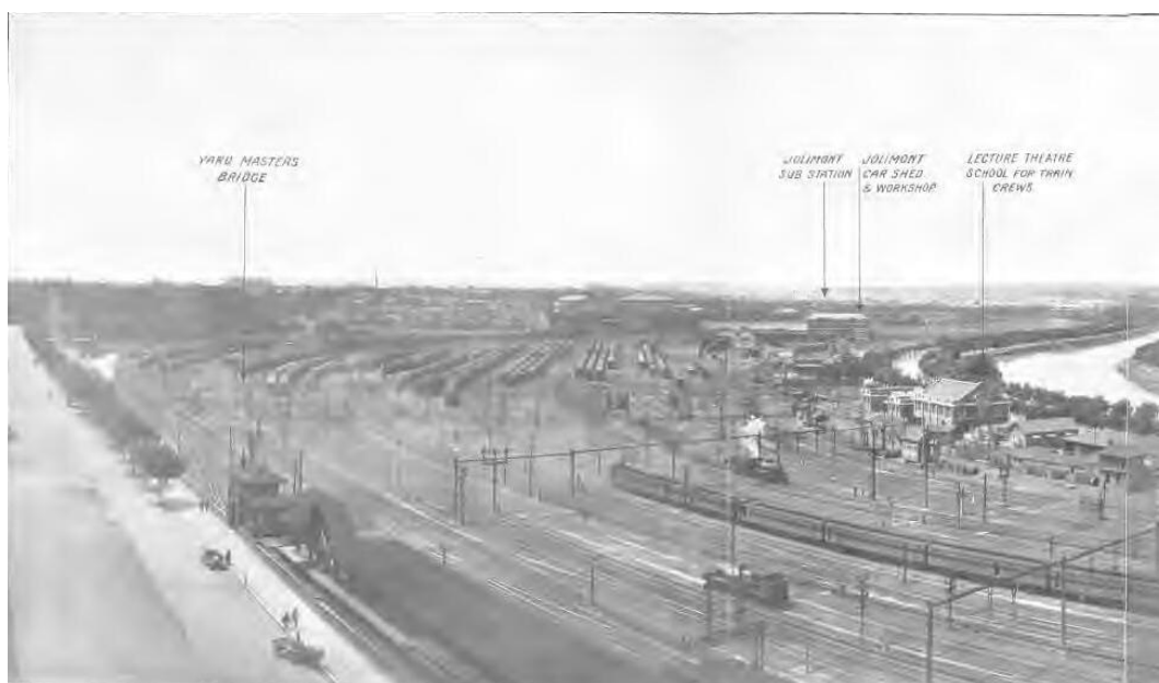
Figure 5. Part of Panoramic view of Flinders Street yard from C T Stephenson, The Electrification of the metropolitan railway system of Melbourne , 1919.
