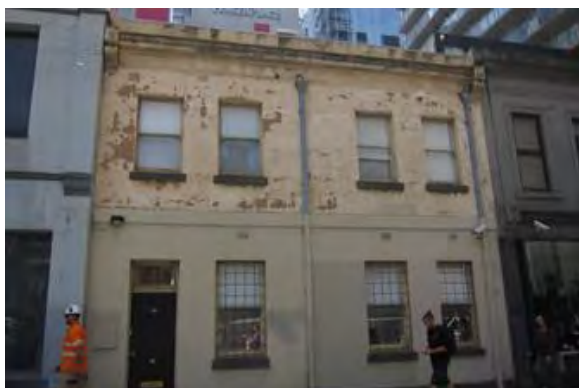
Figure 7. 120 Little Lonsdale Street constructed 1872. (Source: Context 2018)
