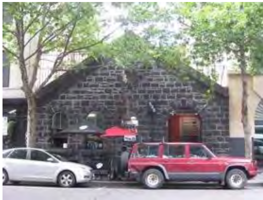
Figure 10. 585 Little Collins Street constructed 1865.
