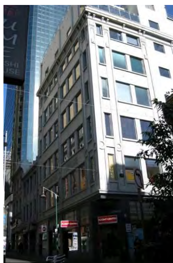
Figure 6. 386-392 Little Bourke Street, built in 1926.
