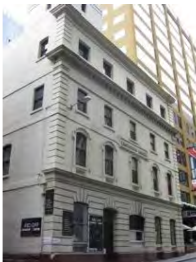
Figure 3. 538-542 Little Collins Street constructed 1878-79.
