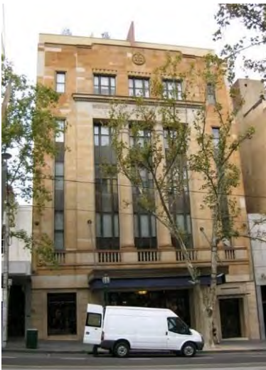
Figure 12. 181-187 Collins Street, built in 1936-37.
