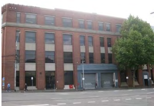
Figure 7. 258-274 Queensberry Street, Carlton, built in 1928.
