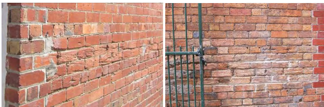
Figure 6. Vehicle marks on 27-29 Little Lonsdale (left) and a neighbouring building at 23-25 Little Lonsdale Street. (Source: Context 2018)
