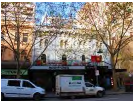
Figure 5. 209-215 Bourke Street constructed 1876. (Context 2018)
