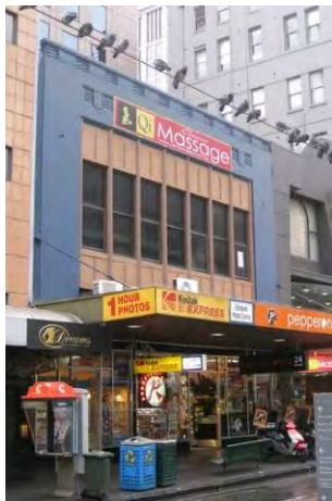
Figure 4. 7-9 Elizabeth Street, constructed in 1933.
