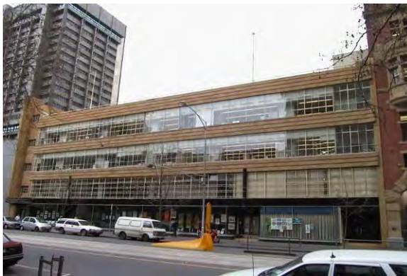
Figure 11. 546-566 Collins Street, built in 1935. (Source: iHeritage)
