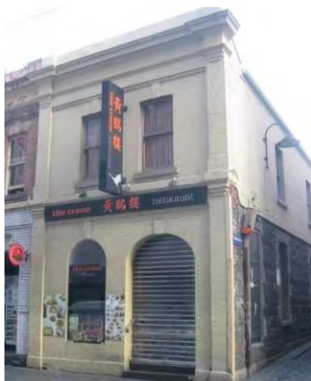
Figure 5. 212 Little Bourke Street, built in 1883.
