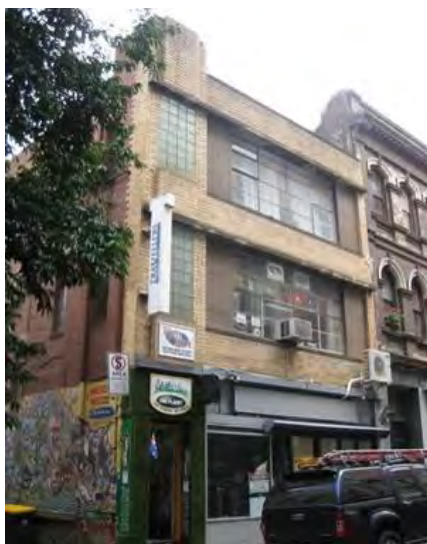
Figure 4. 361-363 Little Bourke Street, built in 1939.
