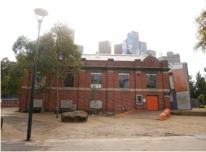
Figure 23. South elevation of the Former Princes Bridge Lecture Room. (Source: GJM Heritage May 2020)
