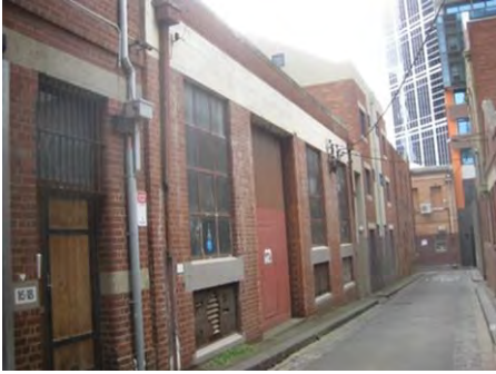
Figure 6. 12-14 Guildford Lane, constructed c 1920.
