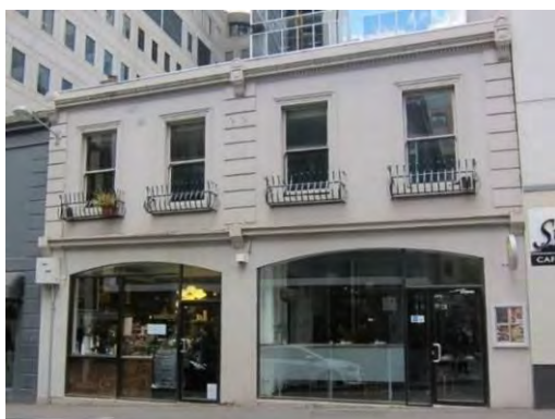
Figure 6. 470-472 Little Lonsdale Street, built in 1872. (Source: Context 2017)
