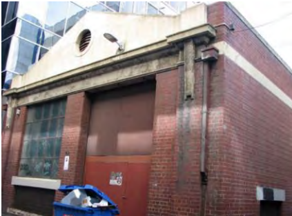
Figure 8. Substation, 10-14 Park Street constructed 1928. (Source: Context 2017)
