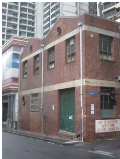
Figure 3. Substation at 620-648 Little Bourke Street constructed 1910-1925.
