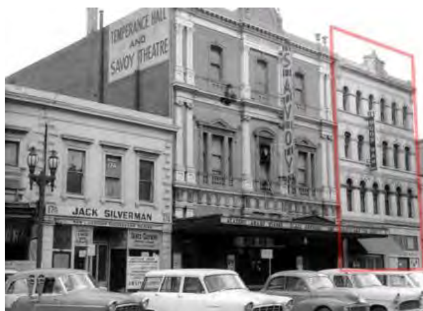
Figure 2. 166-168 Russell Street before the demolition of no 168. (Source: VHD)
