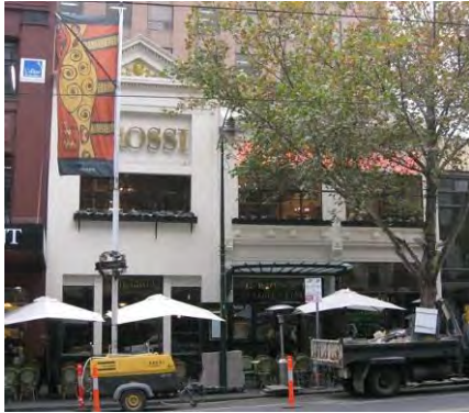
Figure 4. Grossi Florentino, 78-84 Bourke Street, built in 1860 & 1922.
