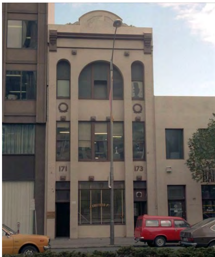
Figure 2. The subject site as it appeared in 1984. 'J Creffield' can be seen in gold lettering across the front window, indicating the firm's presence. (Source: Butler 1984 copyright )
