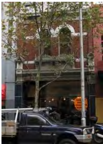
Figure 3. 309 Exhibition Street constructed 1903.
