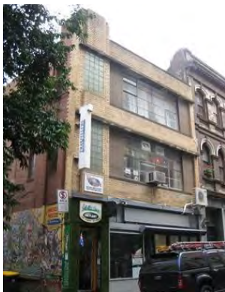
Figure 7. 361-363 Little Bourke Street, built in 1939.
