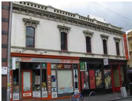
Figure 8. 189-195 Exhibition Street, built in 1882. (Source: Butler 2011)
