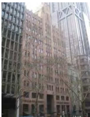
Figure 5. ACA Building, 118-126 Queen Street constructed 1936.
