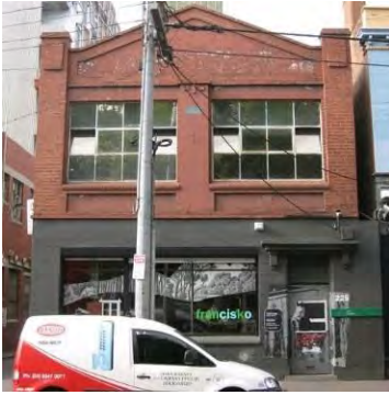
Figure 3. 225-227 Queensbury Street, Carlton, built in 1923.
