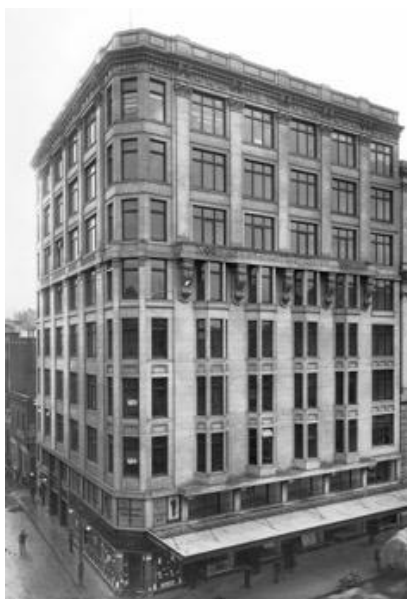
Figure 2. Signage for the Adelaide Tailoring Company is visible on the ground and first floors, at Elizabeth House (now demolished). (Source: University of Melbourne)
