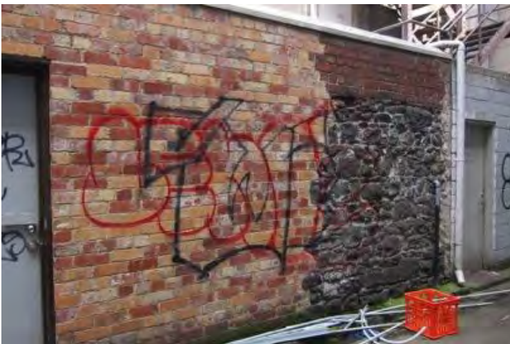
Figure 4. Bluestone section dating from the mid-nineteenth century. (Source: Context, November 2017)
