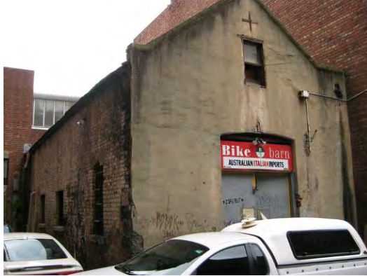
Figure 9. Rear of 361 Little Lonsdale constructed 1854.
