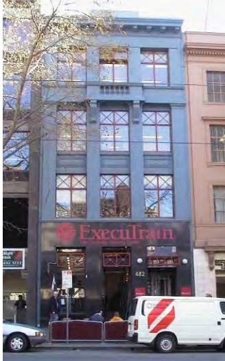
Figure 5. 482-484 Bourke Street, built in 1926. (Source: iHeitage)
