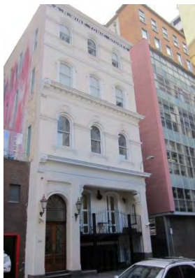
Figure 6. 384-386 Flinders Lane constructed 1885 and 1888. (Source: Context 2017)
