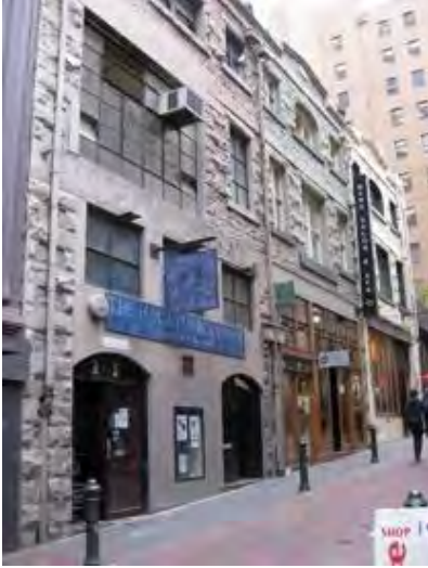
Figure 6. 15-19 McKillop Street constructed 1860.
