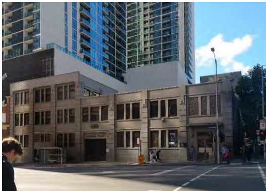
Figure 10. 594-610 Lonsdale Street, Melbourne, 1924
