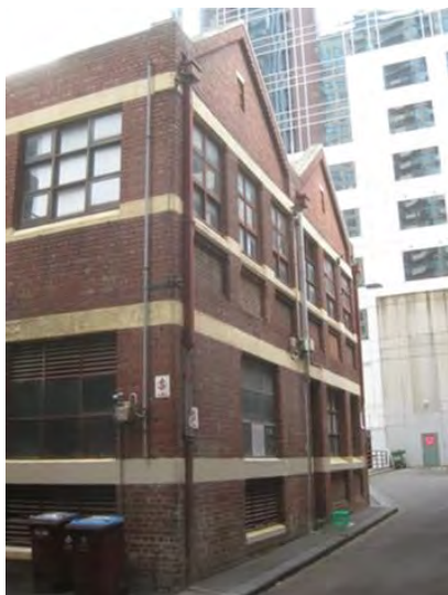
Figure 4. 1-3 Evans Lane constructed 1913.
