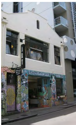
Figure 9 34-36 Little Latrobe Street, built in 1929.
