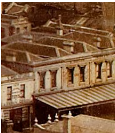
Figure 1. A group of two-storey brick shops and residences in Swanston Street, c1860. 215-217 Swanston Street is the third building from the left. (Source: Melbourne Heritage Action 2015)
