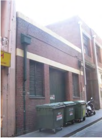
Figure 5. Substation at 28 Crossley Street, unknown built date.
