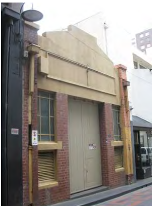
Figure 7. 21 Market Lane, unknown built date
