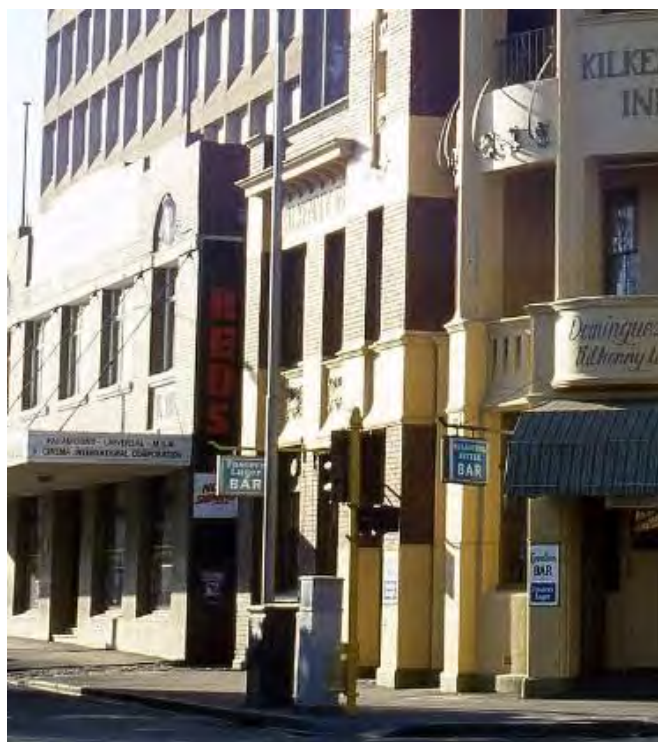
Figure 3. The subject site, to the left-hand side of Kilkenny Inn, with a sign on the cantilevered verandah reading 'Paramount Universal MGM Cinema International Corporation'. (Source: Butler 1982 copyright )
