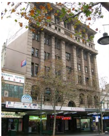
Figure 12. Curtin House, 248-258 Swanston Street, formerly the Tattersall's Club constructed 1922.
