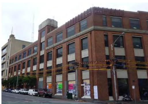
Figure 5. 258-274 Queensberry Street, Carlton, built in 1928.
