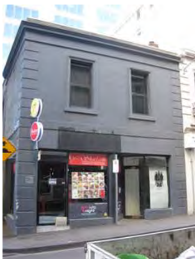
Figure 4. 474 Little Lonsdale Street constructed 1879. (Source: Context 2017)
