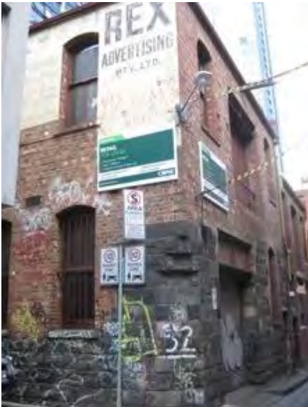
Figure 4. 32-34 Guildford Lane constructed 1908, with first floor added c1920.
