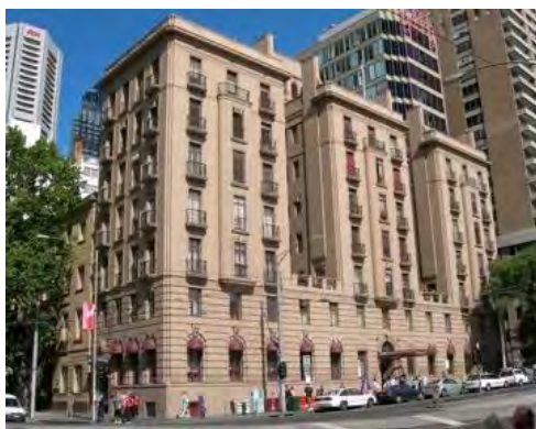
Figure 3. Alcaston House, cnr Collins and Spring streets constructed 1930. (Source: VHD)
