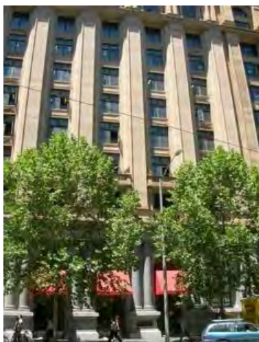
Figure 5. Former National Bank of Australasia, 271-275 Collins Street constructed 1924-25. (Source: VHD)
