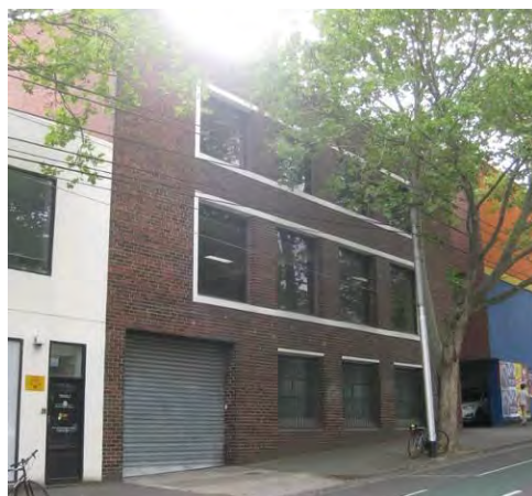
Figure 8. 198-202 Queensberry Street, Carlton, built in 1943.
