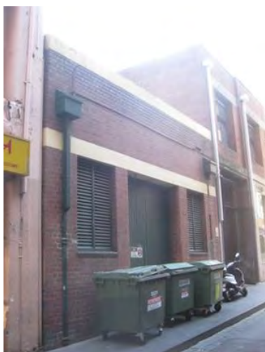
Figure 5. Substation at 28 Crossley Street, unknown build date.
