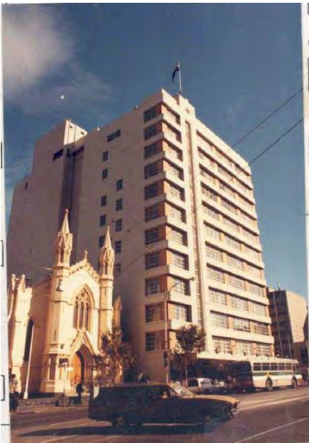
Figure 5. Manchester Unity Building in 1985, with flagpole intact . (Source: Graeme Butler, 1985 CAD Survey Hermes)
