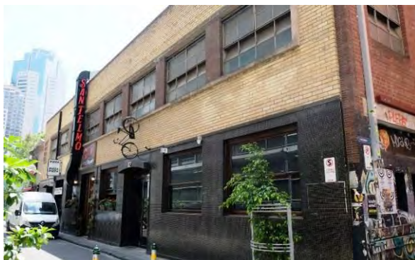
Figure 12. 12-18 Meyers Place, built in 1940. (Source: Context 2018)
