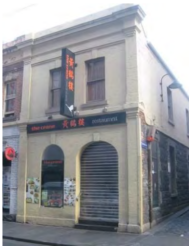
Figure 11. 212 Little Bourke Street built in 1883.
