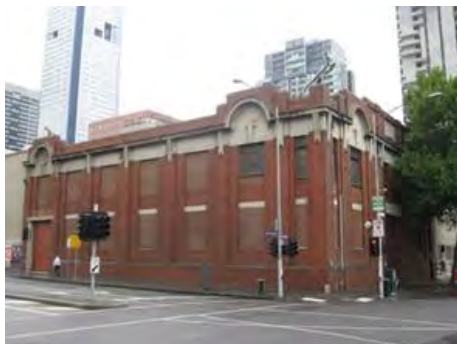
Figure 3. Substation at 651-669 Lonsdale Street constructed 1915.
