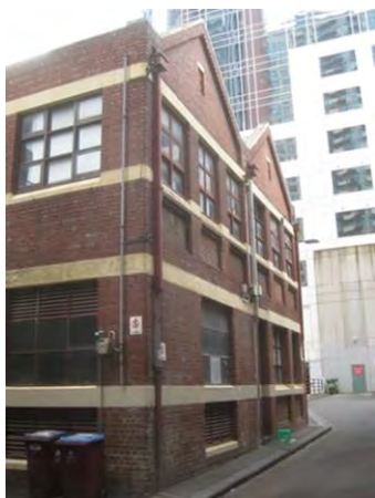
Figure 4. 1-3 Evans Lane, constructed in 1913.
