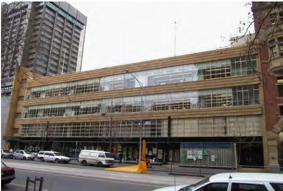
Figure 6. 546-566 Collins Street, built in 1935. (Source: iHeritage)
