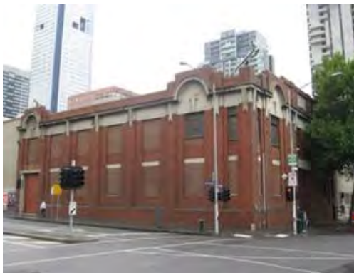
Figure 2. Substation at 651-669 Lonsdale Street constructed 1915.
