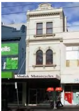
Figure 7. Former Wilson's shop & residence, 299 Elizabeth Street constructed 1885. (Source: CoMMaps)
