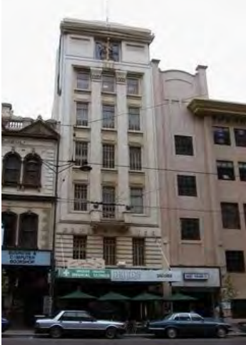
Figure 6. Druids House, 407-409 Swanston Street constructed 1927.
