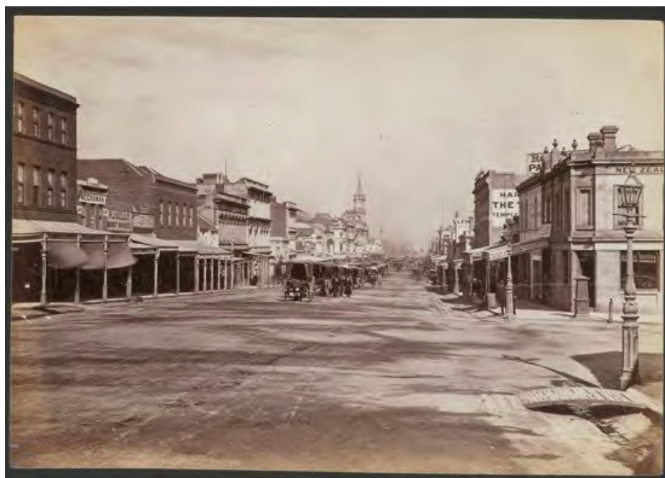
Figure 9. Swanston Street looking south from Lonsdale Street, c1870-c1880, showing on the west side (RHS) the New Zealand Commercial Hotel (formerly numbered 323-325) and Railton & Co, seedsmen (number 321). A three-storey brick building can be seen further down Swanston Street at numbers 305-307. This was demolished to make way for the current building on site, constructed in 1922. (Source: 'Swanston Street looking South' c1870-c1880, SLV).
