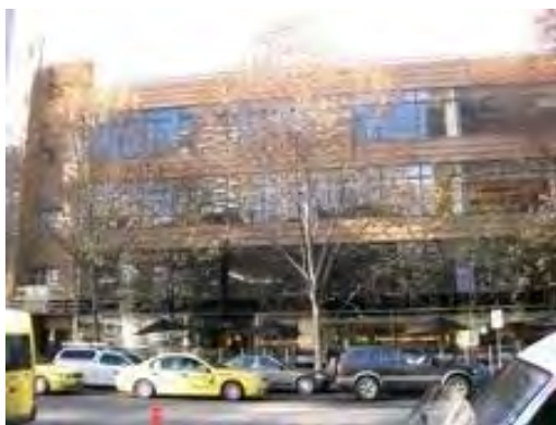
Figure 11. 546-566 Collins Street constructed in 1935.
