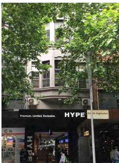
Figure 7. 139-141 Swanston Street, an interwar three storey building of 1924, formerly known as Faul's Building. (Source: Context 2017)
