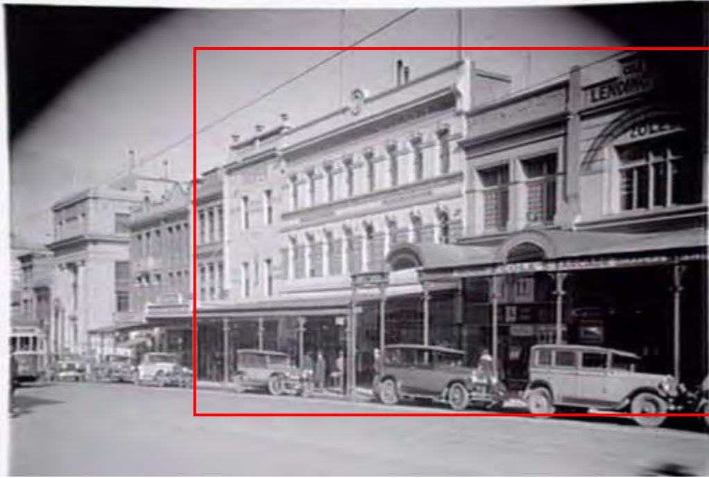
Figure 4. A view of the west side of Swanston Street, between Little Bourke and Lonsdale streets, c1930-40, showing, in rectangle from left, 237 Swanston Street; T Roper Surgical Appliances 239-241 Swanston Street; Arthur J. Veall's Electrical Radio Stores 243-249 Swanston Street; Langsford Personality Clothes 251-253 Swanston Street, and Cole's Book Arcade 255 Swanston Street. (Source: Crothers c1930-1940, SLV)
