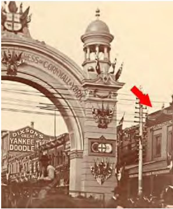
Figure 2. A section of the Citizens' Arch (1901) showing 171 Bourke Street decorated with a temporary festive pediment. The signage above the first-floor windows reads 'Lacey Chemist'. (Source: Jenkins 1901, SLV)
