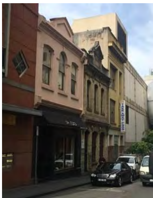
Figure 13. 277-285 Little Lonsdale Street. (Source: Context 2017).
