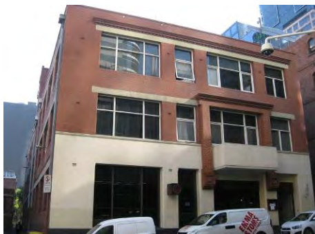
Figure 3. 562-566 Little Bourke Street, constructed in c1920s.
