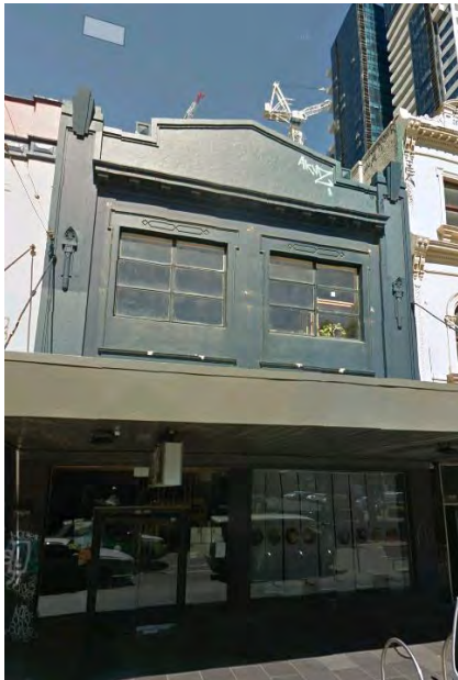
Figure 9. 295-297 Elizabeth Street, built in the early 1930s. (Source: Google 2019)
