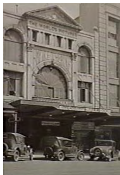
Figure 2. Photograph from 1935 showing the Empire Theatre and the interwar building at 157-163 Bourke Street (RHS). (Source: Moir 1935, SLV copyright )
