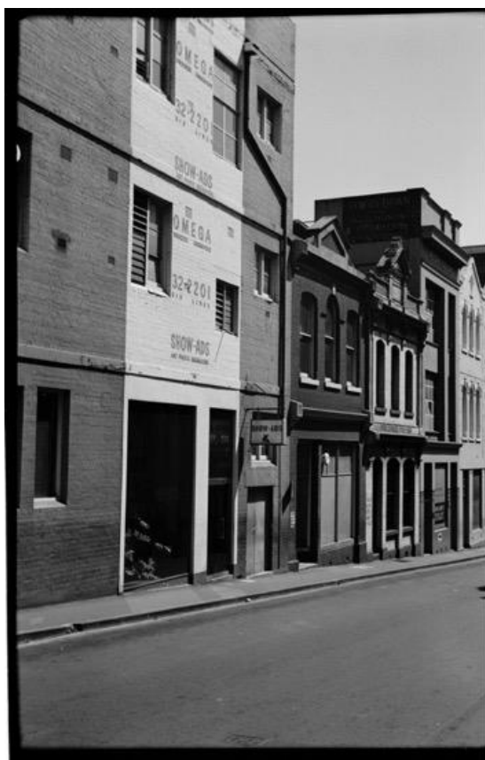
Figure 6. Little Lonsdale Street, 1968, showing numbers 277-279 (middle two-storey building) and 281 (to right of 277-279). (Source: Halla 1968, SLV)
