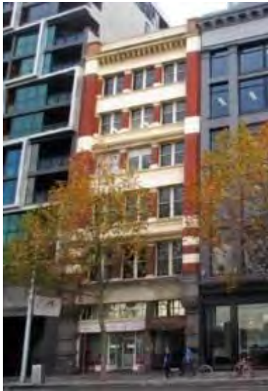
Figure 2. 100-102 Flinders Street constructed 1904. (Source: Context 2017)
