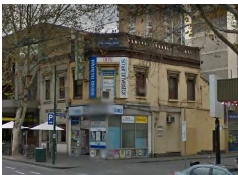
Figure 7. 51-52 Bourke Street built in the 1860s.
