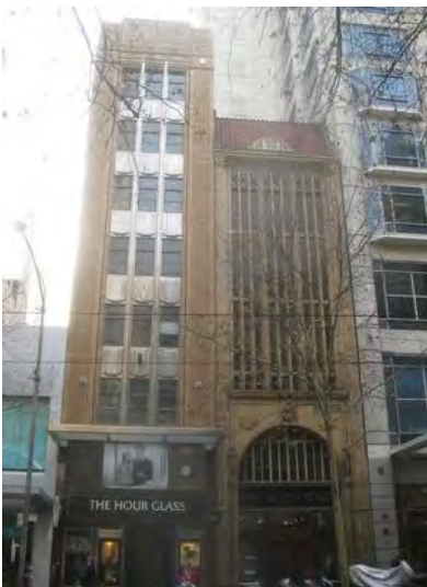
Figure 15. 250 Collins Street on right (built in 1930) and 252 Collins Street on left (built in 1935).
