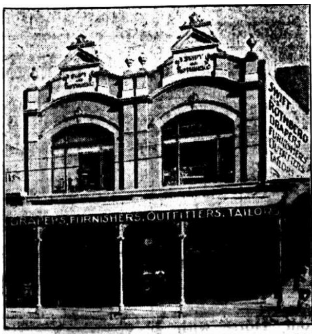
Figure 3. 257-259 Swanston Street in 1912. (Source: Herald 30 May 1912:3).
