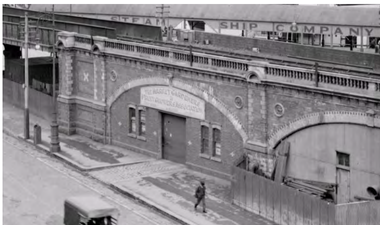
Figure 5. A close up of the viaduct buildings c1911. The buildings were removed and replaced during the 1930s, but some fabric remains, including brick and bluestone remnant walls. (Source: 'Looking east along Flinders Street', c1911, SLV)
