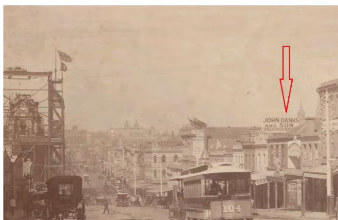
Figure 1. Showing John Danks & Son located at its original smaller building at 403 Bourke Street in the 1880s. (Source: Nettleton c1880-1890, SLV)
