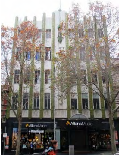
Figure 14. Former Patersons Pty Ltd 152-158 Bourke Street, built in 1934.
