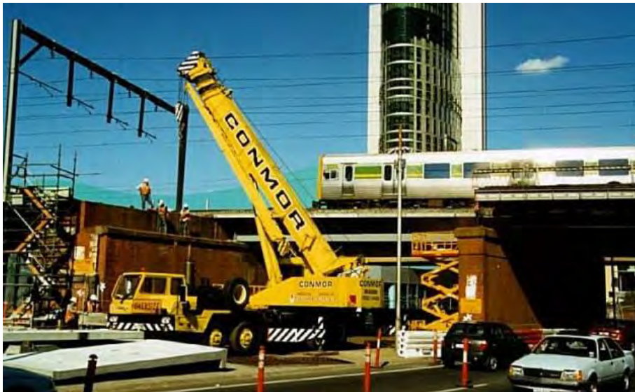
Figure 11. Re-decking of the viaduct was carried out in 2000. (Source: VICSIG 2010)
