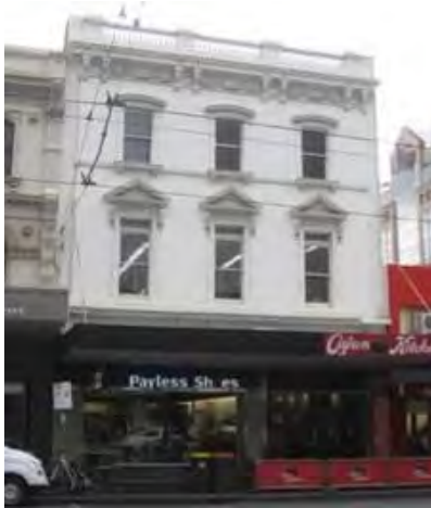
Figure 2. 136-140 Elizabeth Street constructed c1870.
