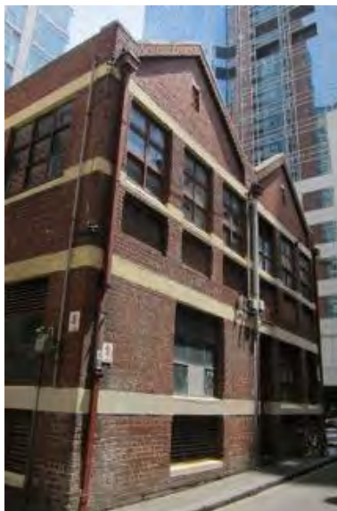
Figure 12. 1-3 Evans Lane, interwar factories converted to a substation. (Source: Context 2017)
