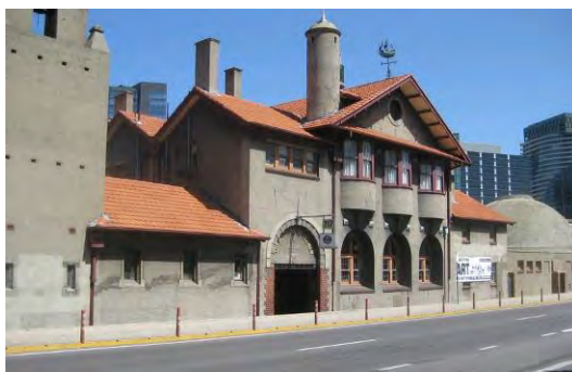
Figure 5. 717 Flinders Street, built in 1916.
