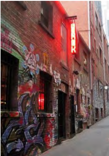
Figure 7. 11-15 Duckboard Place constructed 1885-87.
