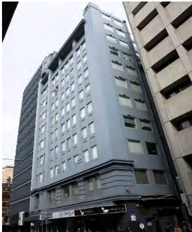
Figure 10. 345-349 Little Collins Street, 1925.
