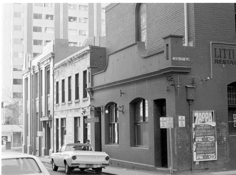
Figure 3. Showing the northern side of Little Collins Street, including the subject building (left-hand side) at 114-122 Exhibition Street in the 1960s. (Source: Halla 1960-69, SLV)
