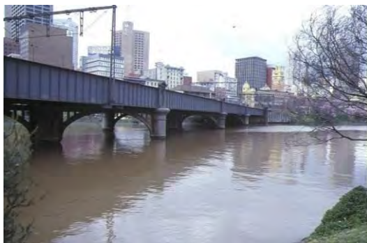
Figure 21. Sandridge Railway Line Bridge, 1886.
