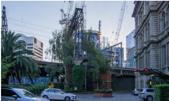
Figure 20. The former Vic Railway Administration Building (RHS) and the viaduct running behind it. (Source: Context 2019)
