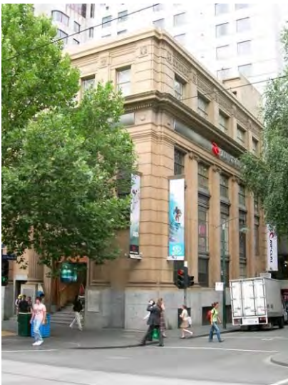
Figure 12. 119-225 Swanston Street, built in 1928 (Source: VHD)
