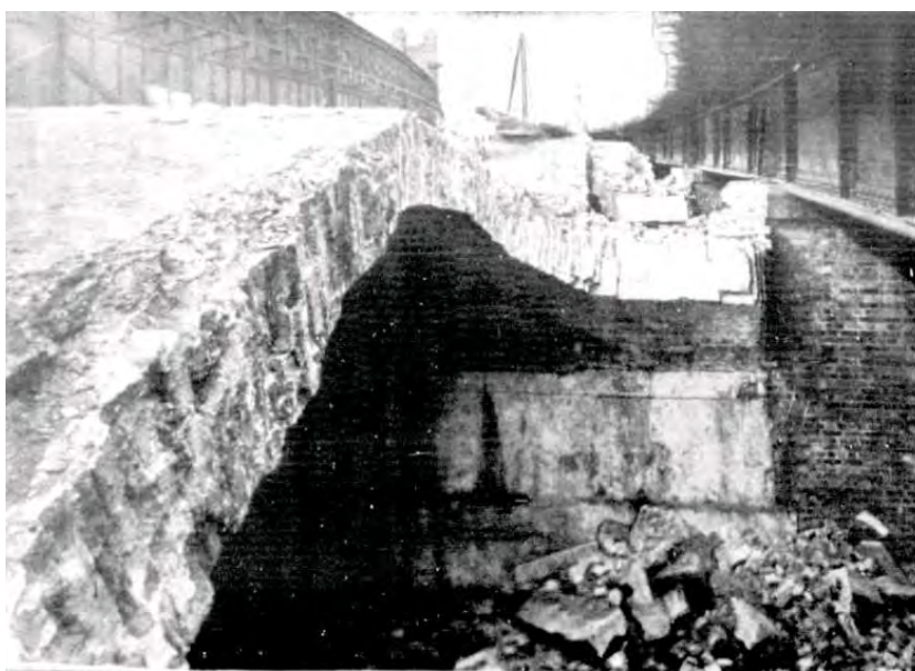
Figure 7. The arches near the Fish Market were demolished in 1916 and replaced with iron girders. ( Australasian 23 September 1916:54)
