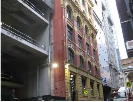
Figure 5. 164-170 Flinders Lane, now rear of 161 Collins Street, built c1910.
