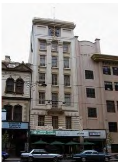
Figure 8. Druids House, 407-409 Swanston Street constructed 1927
