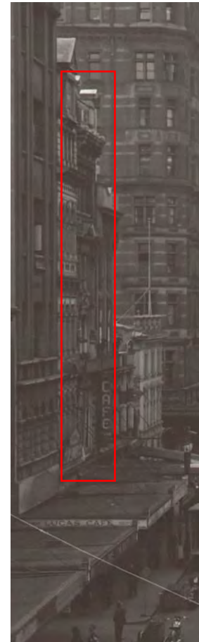
Figure 6. A 1946-53 photograph indicates a high level of soot on the façade, though original decorative façade details from 1889 appear to be intact. (Source: unknown photographer 1946-53, SLV)
