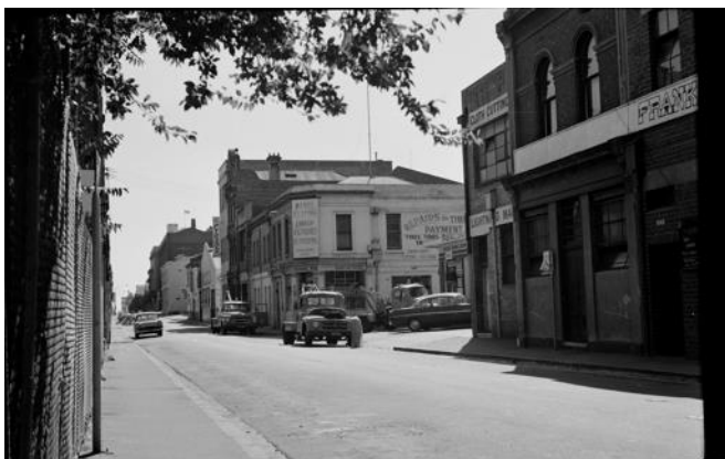
Figure 6. The second group of buildings from the RHS (in the middle of the photo) comprise 116-132 Little Lonsdale Street (HO984), then Bennetts Lane, then 134-144 and 146-148 Little Lonsdale Street, then Davisons Place, 1966. In the foreground is 100-106 Little Lonsdale Street with a car mechanic premises with a large frontage setback in front of Exploration Lane. (Source: Halla 1966, SLV)
