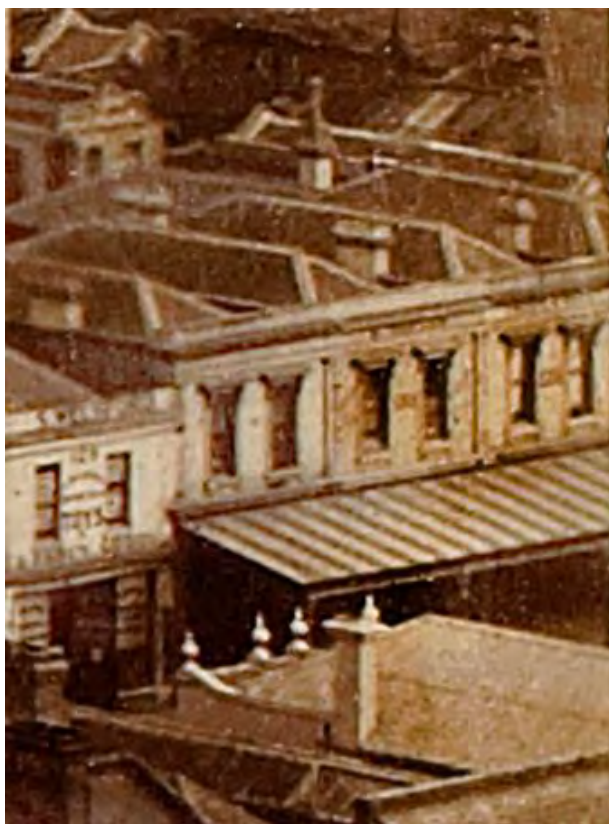
Figure 2. A group of two-storey brick shops and residences in Swanston Street, c1860. 215-217 Swanston Street is likely the third building from the left. (Source: Melbourne Heritage Action 2015)
