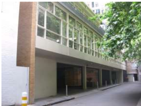
Figure 2. Lyceum Club, 2-18 Ridgway Place constructed 1959.
