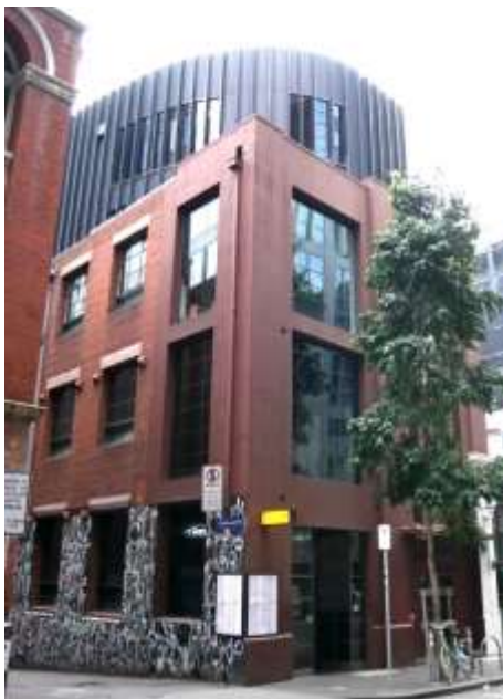
Figure 5 91-93 Flinders Lane, Melbourne
