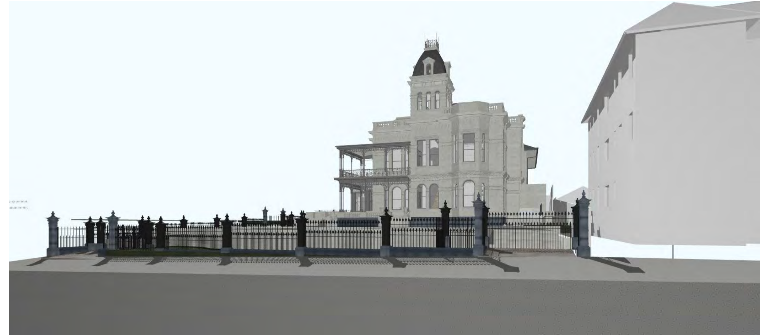
VIEW FROM TOORAK RD LOOKING NORTH ROOF TERRACE NOT VISIBLE
