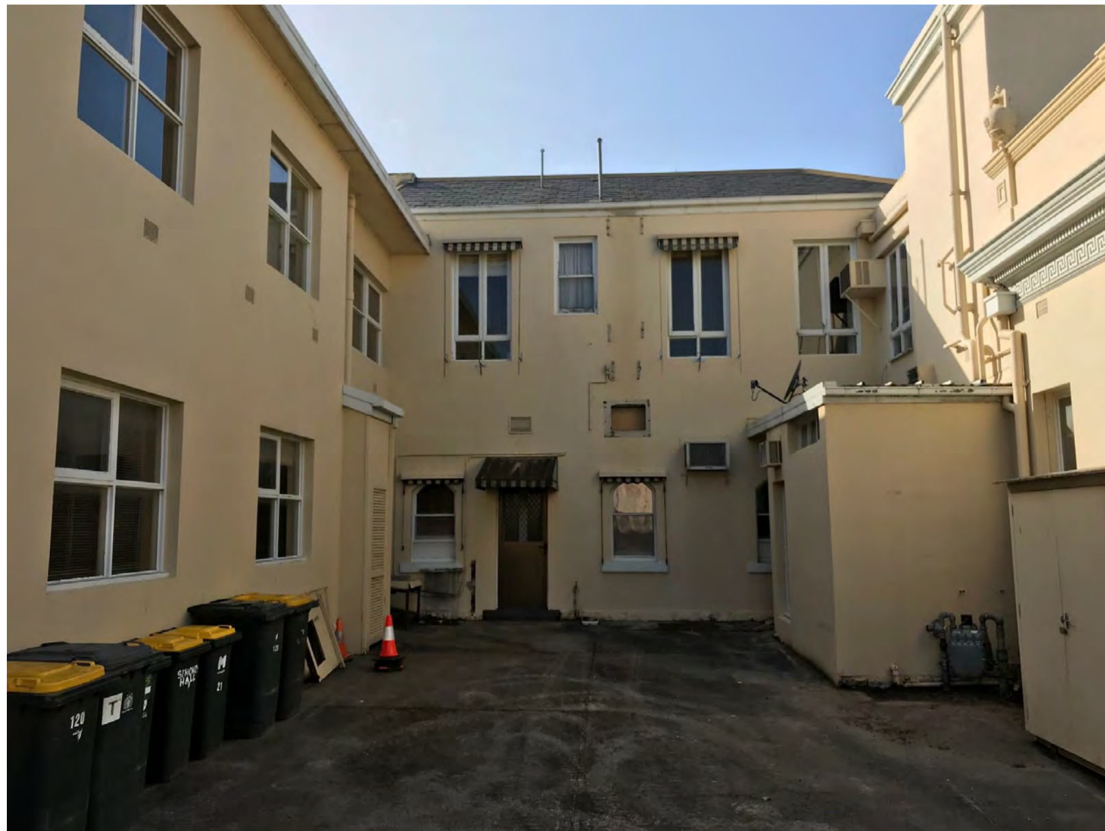
SUBJECT SITE - WEST ELEVATION
