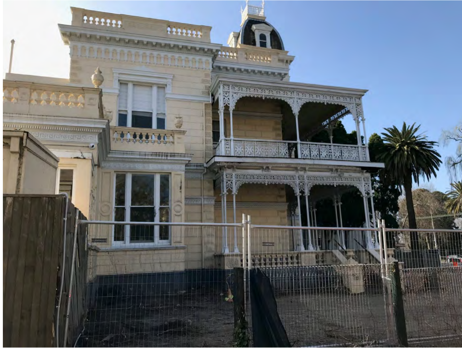
SUBJECT SITE - WEST ELEVATION
