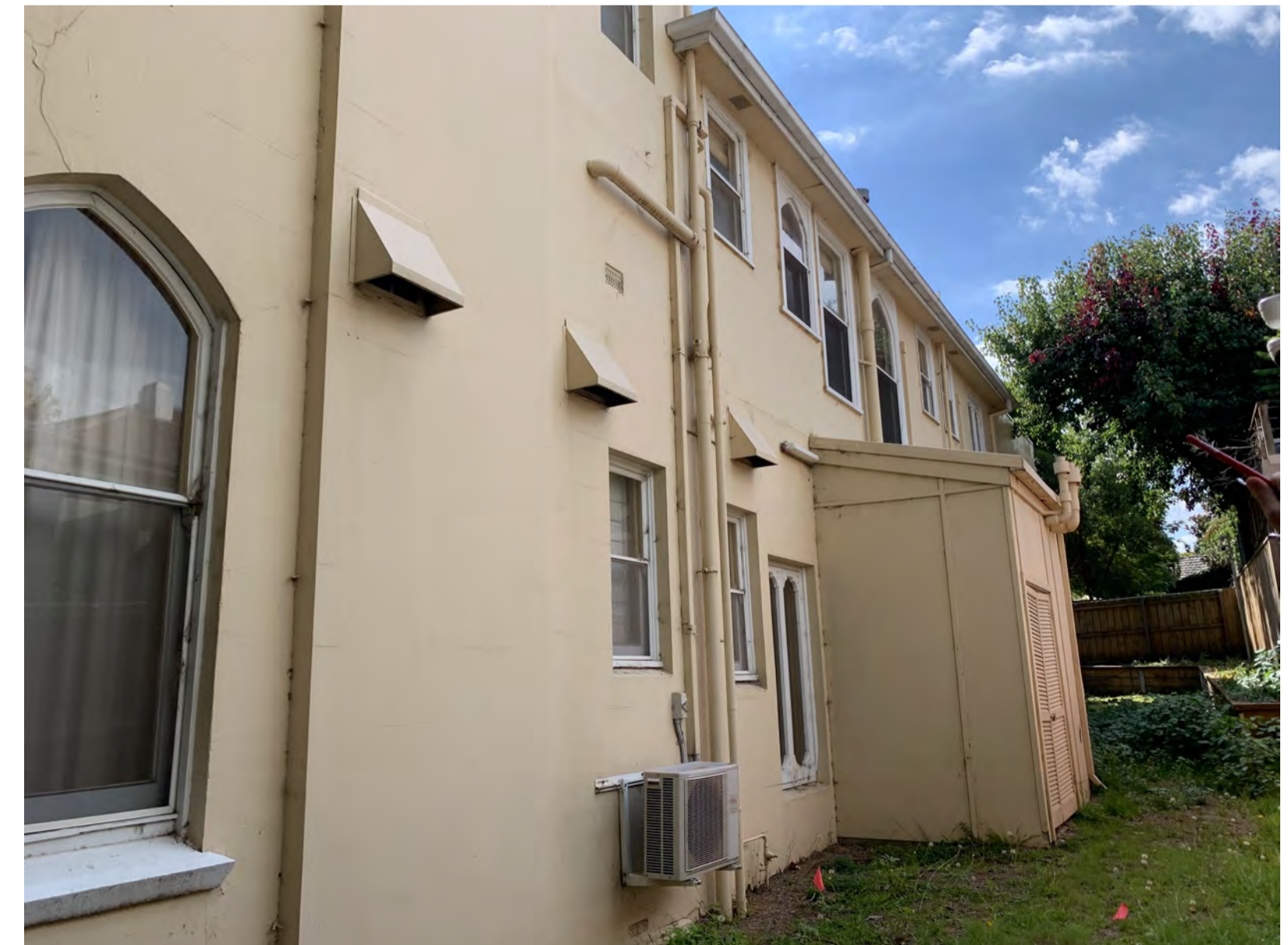
SUBJECT SITE - EAST ELEVATION
