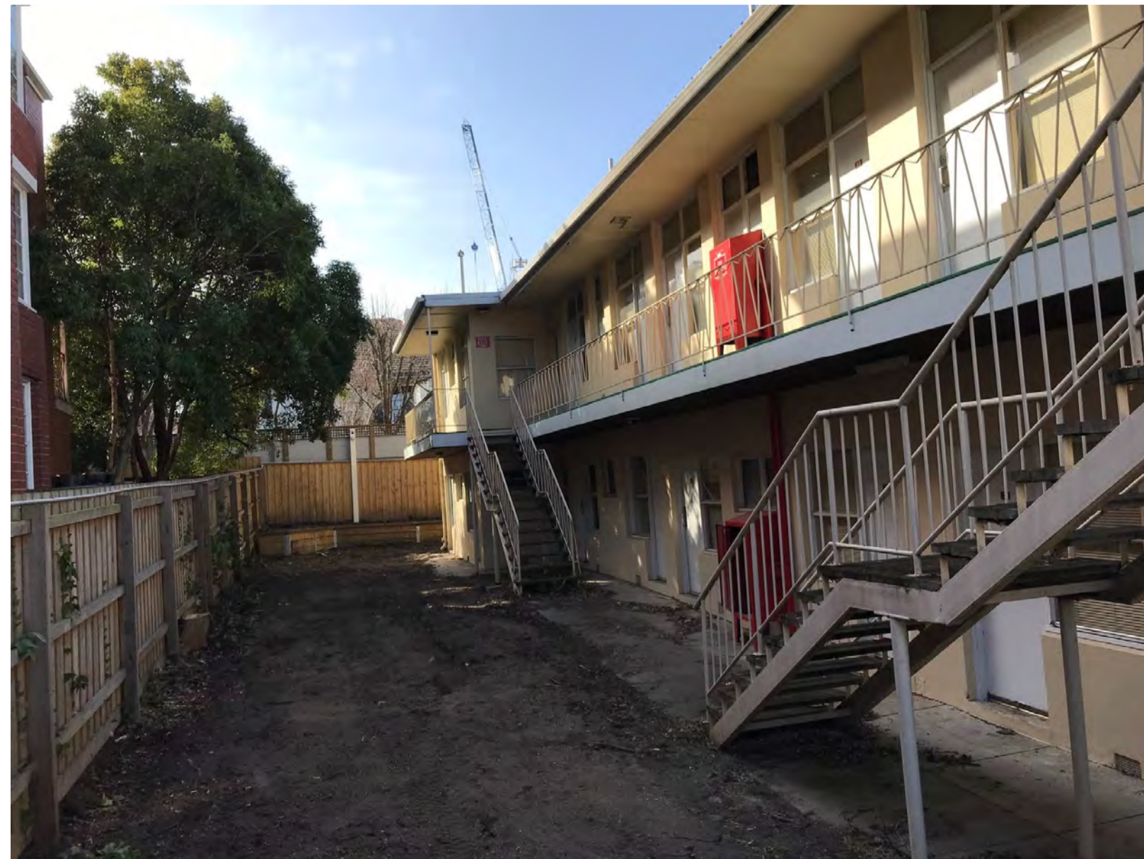
SUBJECT SITE - NORTH ELEVATION
