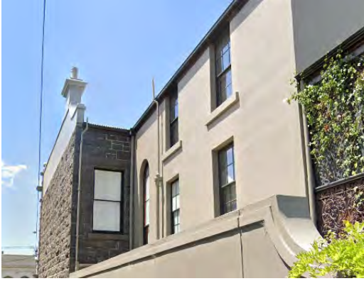
Figure 31 – extract of the north facing windows at 91 Powlett St (Source: Google, image taken November 2018)
