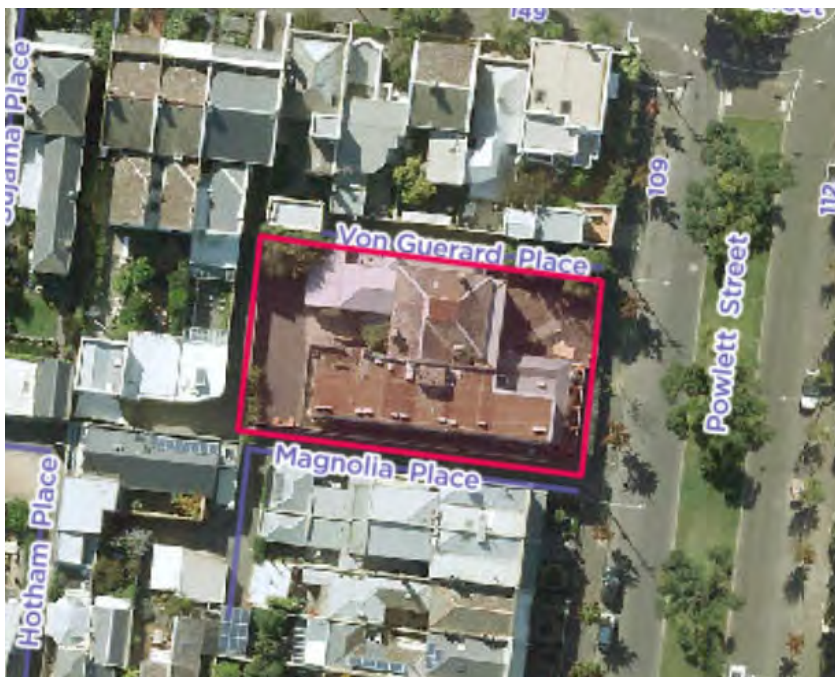
Figure 1 – aerial image of the Site (Source: CoMPass, image taken 4 April 2021)
