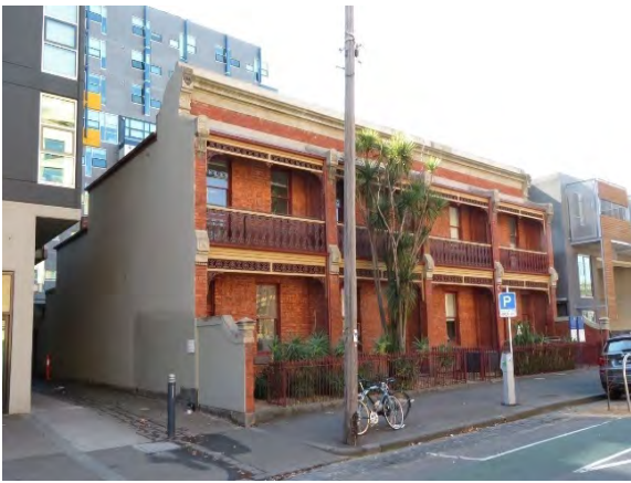
Figure 15 Royal Terrace, 272-278 Faraday Street, Carlton (HO56) Source: Lovell Chen
