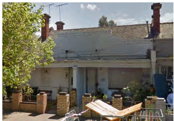
Figure 19 323-234 Faraday Street, Carlton (HO1) Source: Streetview
