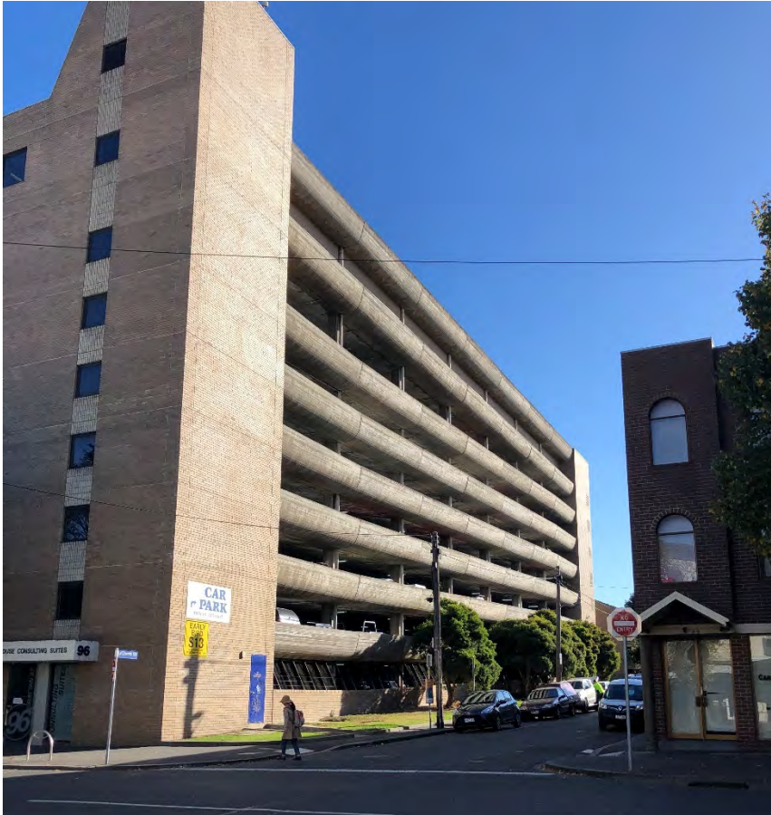
Figure 11 Rear (east) elevation of carpark Source: Lovell Chen
