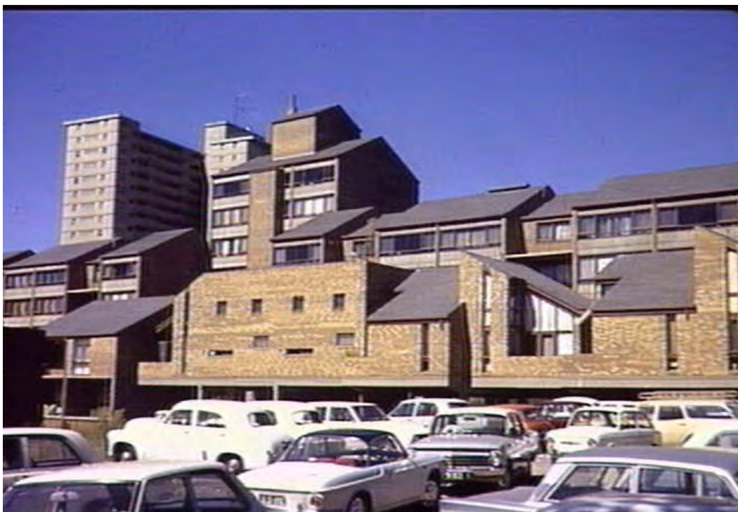
Figure 9 Completed Cross Street Co-operative Development, Lot 1, 1970 Source: Peter Wille, H91.244/1839, State Library of Victoria Picture Collection
