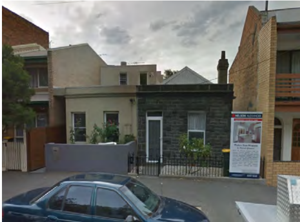
Figure 11 46 Palmerston Street, Carlton (HO1) Source: Streetview
