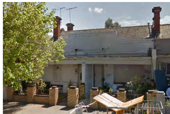
Figure 20 323-234 Faraday Street, Carlton (HO1) Source: Streetview
