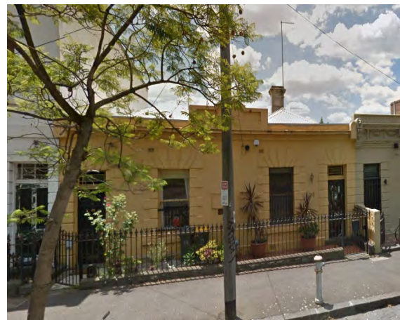
Figure 13 26-8 Barkly Street, Carlton (HO1) Source: Streetview
