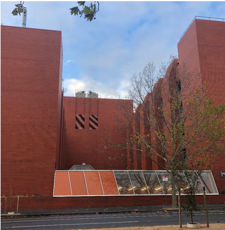
Figure 12 At right is the south elevation of Building 56; the glazed roof/atrium at centre image is over the basement level which connects Buildings 56 and 57; the north end of Building 57 is at left Source: Lovell Chen
