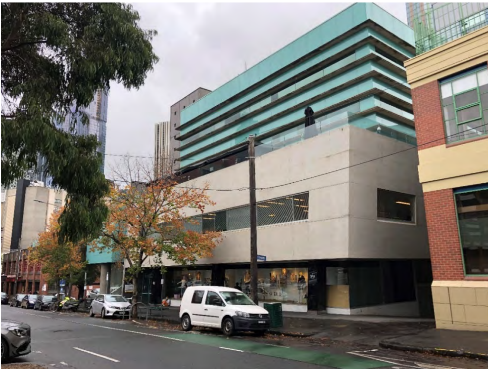
Figure 9 Subject building, viewed from the north; the projecting northern bay at centre is clad in off-white mosaic tiles, with the large volume above clad in blue-green coloured glass Source: Lovell Chen
