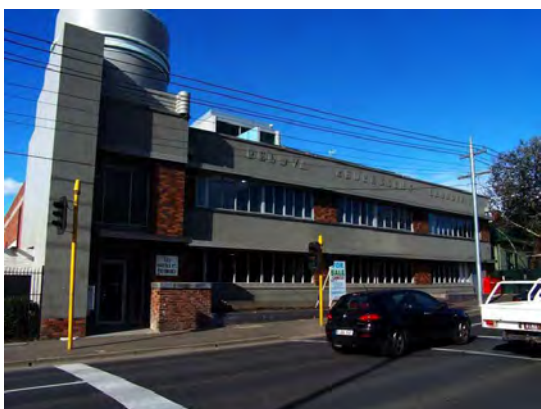
Figure 10 129 Hoddle Street, Richmond (HO391) Source: Victorian Heritage Database
