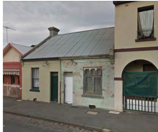
Figure 11 126 Station Street, Carlton (HO1) Source: Streetview
