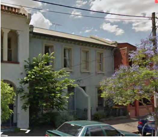
Figure 15 38 Carlton Street, Carlton (HO1) Source: Streetview
