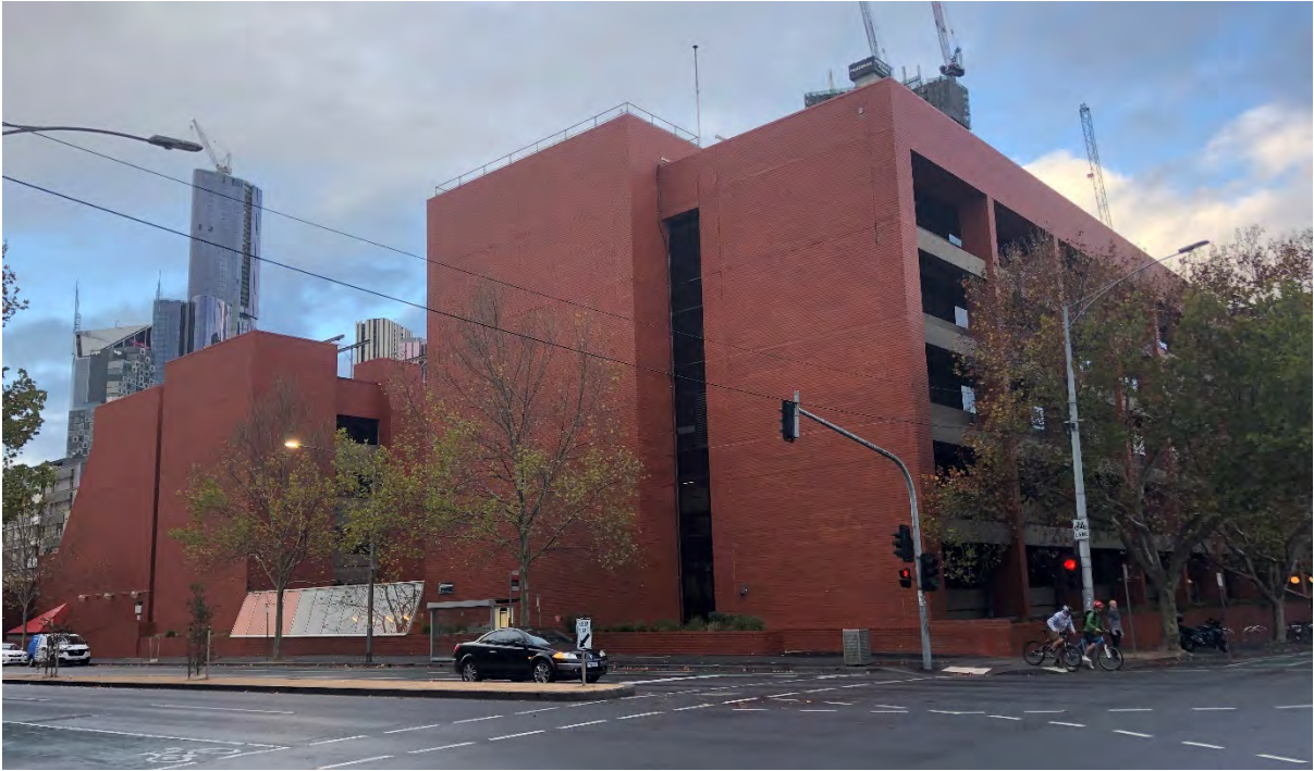
Figure 9 Building 56, east elevation to Lygon Street, with the east elevation of Building 57 at left Source: Lovell Chen
