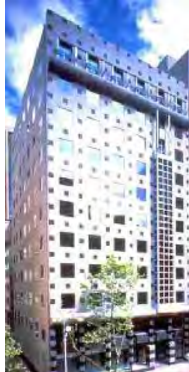
Figure 13 91-97 William Street, Melbourne (1987) Source: http://www.walkingmelbourne.com/building443.html
