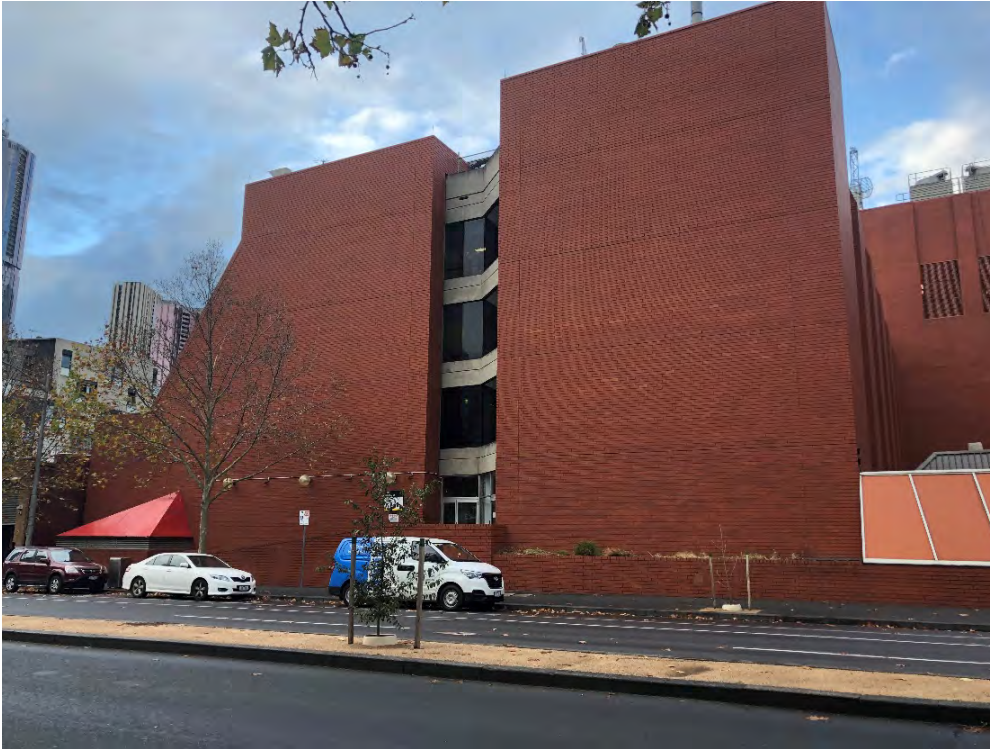
Figure 13 Building 57, east elevation; note entrance in recessed centre bay and the angled profile at the south end (left of image) Source: Lovell Chen
