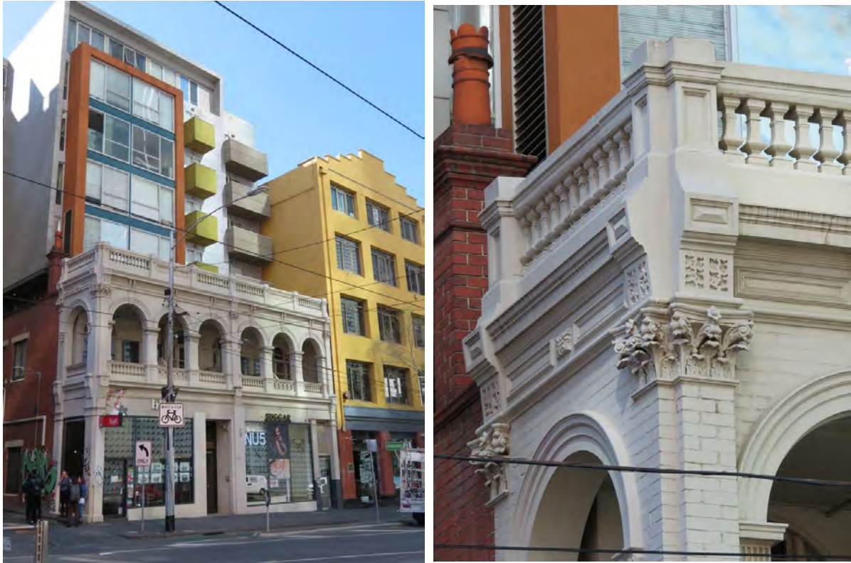
Figure 10 466 Swanston Street (at left), decorative detail to upper façade and return parapet at north corner of the building (at right)
