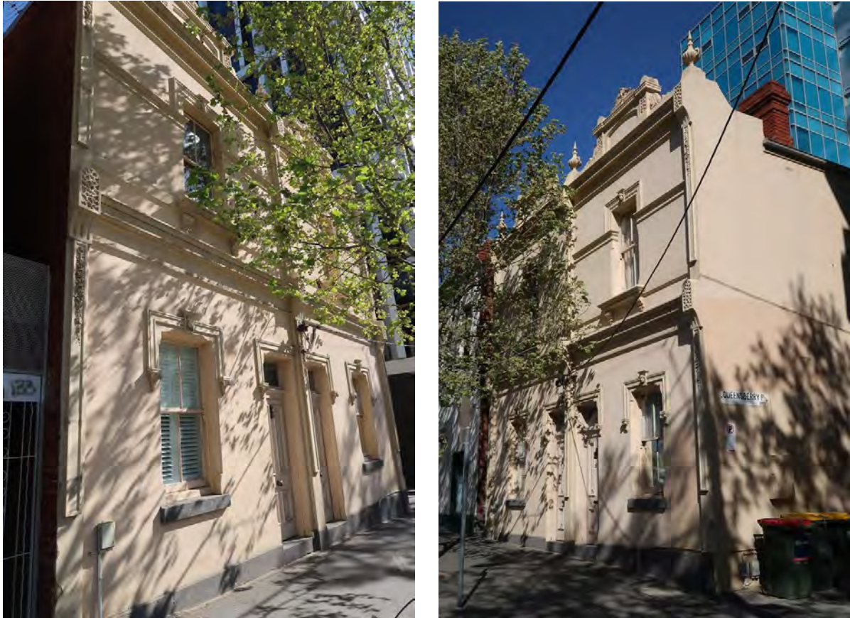
Figure 7 133-5 Queensberry Street from the north- east (at left) 133-5 Queensberry Street from the north-west (at right) Source: Lovell Chen
