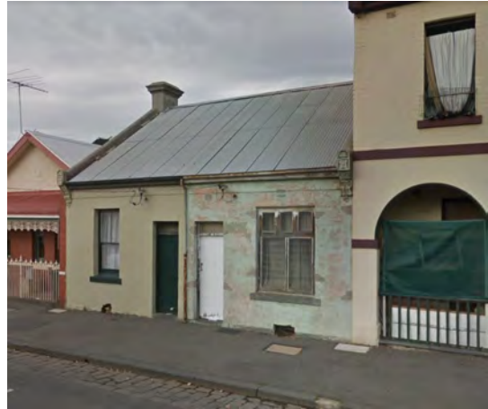
Figure 12 126 Station street, Carlton (HO1) Source: Streetview
