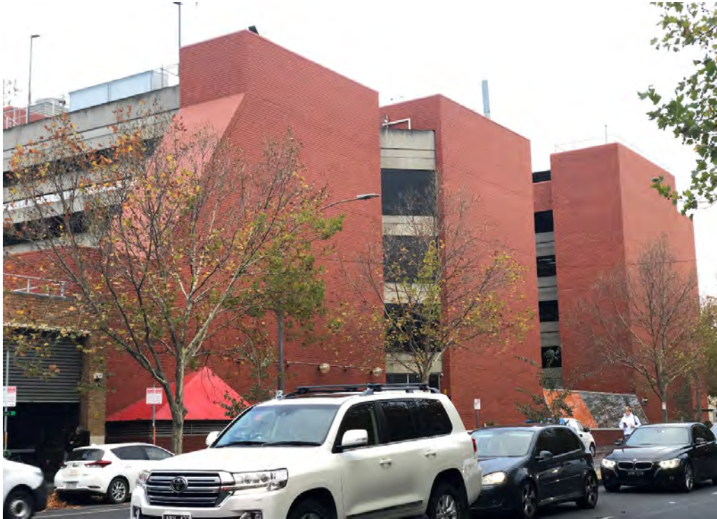
Figure 15 Buildings 57 and 56, as seen from the south on Lygon Street; note the tiered form of the south elevation of Building 57 (at left) Source: Lovell Chen
