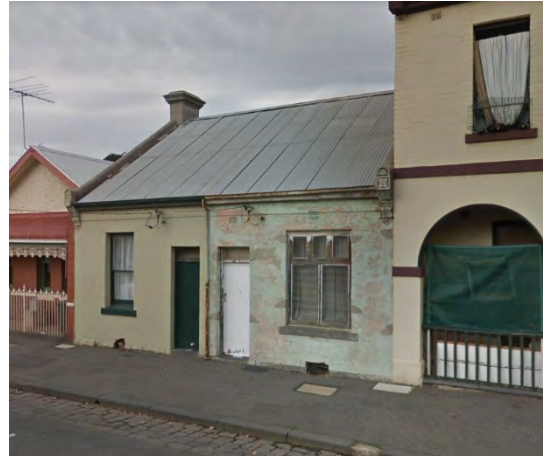
Figure 10 126-8 Station street, Carlton (HO1) Source: Streetview
