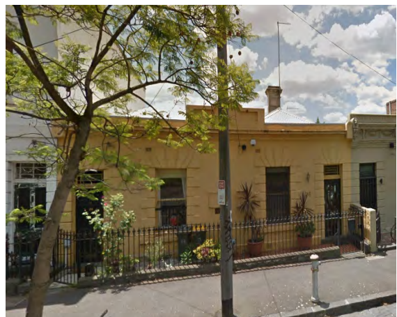
Figure 14 26-8 Barkly Street, Carlton (HO1) Source: Streetview
