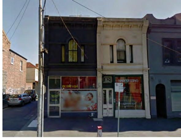
Figure 12 82-84 Elgin Street, Carlton (HO1) Source: Google Streetview
