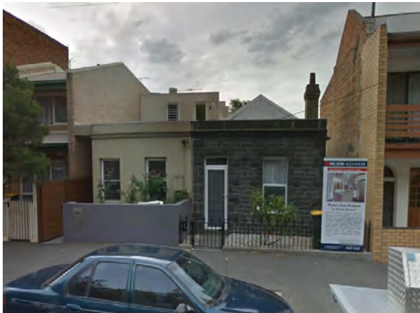
Figure 10 46 Palmerston Street, Carlton (HO1) Source: Streetview
