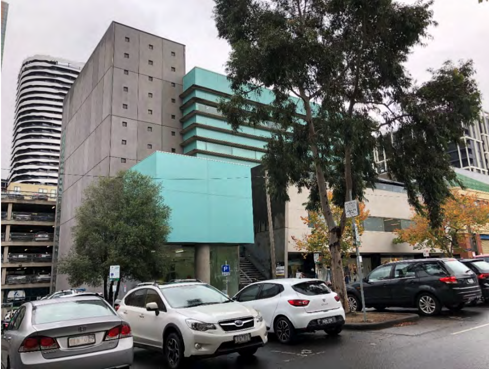
Figure 10 Subject building, viewed from the south; the grey concrete service block is at left, fronted by the southern bay clad in blue-green mosaic tiles Source: Lovell Chen
