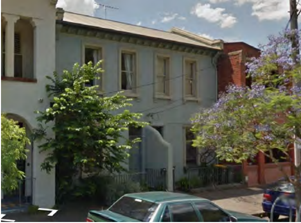
Figure 14 38 Carlton Street, Carlton (HO1) Source: Streetview
