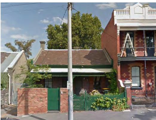
Figure 17 131 Barkly Street, Carlton (HO1) Source: Streetview
