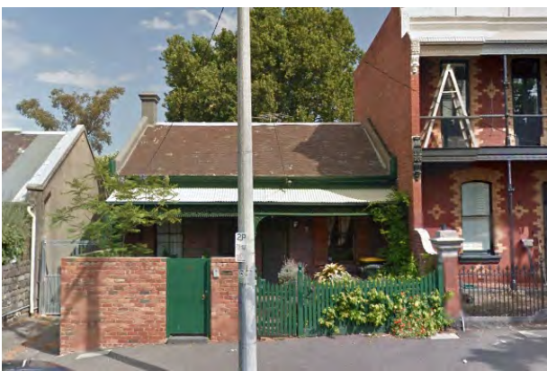
Figure 18 131 Barkly Street, Carlton (HO1) Source: Streetview
