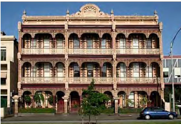
Figure 9 Holcombe Terrace, Carlton (HO1) Source: Victorian Heritage Database
