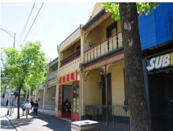
Figure 23 676-82 Swanston Street, Carlton (HO116) Source: Lovell Chen
