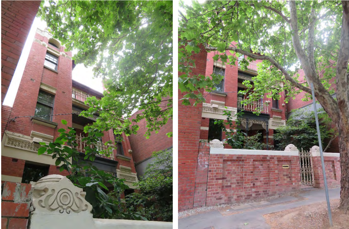
Figure 8 25-7 Rathdowne Street, Carlton; note the central recessed verandah rising up through the building levels
