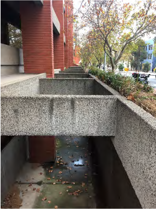
Figure 11 Building 56, north side, detail of lightwell to basement level below Source: Lovell Chen
