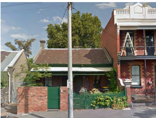
Figure 19 131 Barkly Street, Carlton (HO1) Source: Streetview
