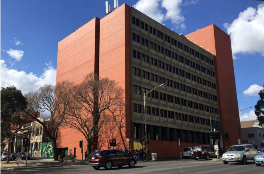
Figure 5 Building 51 as viewed from the corner of Victoria and Cardigan streets; the concrete façade faces south, with the service tower and stepped entry at the east end (right of image); the brick elevation at left faces west Source: Lovell Chen
