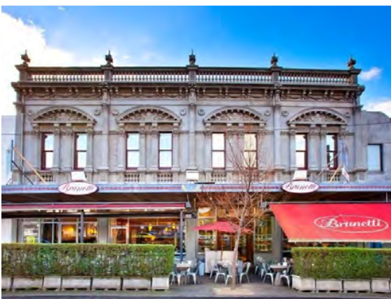
Figure 11 Shops at 198-204 Faraday Street, Carlton, Norman Hitchcock architect, 1886 (HO1) Source: Pinterest
