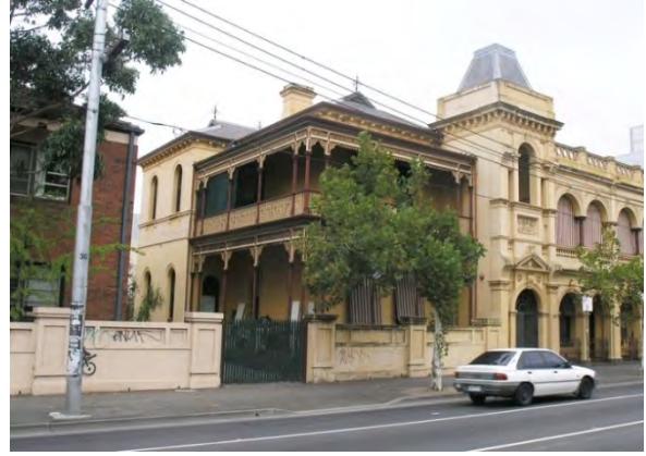
Figure 8 Urbrae, 171 Hoodle Street, Richmond (VHR H0719 and HO267), Source: Victorian Heritage Database
