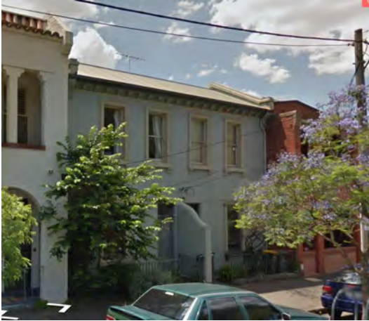
Figure 13 38 Carlton Street, Carlton (HO1) Source: Streetview
