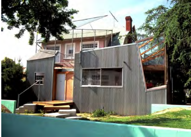
Figure 17 Santa Monica House, Frank Gehry
