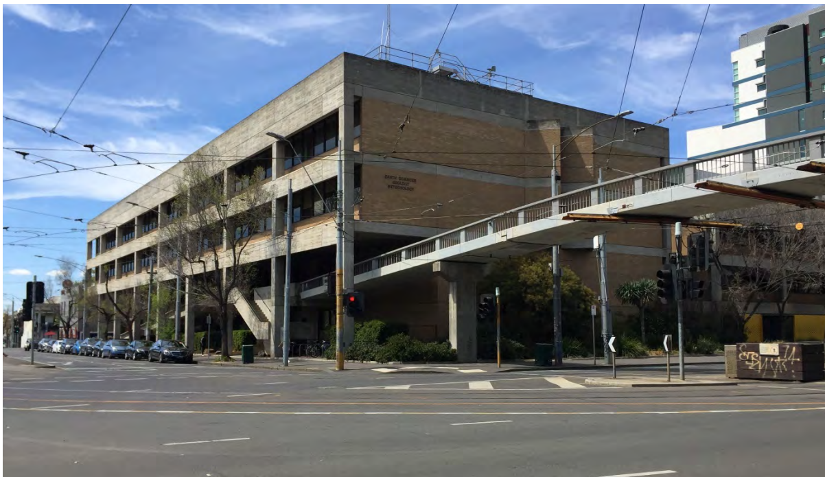
Figure 9 View from the intersection of Elgin and Swanston streets, with footbridge at right Source: Lovell Chen
