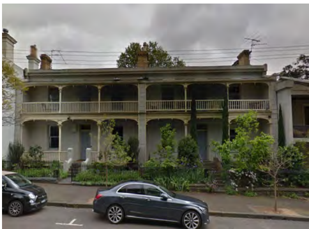
Figure 13 82-4 Carlton Street, Carlton (HO1) Source: Streetview
