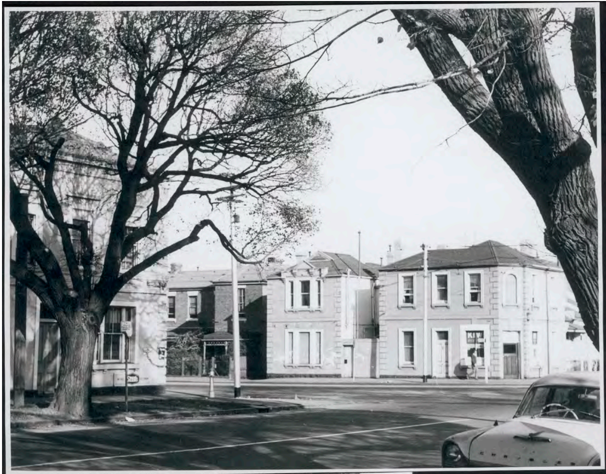
Figure 2 The subject site c. 1956-68, before construction of the Earth Sciences Building Source: State Library of Victoria
