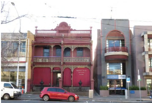
Figure 23 454-6 Swanston Street, Carlton (HO113) Source: Lovell Chen
