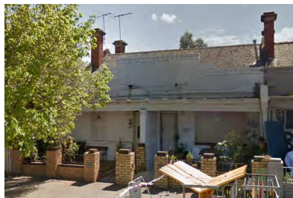
Figure 18 323-234 Faraday Street, Carlton (HO1) Source: Streetview
