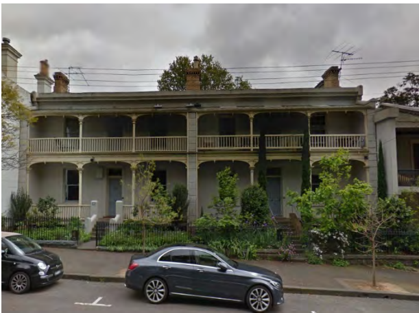
Figure 11 82-4 Carlton Street, Carlton (HO1) Source: Streetview
