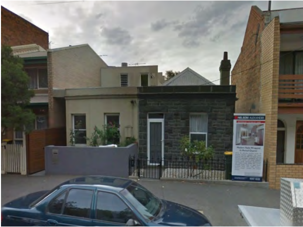
Figure 9 46 Palmerston Street, Carlton (HO1) Source: Streetview
