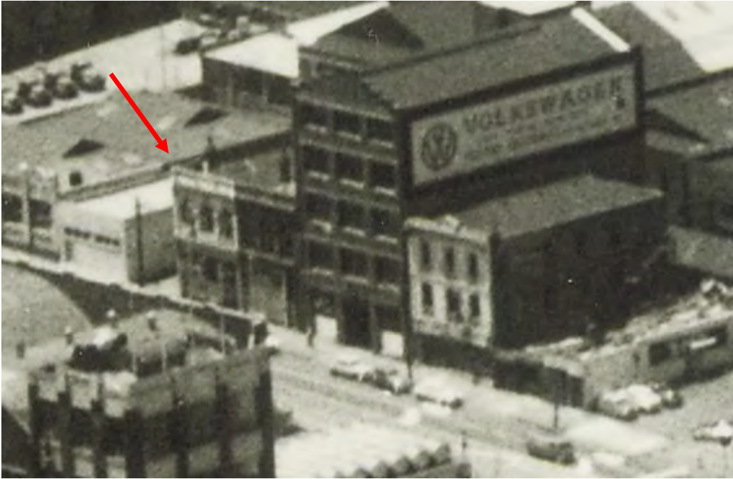
Figure 6 1960 oblique aerial photograph with subject building indicated Source: Commercial Photographic Co., H2009.95/37, Harold Paynting Collection, State Library of Victoria
