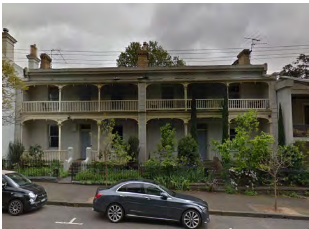
Figure 12 82-4 Carlton Street, Carlton (HO1) Source: Streetview
