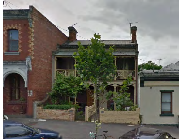
Figure 16 134-6 Barkly Street, Carlton (HO1) Source: Streetview
