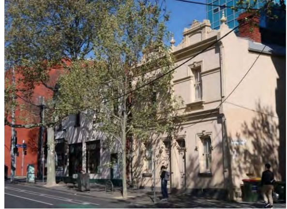
Figure 20 133-5 Queensberry Street (HO36) Source: Lovell Chen
