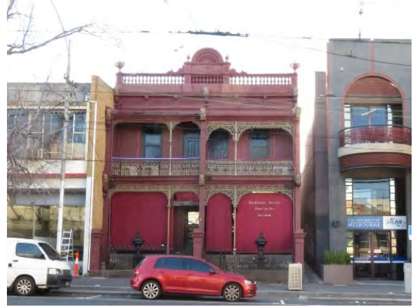
Figure 21 454-6 Swanston Street, Carlton (HO36) Source: Lovell Chen
