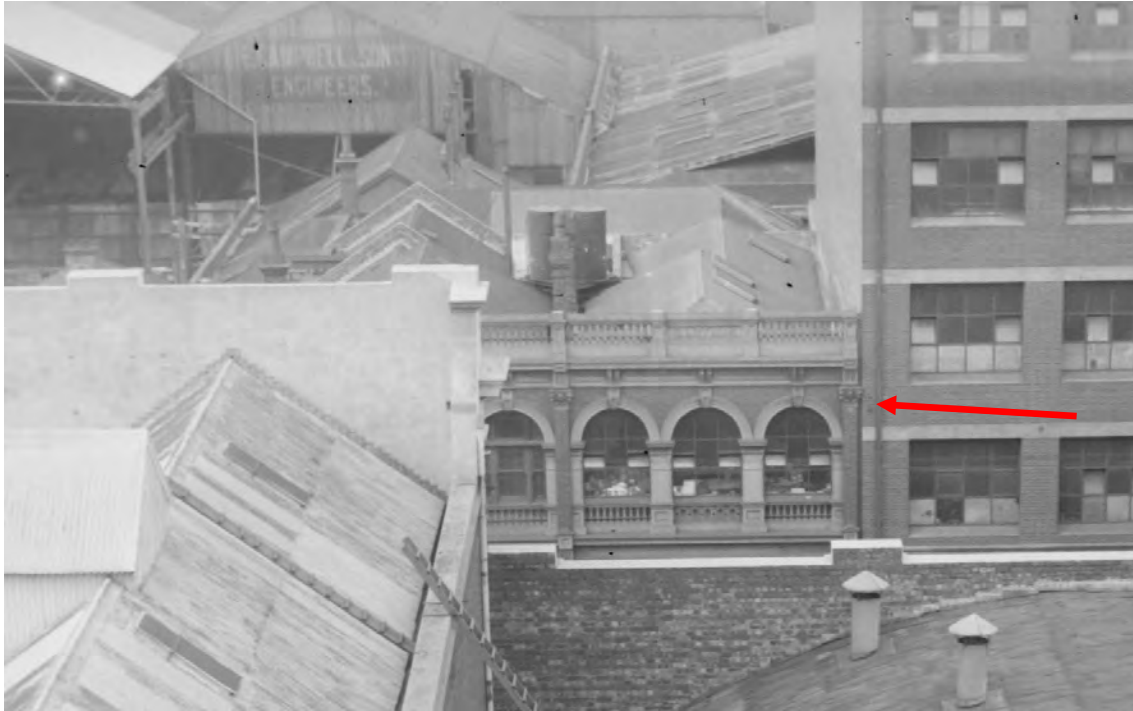
Figure 4 View across Carlton Brewery, c. 1920s, with top level of subject building visible Source: Walter Vears Collection, H99.149/65, State Library of Victoria
