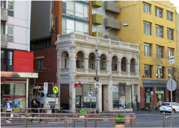
Figure 22 466 Swanston Street, Carlton (HO113) Source: Lovell Chen
