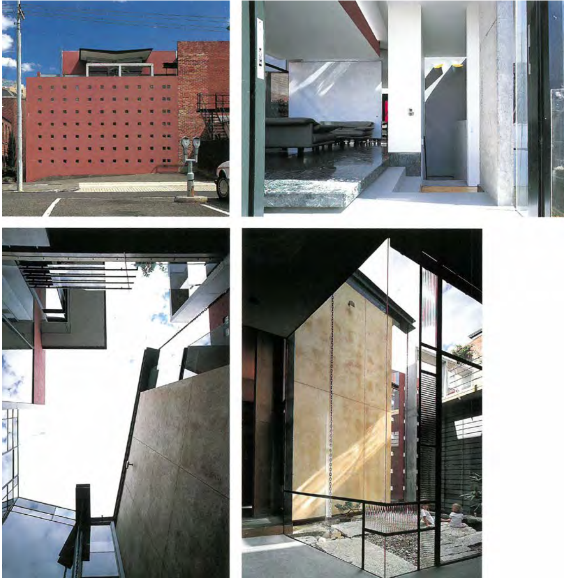
Figure 6 Photographs by Scott Frances of the extension at the rear of 64-68 Drummond Street. The top images depict the addition's north elevation and living room and the bottom images, the internal courtyard
