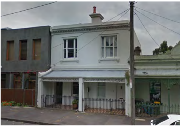
Figure 16 36 Macarthur Place North, Carlton (HO1) Source: Streetview
