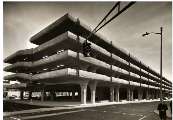
Figure 15 Temple Street Parking Garage, New Haven, US Source: Shorpy.com
