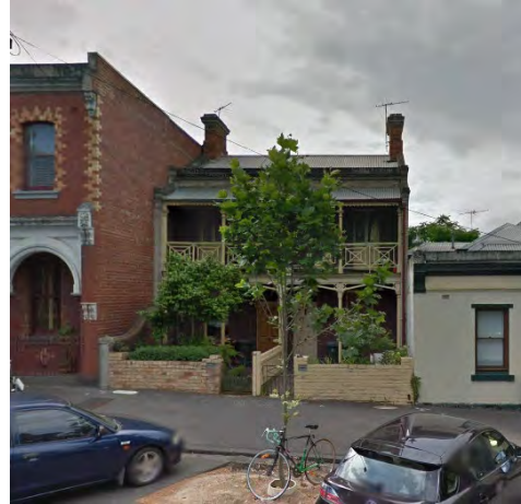
Figure 14 134-6 Barkly Street, Carlton (HO1) Source: Streetview
