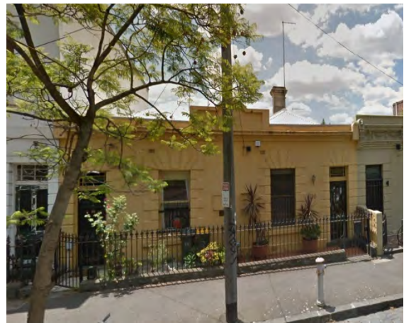
Figure 12 26-8 Barkly Street, Carlton (HO1) Source: Streetview
