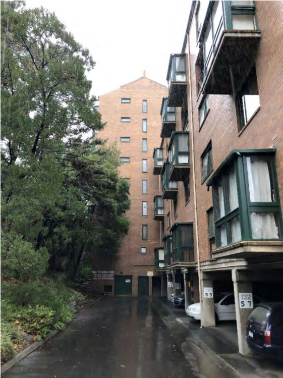
Figure 13 View from Lygon Street, with the taller tower building in the distance, and the rear of other flat blocks at right Source: Lovell Chen
