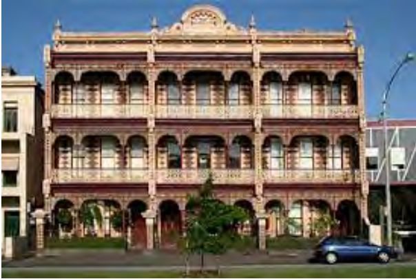
Figure 25 Holcombe Terrace, 201-5 Drummond Street, Carlton (HO1) Source: Victorian Heritage Database
