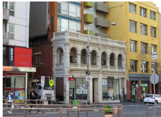
Figure 22 466 Swanston Street, Carlton (HO111) Source: Lovell Chen
