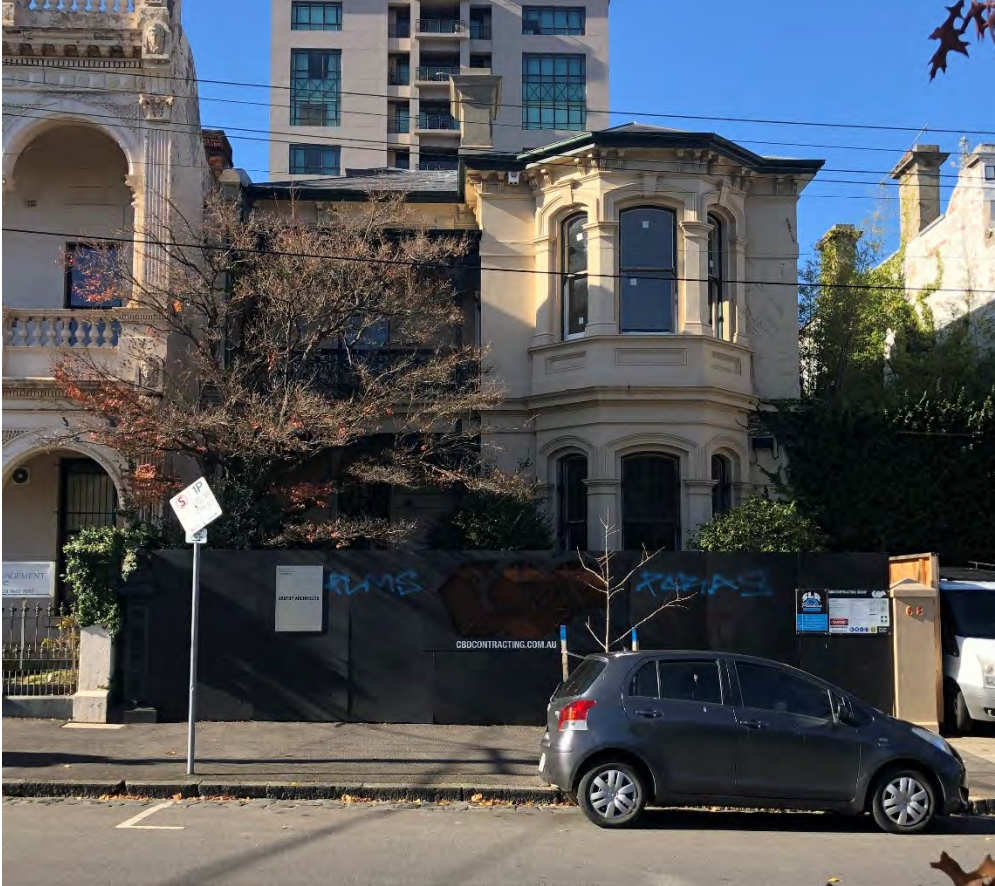
Figure 5 Victorian villa, 64-68 Drummond Street, Carlton
