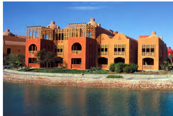
Figure 15 Steigenberger Golf Resort, Egypt, (1993-5) Source: https://www.michaelgraves.com/proj
