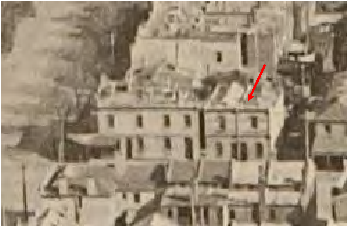
Figure 5 Oblique aerial photograph of 1927, with the subject pair at 133-135 Queensberry Street, Carlton indicated Source: Airspy collection, H2501, State Library of Victoria
