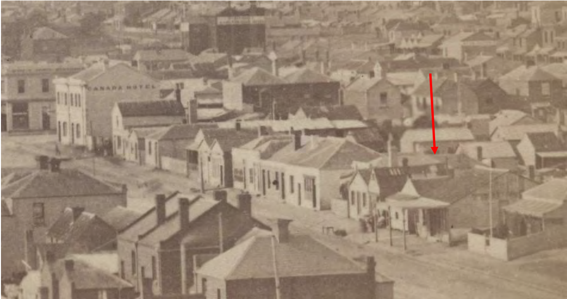
Figure 2 View from Carlton Brewery of east side of Swanston Street between Queensberry and Pelham streets, Carlton, 1870. Approximate location of subject site indicated (prior to construction of the current buildings)
