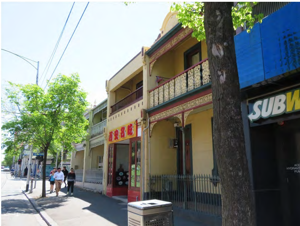
Figure 7 676-682 Swanston Street, Carlton
