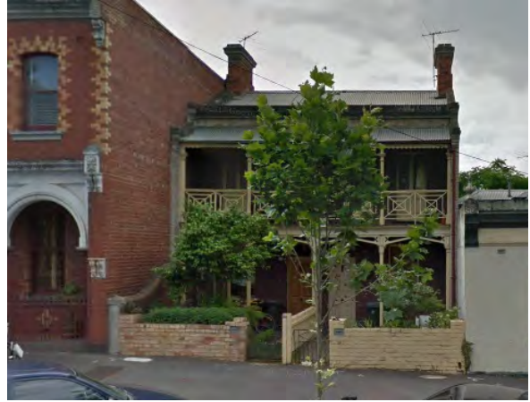
Figure 15 134-6 Barkly Street, Carlton (HO1) Source: Streetview
