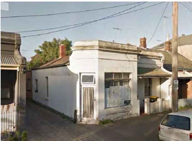
Figure 11 76 Palmerston Street, Carlton (HO1) Source: Google Streetview
