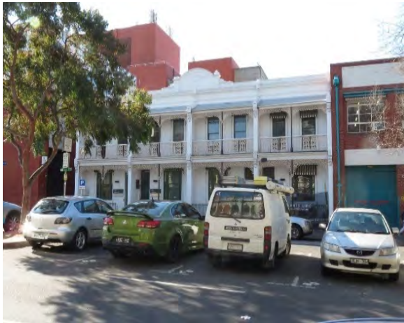
Figure 14 Mary's Terrace, 50-6 Cardigan Street, Carlton (HO36) Source: Lovell Chen
