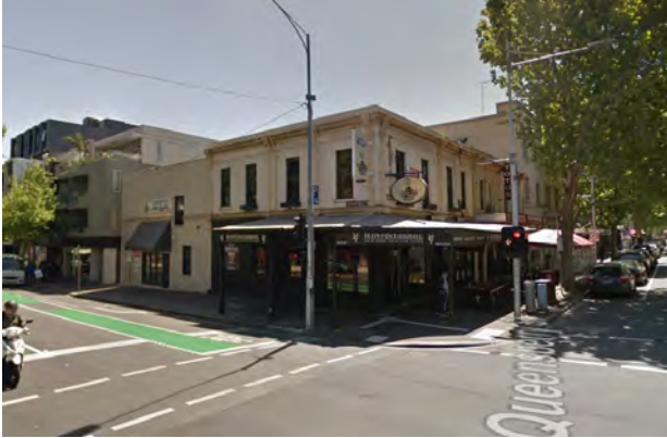
Figure 9 86-92 Queensberry Street, Carlton (HO1) Source: Google Streetview
