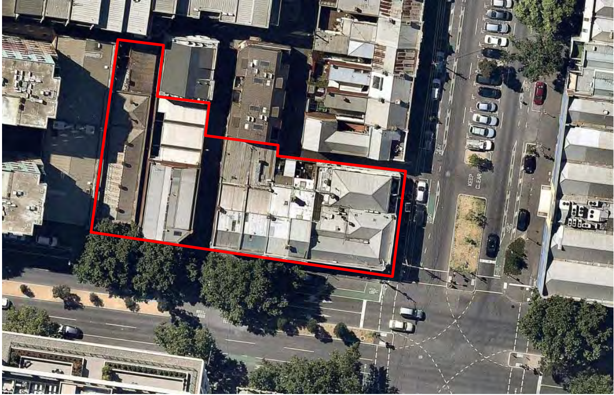
Figure 11 Recent aerial photograph of the intersection of Queensberry Street and Cardigan Street, with the proposed Hotel Lincoln and Environs Precinct indicated Source: Nearmap, February 2019
