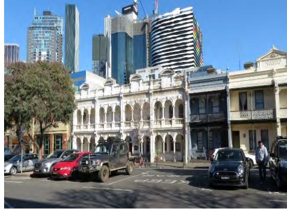
Figure 9 51-65 Cardigan Street, Carlton (HO27) Source: Lovell Chen
