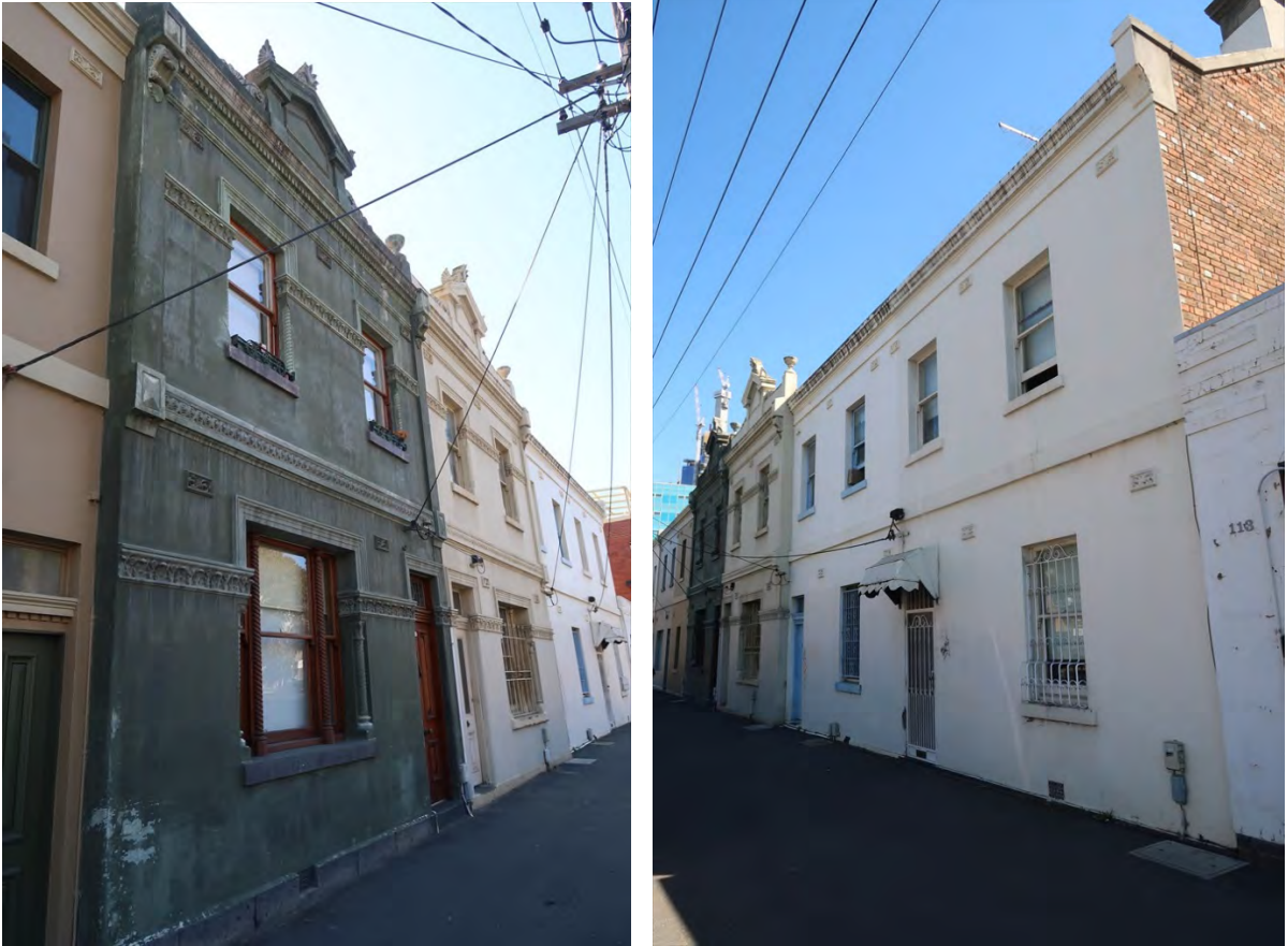
Figure 7 Remodelled facades at nos 105-107 Cardigan Street (at left); 101-111 Cardigan Street viewed from the north
