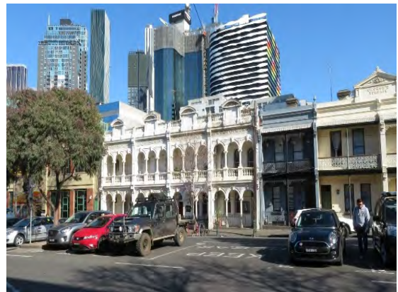
Figure 9 51-65 Cardigan Street, Carlton (HO27) Source: Lovell Chen
