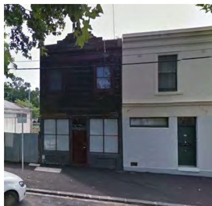
Figure 14 68 Barkly Street, Carlton (HO1) Source: Google Streetview
