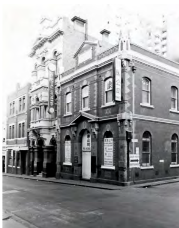
Figure 29 Church of England Mission Hall, 108-110 Little Bourke Street, Melbourne (1884, HO688 and HO507)
