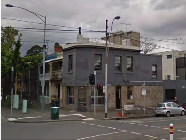
Figure 15 332 Cardigan Street, Carlton (HO1) Source: Google Streetview
