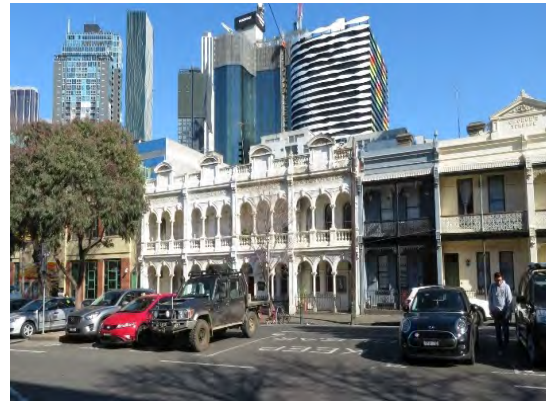
Figure 11 51-65 Cardigan Street, Carlton (HO27) Source: Lovell Chen
