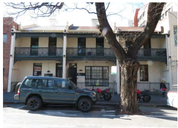
Figure 13 18-22 Cardigan Street, Carlton (HO35) Source: Lovell Chen
