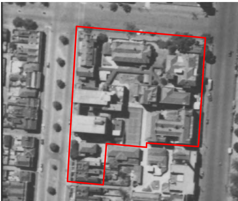
Figure 5 1945 aerial image of the subject site; this illustrates several buildings which were later replaced by modern development, including to the corner of Rathdowne and Pelham streets, and on Drummond Street. Approximate boundaries of precinct indicated
