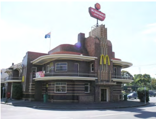
Figure 23 Former United Kingdom Hotel, Clifton Hill (VHR H0684 and HO92 – City of Yarra) Source: Victorian Heritage Database
