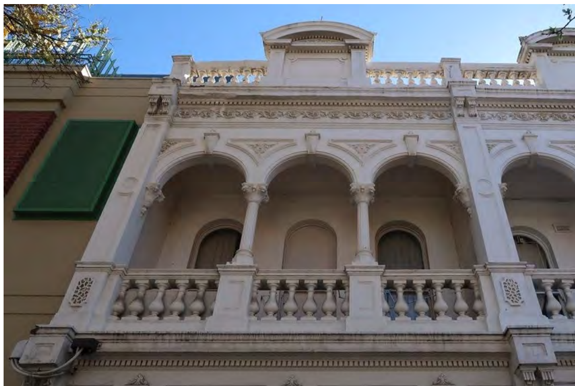
Figure 6 Upper façade, 51 Cardigan Street, Carlton
