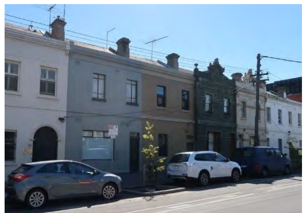
Figure 11 101-111 Cardigan Street, Carlton (H030) Source: Lovell Chen
