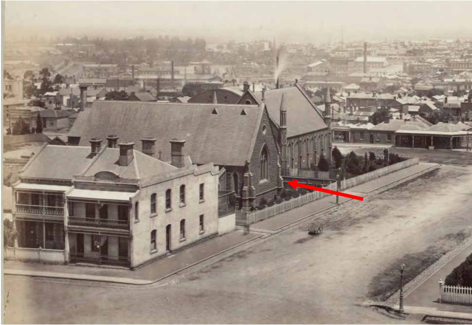
Figure 3 View of Queensberry Street from Gaelic Church, 1875, with the Catholic Apostolic Church indicated, and the Primitive Methodist Church of 1864 to its right; note the timber picket fence to the boundary
