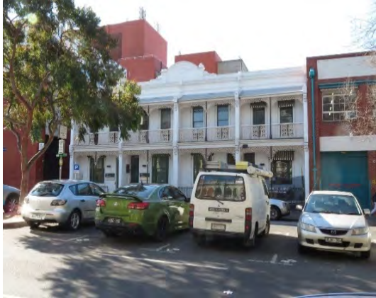
Figure 14 Mary's Terrace, 50-6 Cardigan Street, Carlton (HO36) Source: Victorian Heritage Database
