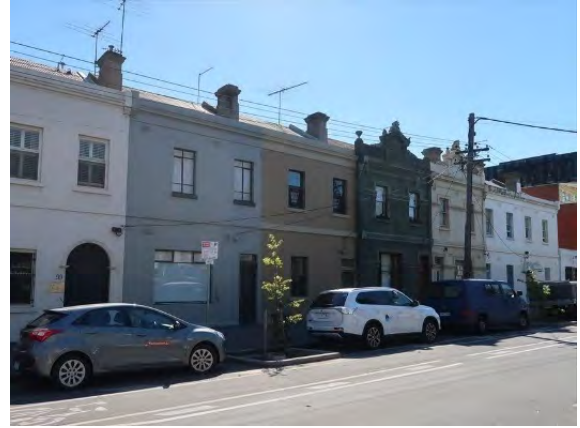
Figure 13 101-111 Cardigan Street, Carlton (HO30) Source: Lovell Chen
