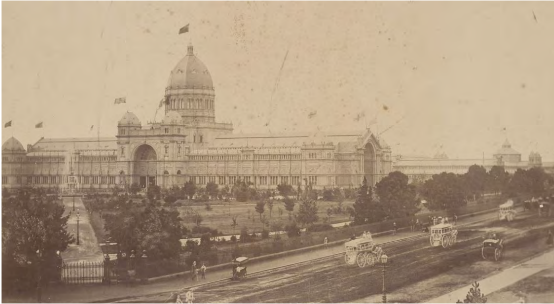
Figure 3 View of Royal Exhibition Building from Nicholson Street, with Carlton Gardens in foreground, c. 1890
