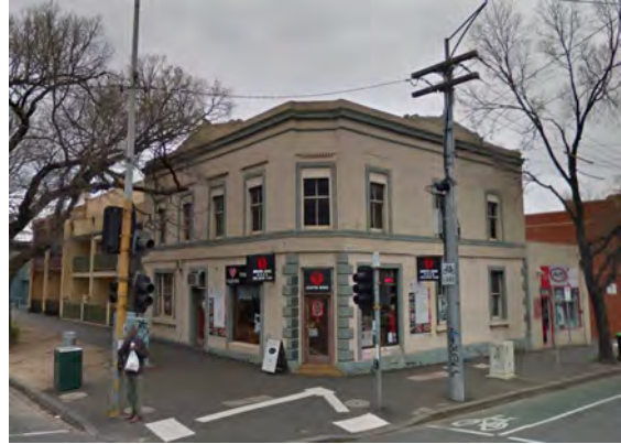
Figure 10 832 Swanston Street, Carlton (HO1) Source: Google Streetview
