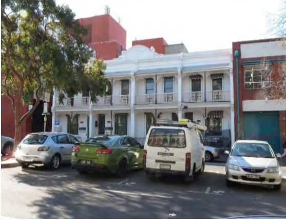
Figure 12 Mary's Terrace, 50-6 Cardigan Street, Carlton (HO36) Source: Lovell Chen
