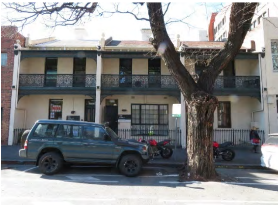
Figure 14 18-22 Cardigan Street Source: Lovell Chen
