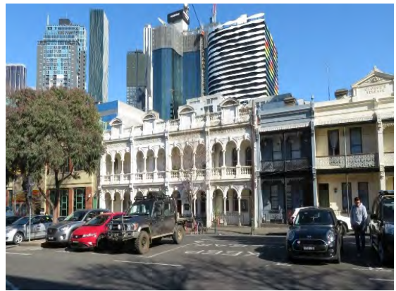
Figure 9 51-65 Cardigan Street, Carlton (HO27) Source: Lovell Chen
