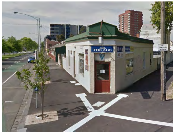
Figure 12 30 Canning Street, Carlton (HO1) Source: Google Streetview
