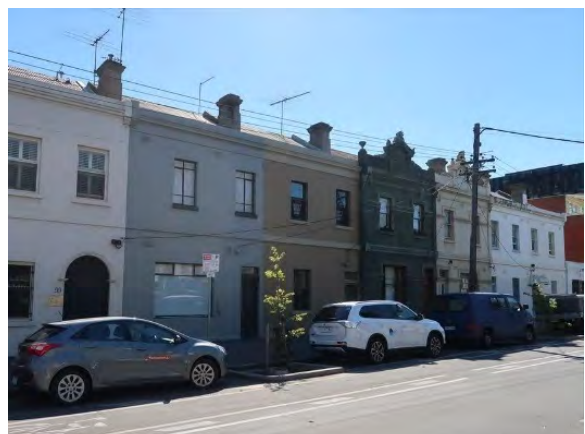
Figure 11 101-111 Cardigan Street, Carlton (HO30) Source: Lovell Chen
