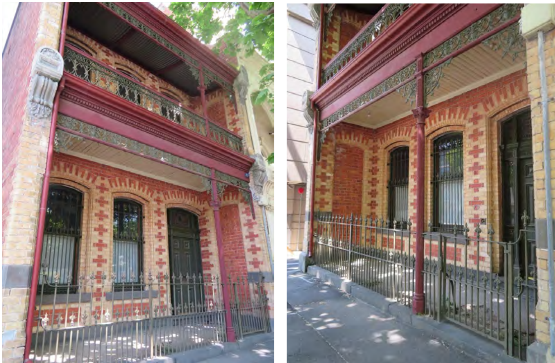
Figure 8 19 Queensberry Street facade (at left); ground floor verandah (at right)
