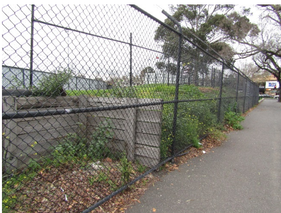
Figure 24. Cyclone fencing, mounding along the Brunton Avenue boundary. (Source: Context 2021)
