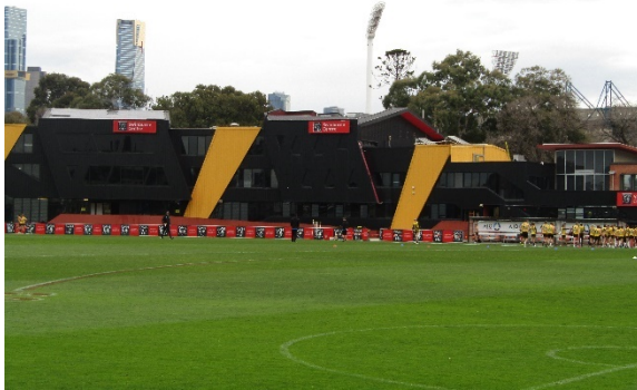
Figure 16. 2011 David Mandie Building (south elevation) facing the ground. (Source: Context 2021)
