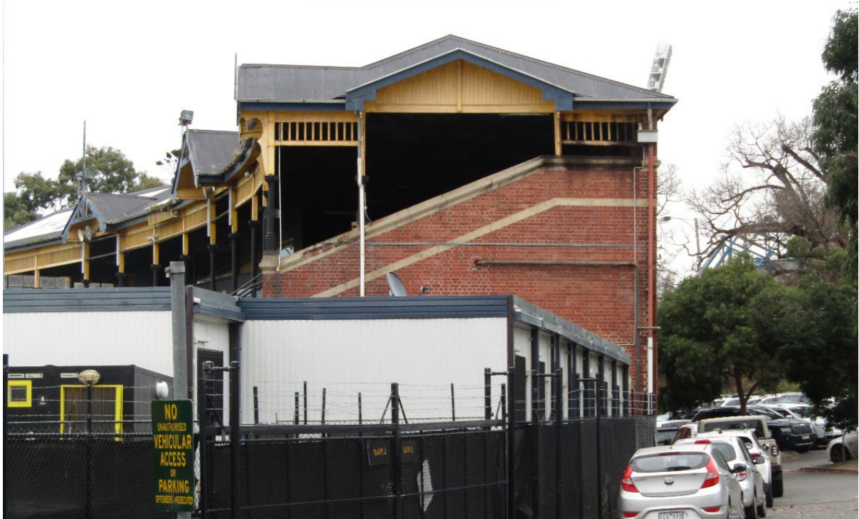
Figure 15. East elevation of the Jack Dyer Stand, and decorative detailing to east and south elevations. (Source: Context 2021)
