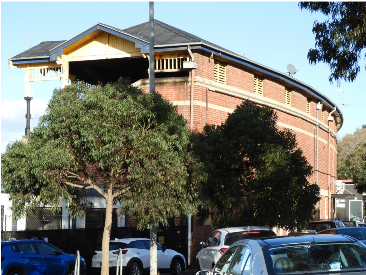
Figure 14. East and the curved north elevation of the Jack Dyer Stand. (Source: Context 2021)
