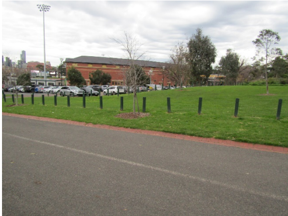
Figure 22. View to the rear of the Jack Dyer Stand approaching from Yarra Park (northeast). (Source: Context 2021)
