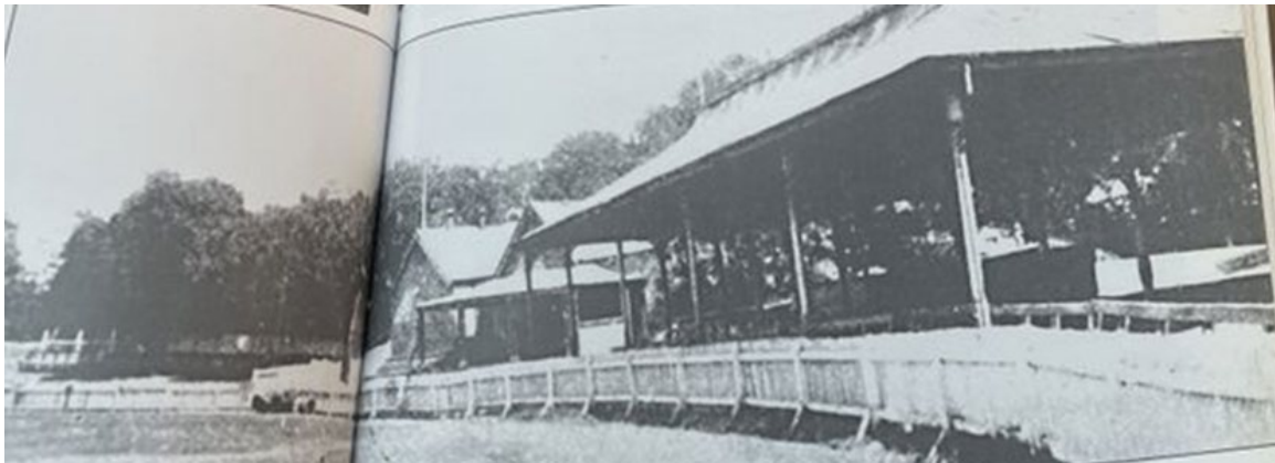
Figure 1. A former pavilion at the Melbourne Cricket Ground, photographed in 1915. (Source: Caruso 2002: 128–129)
