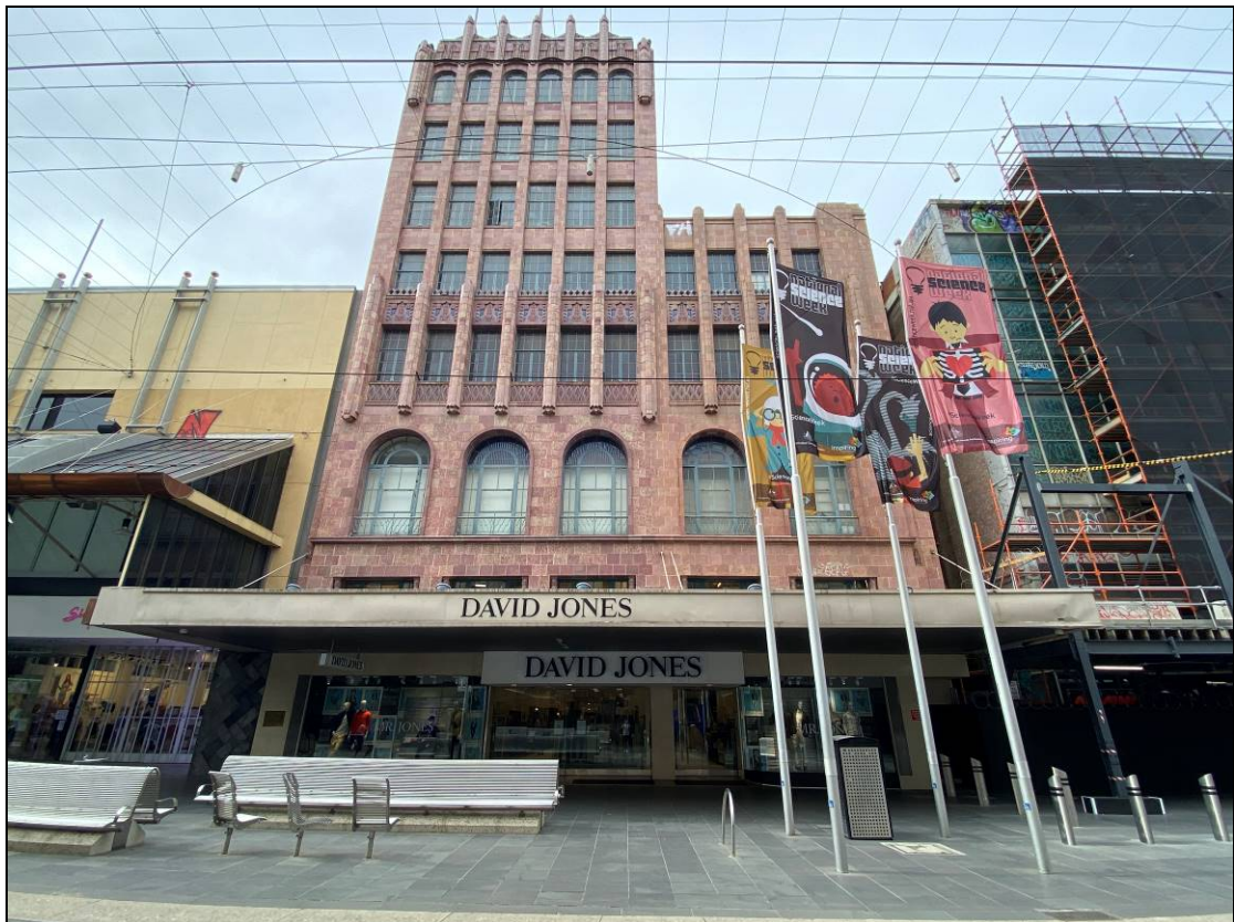
Figure 5: Bourke Street façade
