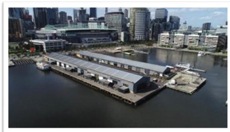
Figure 5: Photograph of Central Pier at Docklands
