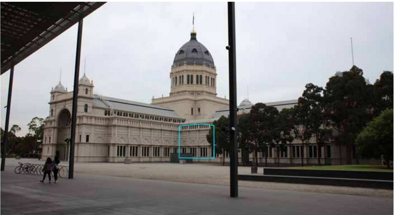
Testing of block form of proposed Vincent's Hospital proposal (outline). Note: the Vincent's Hospital proposal is fully obscured
