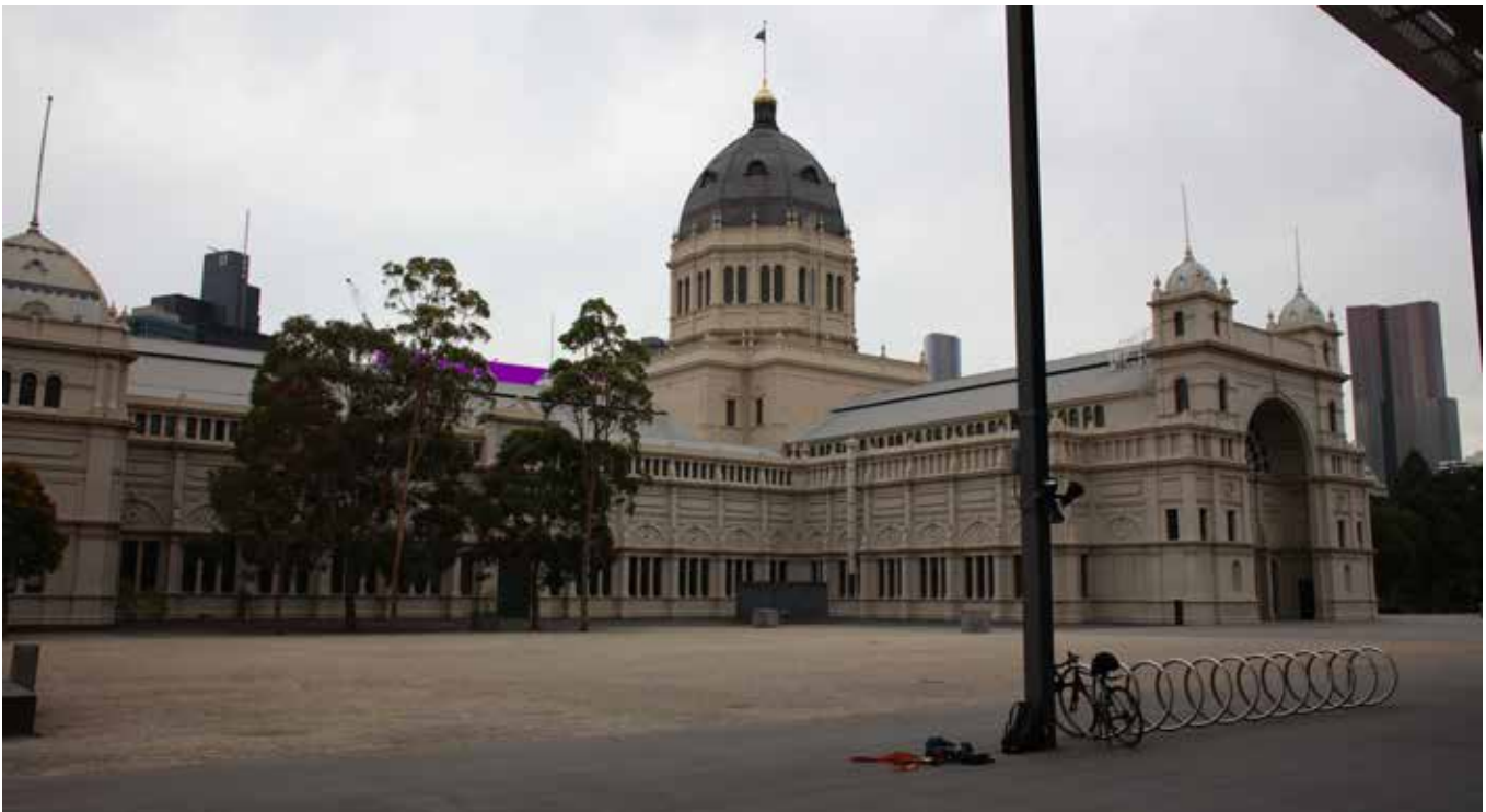
Testing of proposed 10m above 'concealment height' of built form (visible block form)
