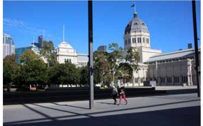
Example of a Primary View of the Dome and the REB
