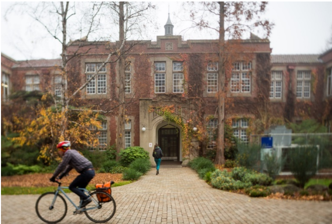
Figure 3 Botany Building (HO329) Source: unimelb.edu.au
