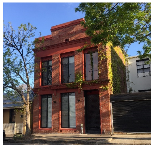
Figure 13 49 Owen Street, Carlton (HO1) Source: Lovell Chen
