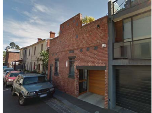
Figure 9 13-23 David Street, Carlton (HO1) Source: Streetview
