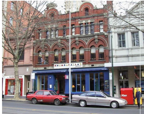
Figure 2 23-29 Bourke Street, Melbourne
