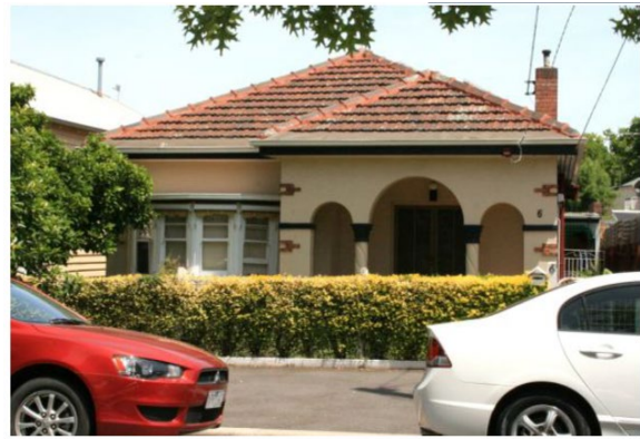
Figure 4 Waddington's houses, 6 Parsons Street, Kensington (HO1167)
