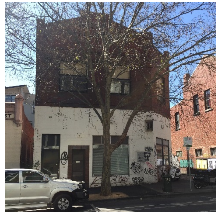
Figure 11 144-146 Queensberry Street, Carlton (HO807) Source: Lovell Chen
