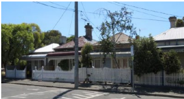
Figure 4 Barnett Street South residential precinct, HO1163 Source: Kensington Heritage Review Statements of Significance, Graeme Butler, March 2018
