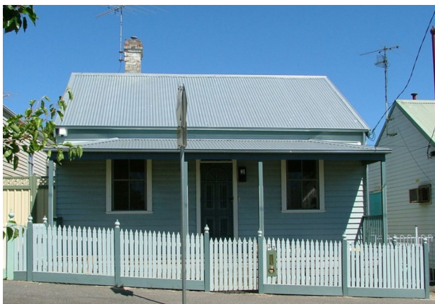
Figure 3 33 Bayswater Road (HO9) Source: City of Melbourne, via Hermes
