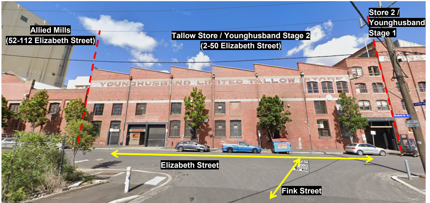
Elizabeth Street frontage (facing west), Source: Google Dec-2020
