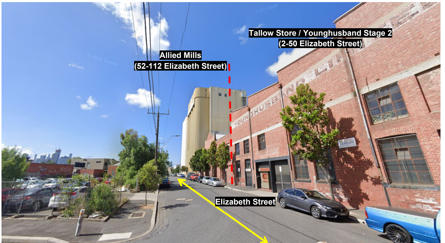
Elizabeth Street frontage (facing south toward Allied Mills), Source: Google Dec-2020
