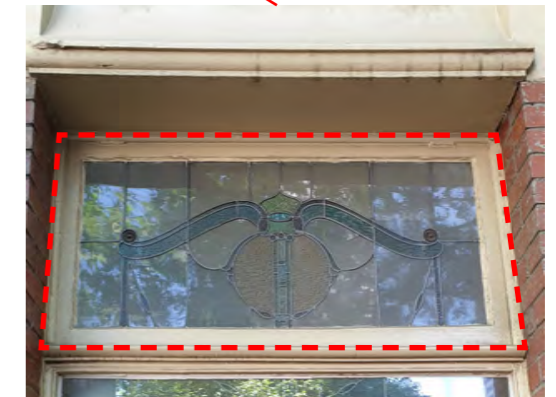
Leadlight windows restored with associated frames repainted and renewed
