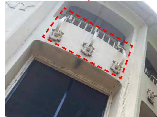
Feature iron balustrade elements restored
