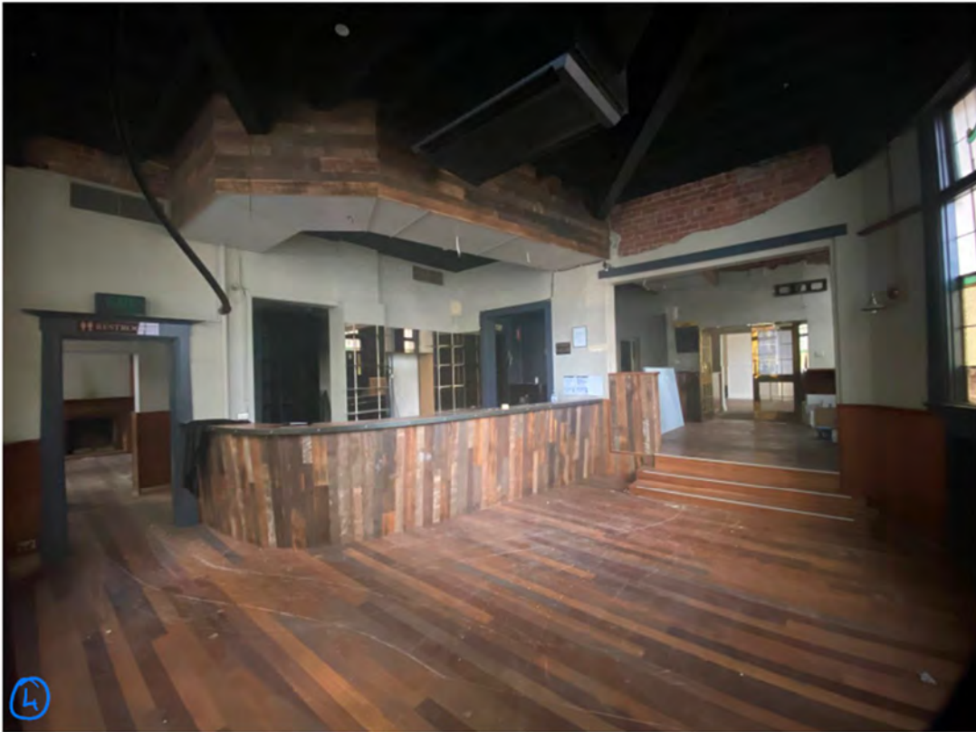
10. Ground floor of Kilkenny Inn. 4. Circular room looking north east. 7.2 metre internal dimension from corner to corner. Source Tract Pty Ltd
