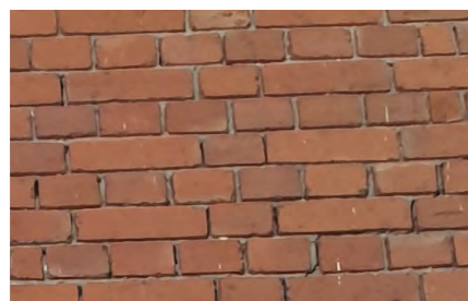
BR 02 Heritage Brickwork
