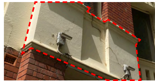
Restoration of rendered facade elements
