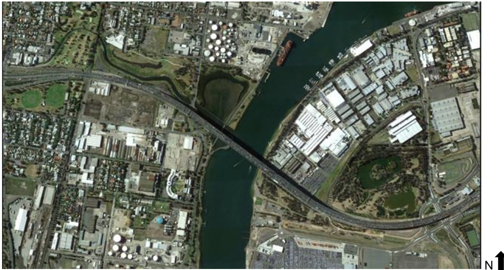
Figure 1: The West Gate Bridge spans the Yarra River
