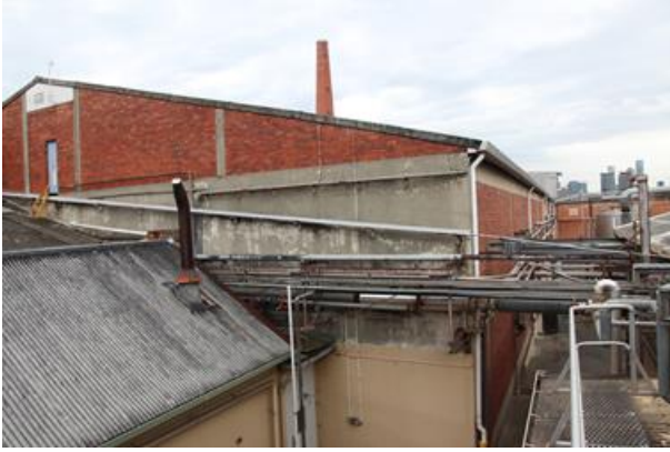
Figures 23: The south and east elevations of the coolroom (P Mills, 4/11/2020)
