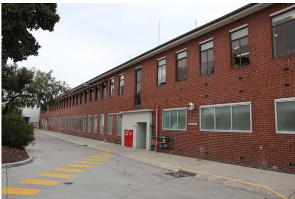
Figure 20: Northwest side of Building 4 on Jindivik Way (P Mills, 2/5/2018)
