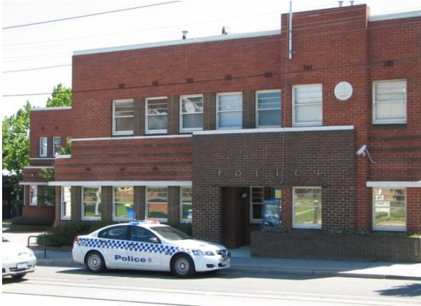
Figure 38: Camberwell Court House and Police Station at 311-317 Camberwell Road, Camberwell. The Court House was designed by Percy Everett and dates to 1938. It is included on the Victorian Heritage Register (H1194). ( http://vhd.heritagecouncil.vic.gov.au/places/1681 )
