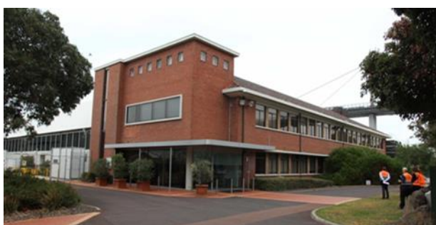
Figure 2: View to Building 6 from Lorimer Street, Gate 2 (P Mills, 2/05/2018)
