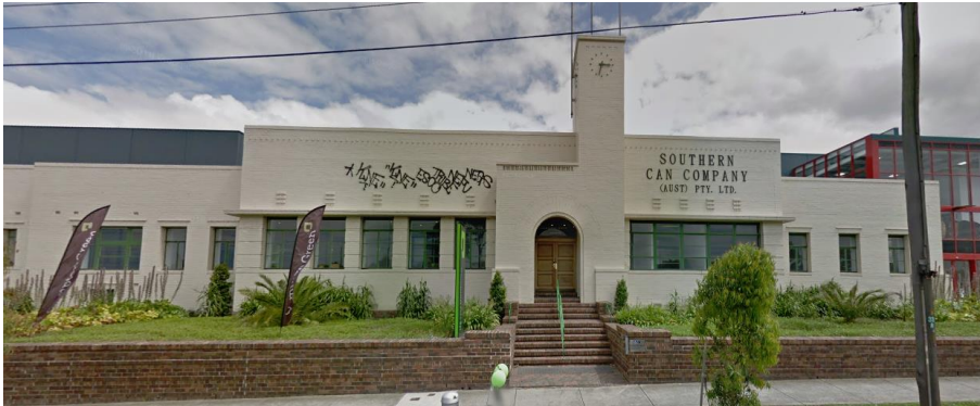
Figure 36: Southern Can Company, 240 Geelong Road Footscray (Google images, December 2017)
