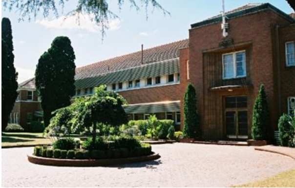
Figure 37: DSTO Administration Building (HLCD, 2004)
