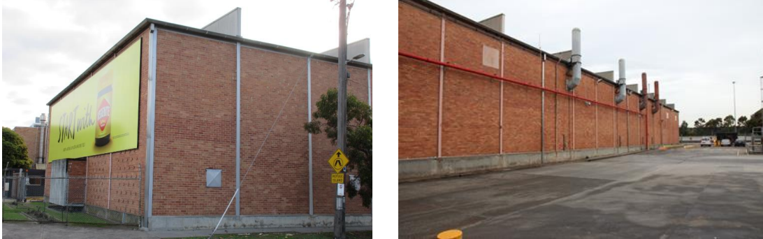
Figures 20 and 21: The 1959-1960 cool store as seen from the Douglas Street boundary and from the northwest. (H Lardner, 10/07/2018; P Mills, 4/11/20)
