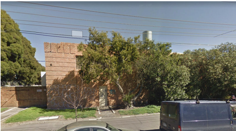
Figure 10: The SEC substation at 193 McKean Street, Fitzroy North (Google image, August 2017)
