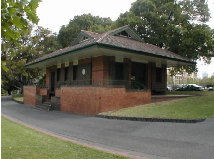
Figure 9: City of Melbourne's c1940 pavilion-style Substation 5 at 2-4 Lansdowne Street, East Melbourne (City of Melbourne i-Heritage database)
