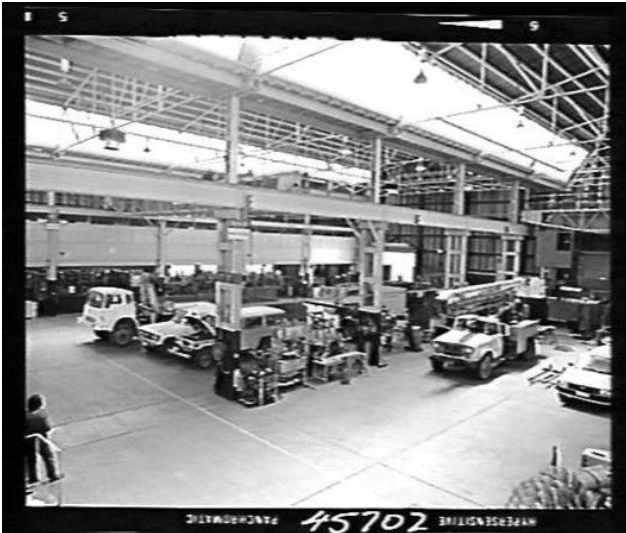
The interior of the large square workshop building with five gables on the west, identifiable by sloping clerestory lighting over box gutters c1968 (MoV MM 11643)
