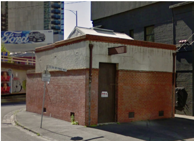
Figure 8: City of Melbourne's 1925 Substation at 7 Moray Street, Southbank (Google imagery, October 18, 2016)
