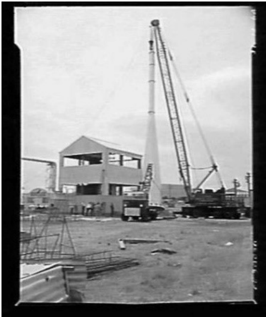
New boiler house construction, 1964 (MoV MM 11316)
