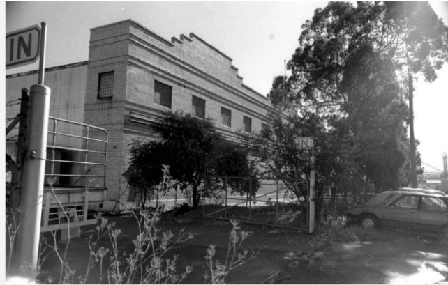
1982 South east corner (Graeme Butler)
