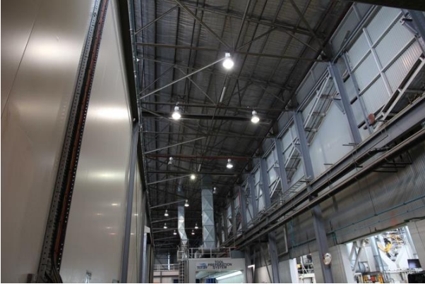
Figure 24: Building 2 interior (P Mills, 2/5/2018)
