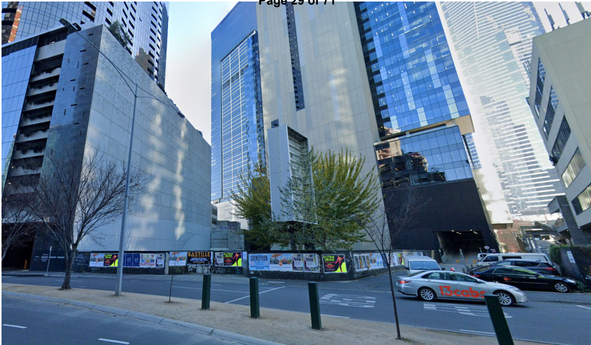
Figure 3 - Site as viewed from Power Street (source: Google streetview)
