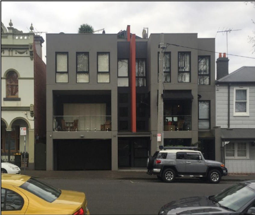
Figure 10 52-54 Macarthur Place North.
