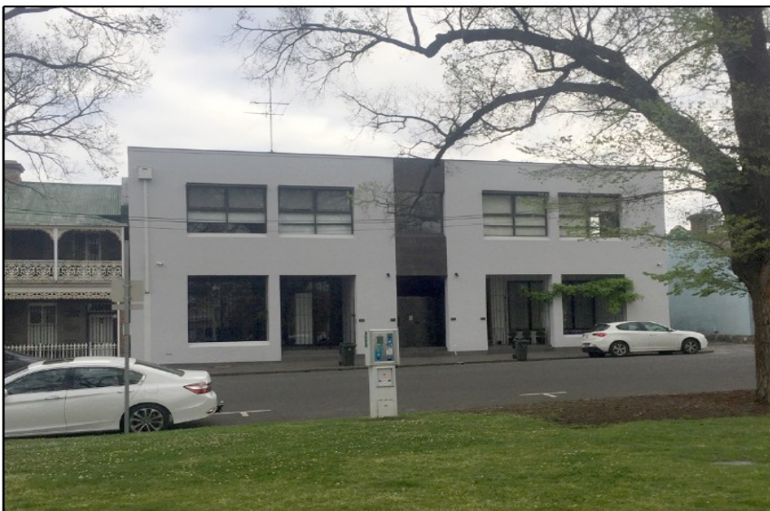
Figure 11 15-21 Macarthur Place North.
