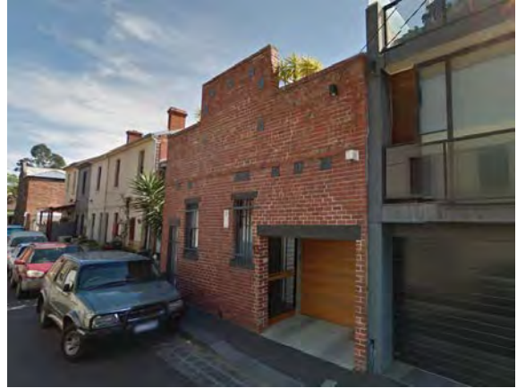
Figure 9 13-23 David Street, Carlton (HO1) Source: Streetview
