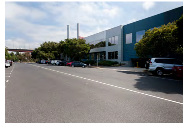
3/ INGLES ST FRONTAGE OF SUBJECT SITE LOOKING NORTH EAST
