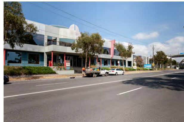
5/ LORIMER ST FRONTAGE OF SUBJECT SITE LOOKING NORTH EAST
